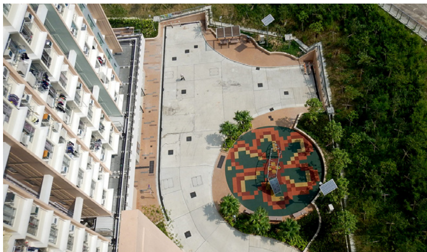
Green treatment for a newly formed slope in Tai Pak Tin Street in Kwai Chung
