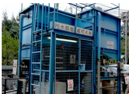
Mandatory installation of water recycling facilities
