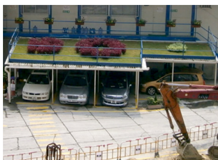
Provision of greening on site
