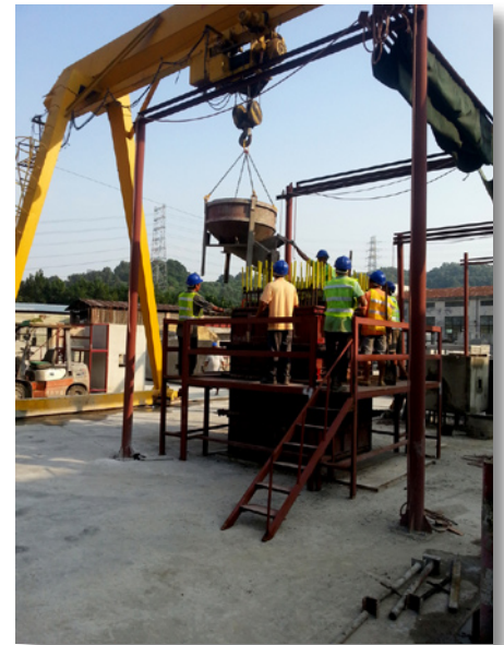
Precast manholes used in Shui Chuen O Phase 1
