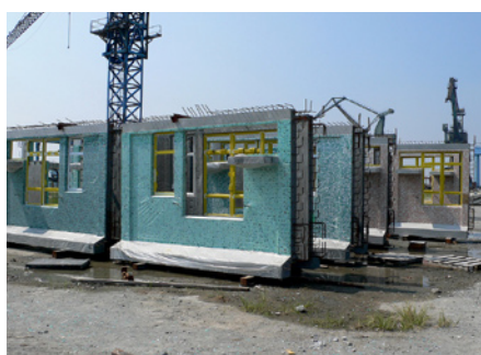
Use of precast concrete component
