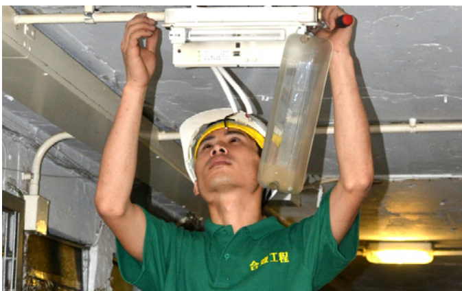
Installation of electronic ballast bulkhead light fitting in Oi Man Estate
