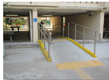
Barrier-free facilities in Oi Man Estate
