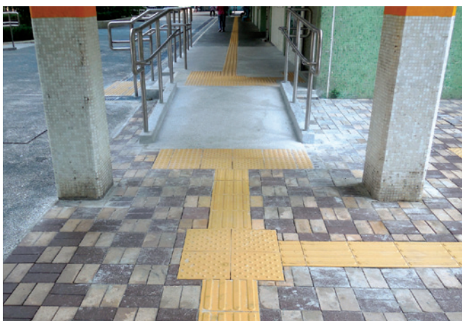
Tactile warning strips and lifts car handrails
