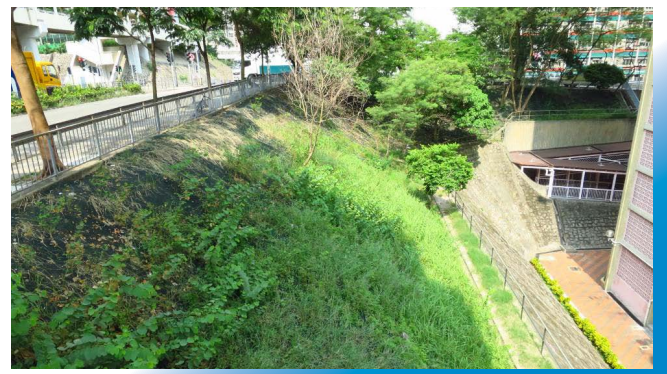
▲ Hydroseeding to Bare Slope Surface in Chuk Yuen South Estate Before (Left) and After Green Treatment Works (Right)
