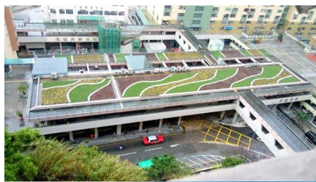
▲ Roof Greening at Kwai Shing West Estate
