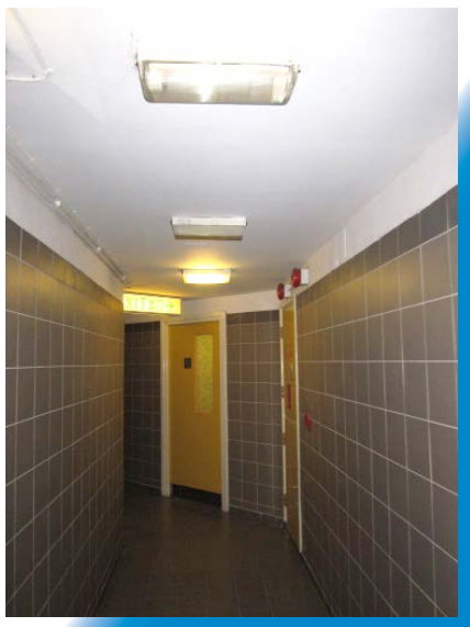
▲ Light Fittings at Tin Heng Estate Replaced with Sensor-controlled LED Light Fittings
