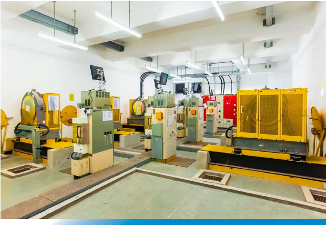
▲ Lift Drives Installation at Kai Ching Estate
