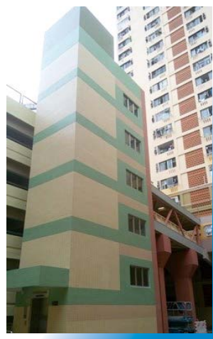
▲ Kwai Shing West Estate Lift Addition
