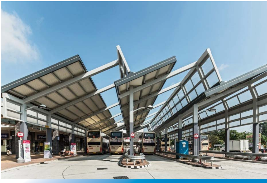
▲ Semi-covered Public Transport Interchange
