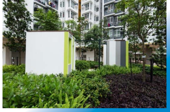
▲ Precast Components in Recycle Garden
