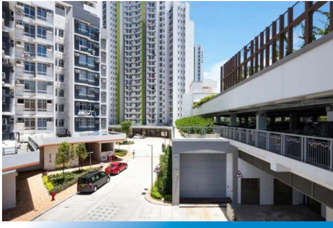
▲ Refuse Collection Chamber (RCC)
