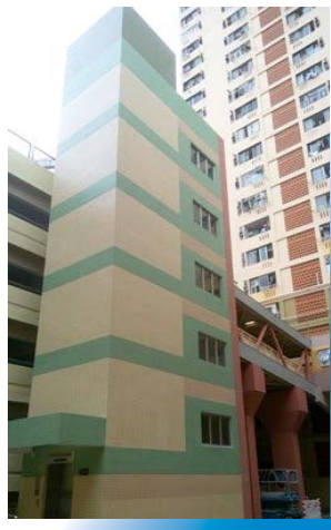
▲ Kwai Shing West Estate Lift Addition
