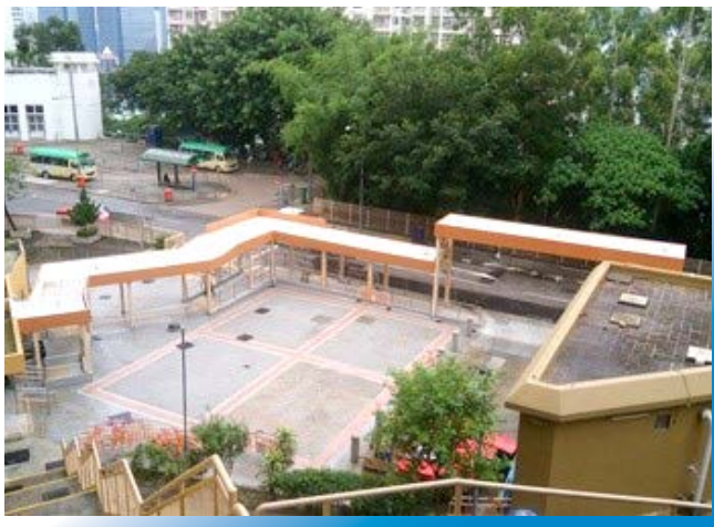
▲ Kwai Shing West Estate Access Ramps
