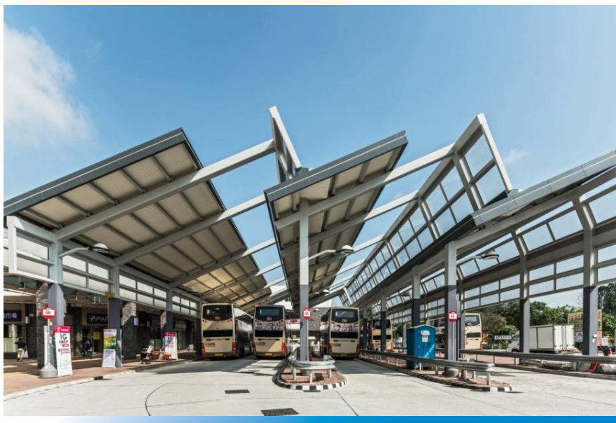
▲ Semi-covered Public Transport Interchange
