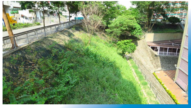
▲ Hydroseeding to Bare Slope Surface in Chuk Yuen South Estate Before (Left) and After Green Treatment Works (Right)
