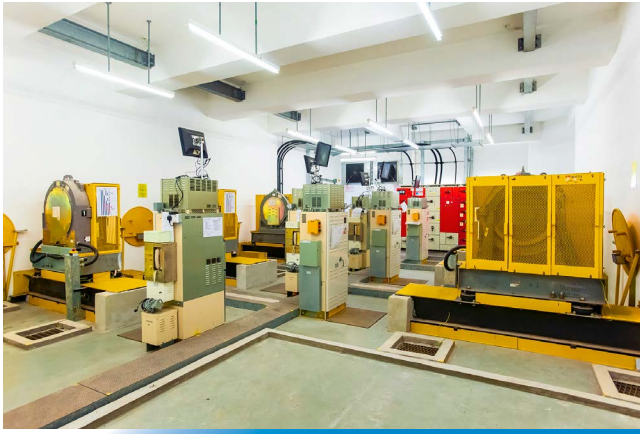
▲ Lift Drives Installation at Kai Ching Estate
