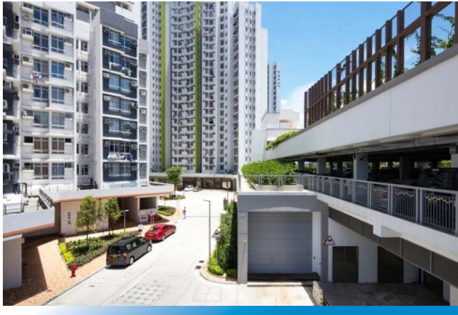
▲ Refuse Collection Chamber (RCC)
