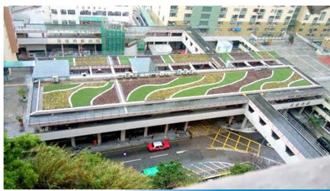
▲ Roof Greening at Kwai Shing West Estate
