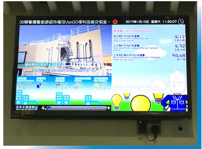
▲ Display of the Smart Meter Monitoring System at Ground Floor Lobby of Tak Long Estate
