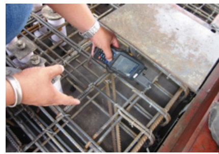
◆ RFID for tracking delivery of building components and construction waste from construction sites
