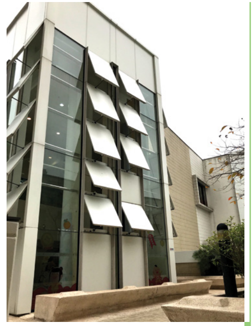
▲ Hybrid ventilation system
