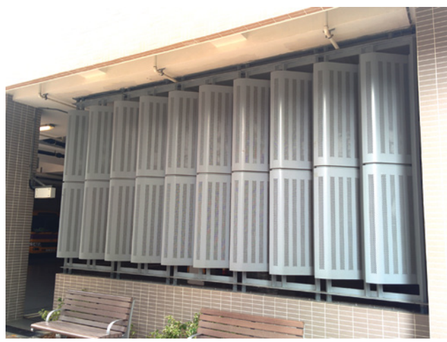
▲ Bio-filtration system at Cheung Sha Wan Estate
