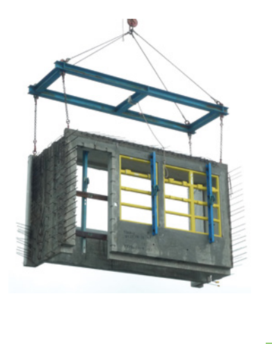
▲ Volumetric precast balconies
