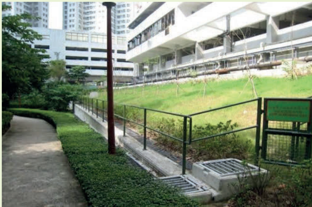
A newly formed slope with hydroseeding and planting in Fung Shing Street
