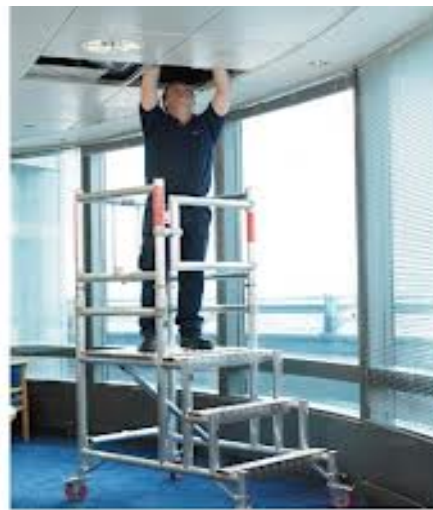
Low-level working platform (toe boards are required when used near building edge or floor opening to avoid risk of falling object)
