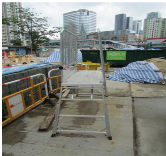
Step platform (full guard-rails and toe-boards are required when used near building edge or floor opening to avoid risk of person and objects falling from height)
