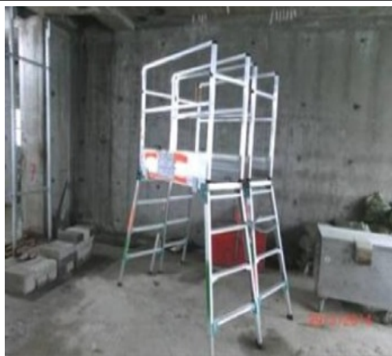
Step platform with platform at more than 900mm but less than 2m from floor level
