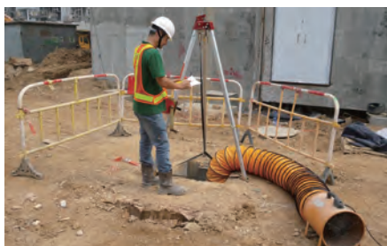
机械通风系统需为密闭空间抽入足够的鲜风 Fresh air supply via mechanical ventilation system to a confined space
