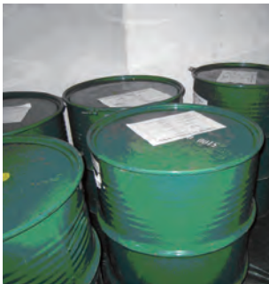
贮存石棉废物于容器内，并加上标签 Containers for asbestos waste and stuck with label
