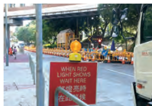
为行车道上的工程采取临时交通安排 Temporary traffic arrangement for work carried out on carriageway
