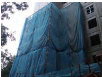
保护幕应覆盖整个受工程影响的外墙 The affected façade of metal scaffolding for works should be covered with protective screen
