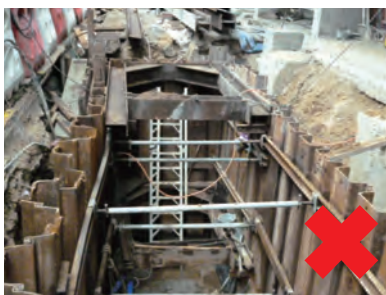
未有于泥坑提供安全进出通道引致工人坠下 泥坑的危害 Hazard of fall of person into excavation due to unsafe access
