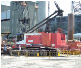
围封工作地区及为移动机械安装防撞棒 Fence off works area and provide warning rod on moving plant
