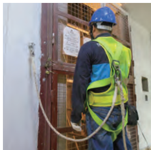
在升降机槽口附近设置锚固点，以供系上防堕装置／全身式安全带。 Provide anchorage near lift shaft opening for anchoring fall arrestor/safety harness
