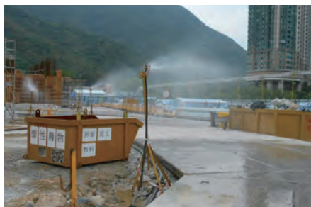
在运料路上洒水，防止尘埃四散。 Dust control by water spraying over the haul road
