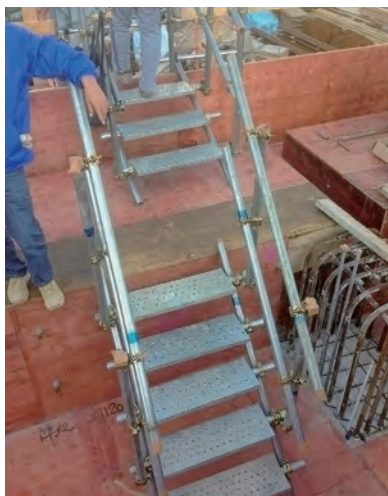
两旁设有扶手的移动式钢梯 A steel ladder (easy movable type) with handrail on both sides
