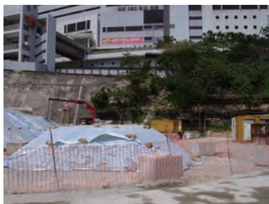
挖掘的物料应妥善遮盖及围封 Excavated material should be properly covered and fenced off
