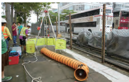
为深井提供机械通风系统 Deep well provided with mechanical ventilation
