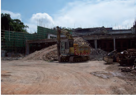
拆卸机械通过斜道驶至下一层 Demolition plant descend a ramp to a lower level
