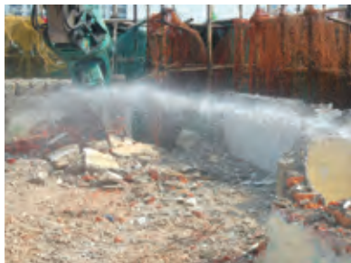
在工地洒水以减少尘埃飘散 Spraying water to reduce the risk of spreading dust from the works site
