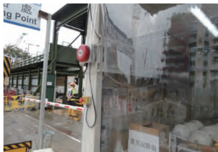
火警钟一般都是安设于物料储存处 Fire alarm bell installed near the material storage area
