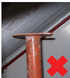
撑杆未有贴紧楼底 Props do not support the bottom of ceiling
