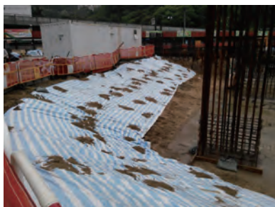
在挖掘工程的斜面盖上有防水功能的塑胶布料 PVC sheeting covers to profile of slope of excavation
