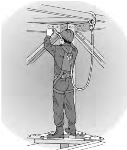
工作前应将随带吊绳系于牢固点 Tie the lanyard to anchorage point securely before works commencement
