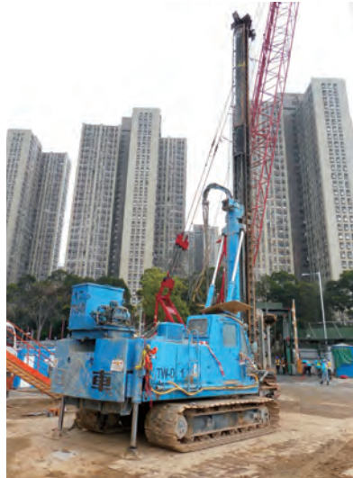
在平地上操作小口径钻桩机 Piling machine operated on level ground
