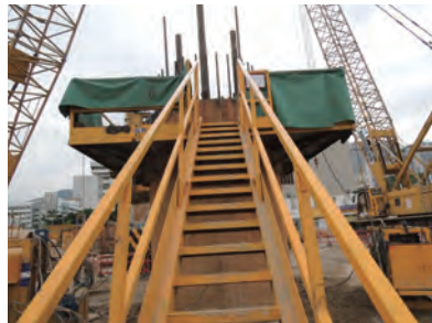
为工作平台提供的护栏和踢脚板 Provide barrier and toe-board to working platform
