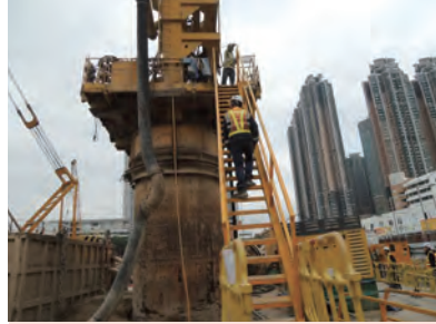
提供有扶手的楼梯往返工作平台 Provide staircase to working platform
