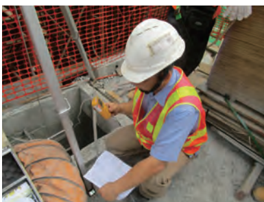
安全主任应在工作许可证上记录空气测试结果 Safety officer records the results of air test of a confined space in the certificate
