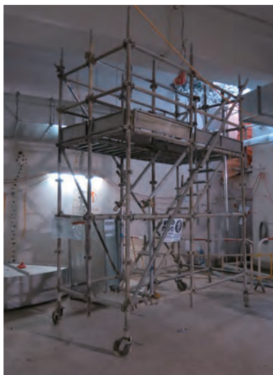
设有轮子锁定装置的流动工作平台 Mobile working platform fitted with castors locking device
