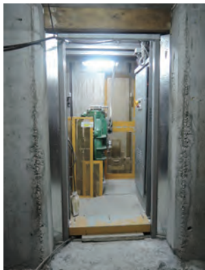
升降机槽内的建筑工地升降机临时机房 Builders' lift cathead inside lift shaft
