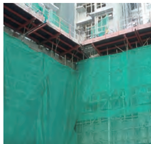
棚架须要合资格人员检查，并须把填妥的表格5贴于棚架显眼的位置 A scaffold should be inspected by competent person with a duly signed Form 5 posted on a conspicuous space
