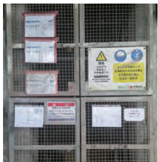
在闸门上张贴足够的安全／警告告示 Sufficient safety/warning notices and permit-to-work posted to barrier
