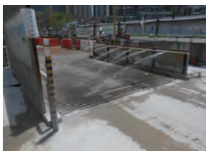
车轮清洗处的喷水器正在运作 Operation of water-jet in a vehicle wheel – washing area
