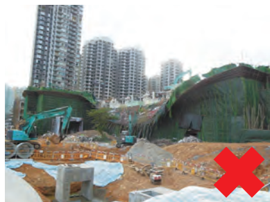
棚架倒塌 Collapse of scaffolding
