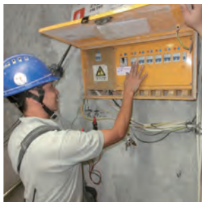
在消除故障后，只有注册电工方可重设配电箱内的开关 Only Registered Electrical Worker allowed to reset the switch of distribution board after fault rectification
