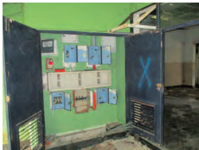
拆卸工程前，要求电力公司必需把主供电截断 Prior to demolition, the main power supply must be dead and disconnected by Power Company
