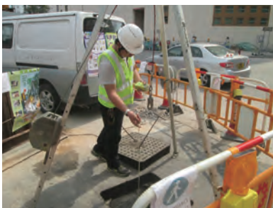
安全主任以气体探测器测试密闭空间内的空气成份 Safety officer uses multi-gas detector to conduct air-testing of the confined space
