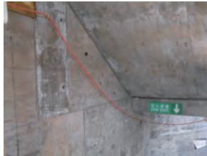
一般电线，如在走廊或楼梯应在高位挂定 Fixing the cable at high level in corridor, staircase
