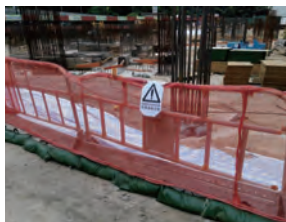
在挖掘工程边缘设置的围栏和土堤并挂上的警告标志 Barrier with warning sign and earth bund along the edge of the excavation
