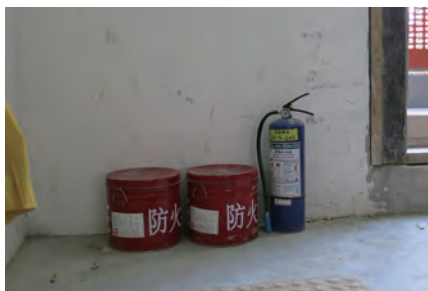
在标准楼层提供灭火筒和沙桶 Provision of fire extinguisher and buckets of sand on typical floor
