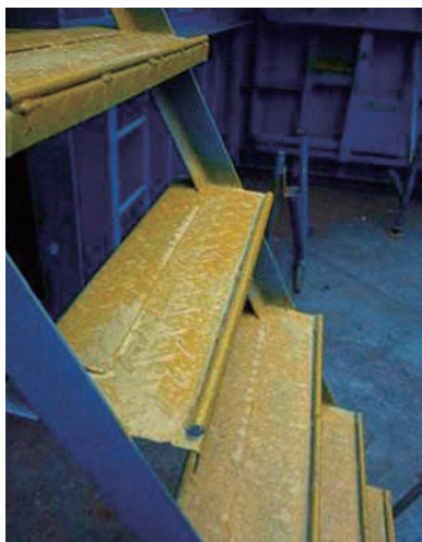
梯子级面加上金属杆，增强防滑效果 Access staircase with additional steel rod as anti-slip device
