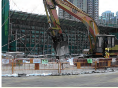
为免大量地面水流进土坑，挖掘工程的边缘应放有土堤或沙包等 Provide earth bund or sand bags along edge of excavation to curb surface water run off
