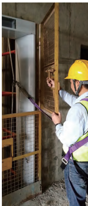
当需要进入升降机槽或井底工作时，工人必需将随带吊绳紧固于独立救生绳 Worker should attach the lanyard to the independent lifeline before making access to lift pit/shaft
