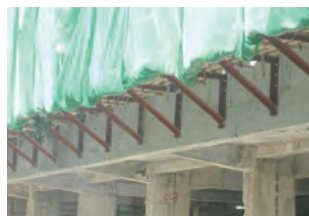
钢料托架必须有足够强度和按照注册结构工程师核准的施工说明书安装 Steel bracket with adequate strength installed according to the method statement approved by registered structural engineer
