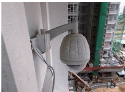
闭路电视摄录机设置在吊运区上方，协助塔式起重机操作员进行吊运操作 CCTV camera with recording function positioned above lifting zone to assist tower crane operator to carry out the lifting
