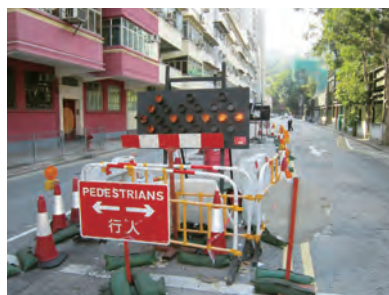
为行道上的工程采取临时交通安排 Temporary traffic arrangement for work carried out on carriageway
