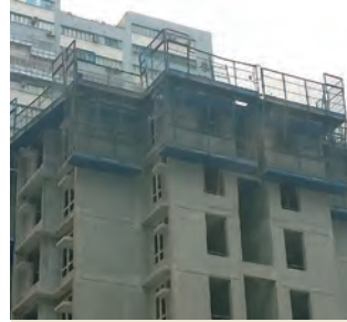
在工作平台边缘安装护栏 Guard-rails installed to perimeter of large steel formwork
