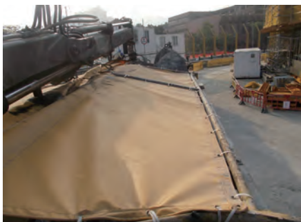
以胶布覆盖卸泥货车，以防易生尘埃的物料飞散 Dump truck with PVC cover to prevent spread of dusty materials
