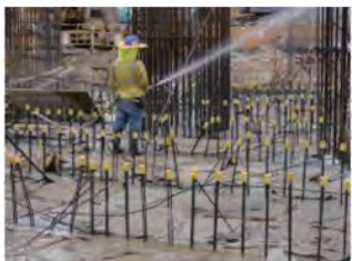
以铝槽和胶盖覆盖金属枝 Aluminium trough and plastic caps to cover the metal bars
