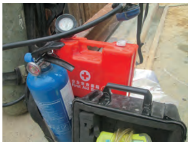
在密闭空间入口附近设置的急救箱和灭火器 Provision of first aid box & fire-fighting apparatus near the entrance of a confined space
