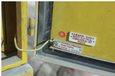
金属可导电部份如门，须由等位电线接地，并挂上标签牌（安全接地终端 - 切勿移去） Bonding conductor should be connected to the metal door with warning label "safety electrical connection - do not remove"
