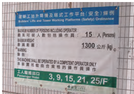
建筑工地升降机旁需有展示载人数目的告示 Capacity displayed adjacent to entrance of a builder's lift
