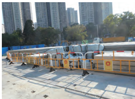
在指定并围起的安全范围内整齐堆放物料 Materials stacked neatly in a safe fenced and designated area
