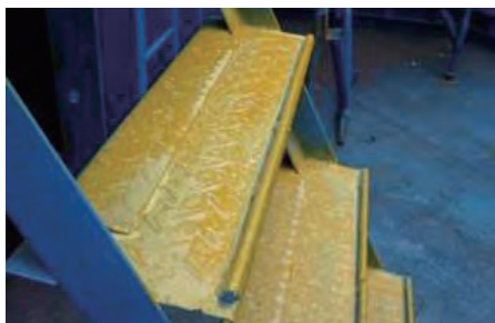
于梯级加装钢棒，有助防滑 Additional steel rod on the staircase as anti-slip device
