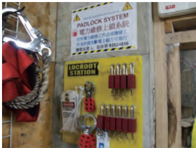
一套齐全的工地电力上锁系统 A well equipped padlock system of a construction site
