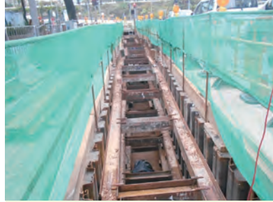
为深度超过1.2米的挖掘沟槽提供支撑设施 Shoring support to excavation with depth greater than 1.2m
