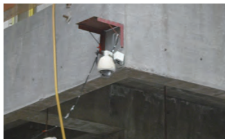
吊运区域低层装设附有录影功能的闭路电视系统，可供操作员监察吊运作业过程 CCTV camera installed at low level of lifting zone for operator to monitor the lifting operation process
