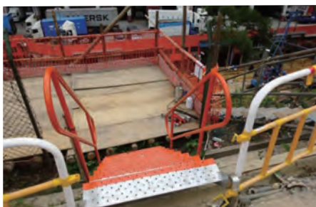
前往斜坡工作地点的安全通道 Safe means of access for slope work
