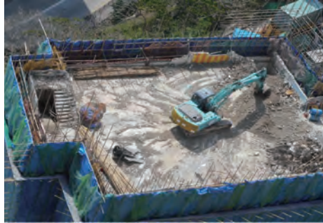
拆卸下的废料，应及时移除，以免超出负荷 Debris on the demolishing floor must be removed/cleared regularly to avoid overload to the structure
