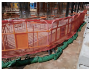
在挖掘工程边缘设置的围栏和土堤并挂上的警告标志 Barrier with warning sign and earth bund along the edge of the excavation
