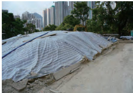
用防水布为斜坡提供适当的保护 Protect slope with tarpaulin cover
