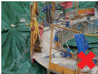
没有合适围栏造成人体从高处坠下风险 Risk of fall of person from height due to missing proper guard rail
