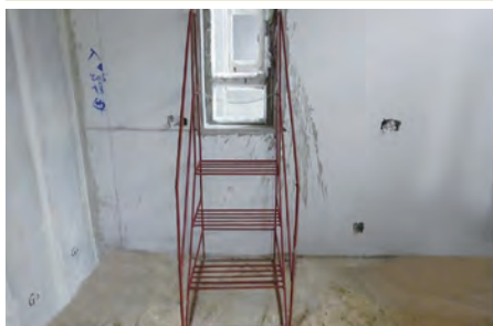
前往吊船的安全通道 Safe means of access to gondola
