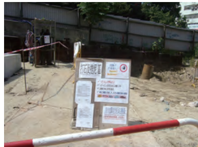
挖泥区放置围栏及警告告示 Barrier with warning notice to excavation
