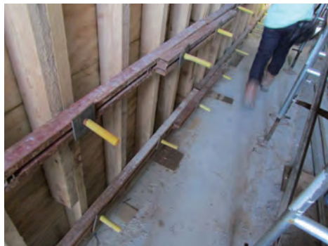
对突出的螺栓作好防护 Protection for projecting bolts
