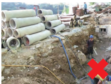
遭坠下沟槽的物件击中的危害 Hazard of being struck by materials falling into trench
