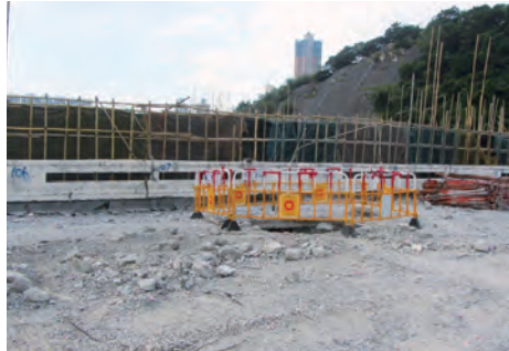
在楼面地台开口位置，应竖设围栏防止物料下堕 Hole/opening on the demolishing floor should be protected with fencing from falling object
