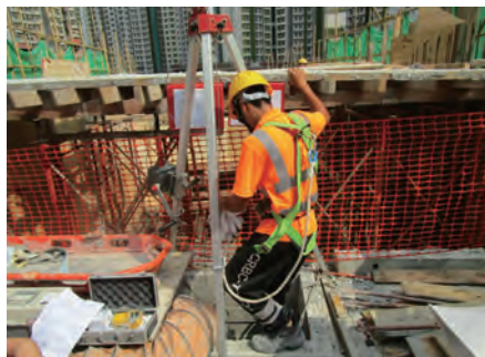
工人进入密闭空间前，应把全身式安全带和救生绳系稳。 Full-body harness and lifeline securely fixed before entering a confined space
