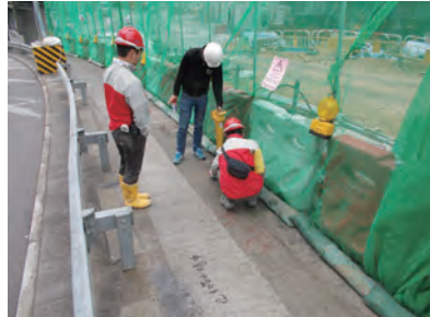
以探测器和量度工具等去确定地下公用设施的位置 On site identification for existing underground utilities with detector and measuring instrument
