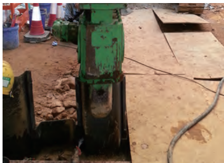
利用隔音罩减少噪音 Reduce noise by means of noise barrier
