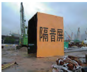
为建筑地盘设置隔音屏 Noise screen provided for construction site
