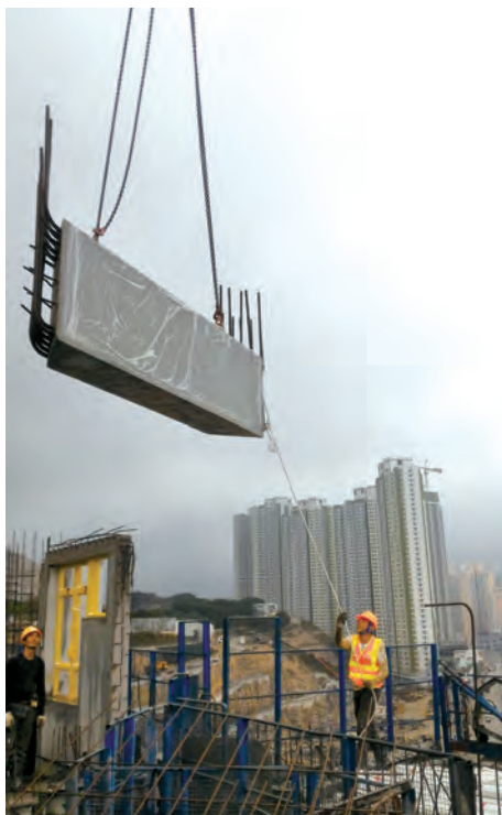
索具工吊运固定好的预制横梁 Lifting and fixing precast concrete beams by rigger
