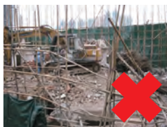
棚架损毁 Damage of scaffolding
