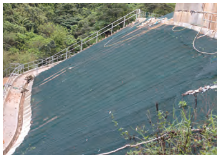
在斜坡底设 U 形排水道，并用防水布保护斜坡面 Provide U-channel at toe of cutting and cover slope surface with tarpaulin
