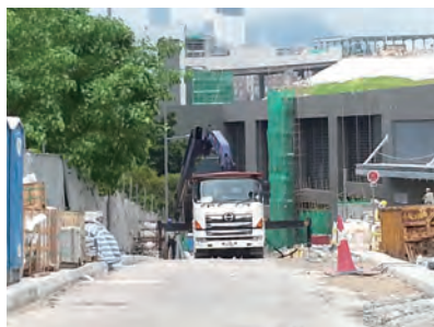
当随车式起重机运作前，其支重脚撑应完全伸展及其踏板正确放在起重垫板上 Lorry-mounted mobile crane under operation should fully extend the outrigger legs
