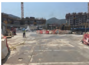
洒水以免尘土飞扬 Dust control with water spraying
