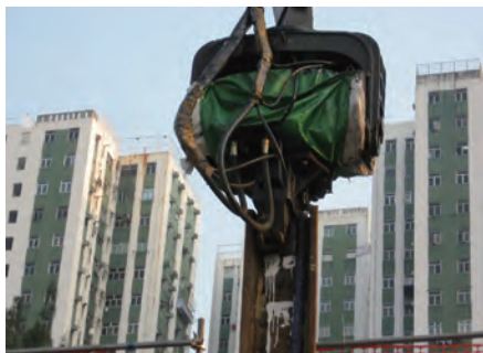
利用震锤减少打闸板桩产生的噪音 Noise attenuation using vibration hammer during sheet piling installation
