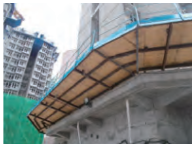
设置临时保护篷，为工人提供安全的进出通道 Temporary protective canopy for workers with a safe access/egress
