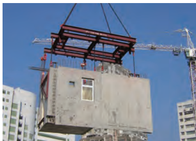
安全吊运大型预制组件 Lifting volumetric precast concrete unit with lifting frame
