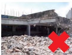
缺乏支撑的横梁 No support to beam
