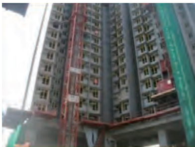
在大厦的第七层楼板工作尚未展开前，应完成设置大厦的临时保护篷 The erection of protective canopy should be completed before the 7th floor slab is cast
