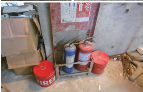
在重要位置提供灭火筒和沙桶 Fire extinguisher and buckets of sand at strategic locations
