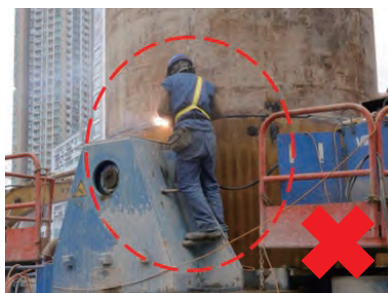
工人没有适当保护引致人体从高处坠下的 风险 Hazard of fall of person from height due to lack of fall protection measure
