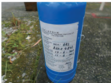
在密闭空间附近设置灭火器 Provision of fire-fighting apparatus near a confined space
