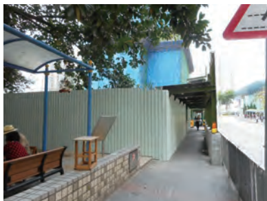
沿地盘界线的围板和有盖行人路设置坠台，以保护行人。 Hoarding and covered walkway with catch platform along the site boundary to protect pedestrian
