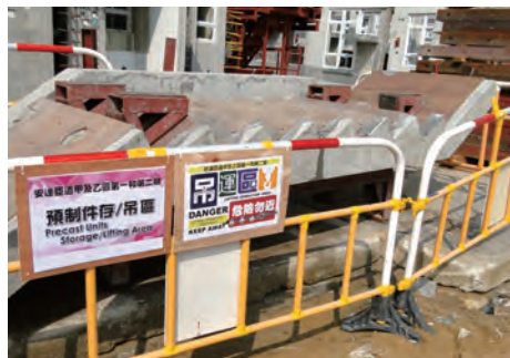
妥善放置贮存及围封预制楼梯 Precast concrete staircases properly stored/fenced off
