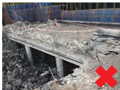
没有妥善围封／承托拆卸工程范围 No proper fencing/support to demolition areas
