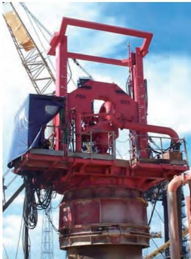
大口径钻孔桩一般涉及的机械 Plant and equipment used in large diameter bored pile construction
