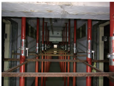
提供支撑和支柱承托须拆卸的建筑物 Shoring and propping for buildings to be demolished
