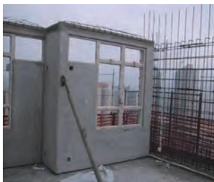
为外墙安装支撑托架 Install supporting bracket for facade
