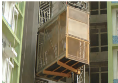
升降机吊笼要有足够围封 Substantial enclosure to builder's lift car cage
