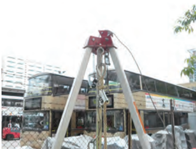
在密闭空间工作时，工人的救生绳需系稳在密闭空间外 The lifeline of the worker working inside the confined space is tied securely outside a confined space
