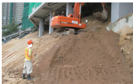
为挖土机操作员安排讯号员 Signaler works with the excavator operator
