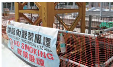
楼洞的边缘设置围栏 Guard-rail around floor opening
