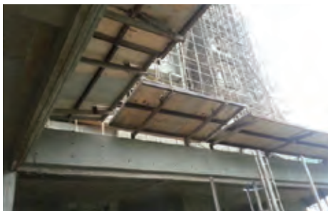
在大厦的第七层楼板工作尚未展开前，应完成设置大厦的临时保护篷 The erection of protective canopy should be completed before the 7th floor slab is cast
