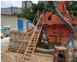
另一设置扶手的楼梯，供通往工作平台 Provide handrails to staircase leading to working platform
