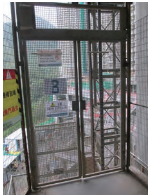
建筑工地升降机装有全高度的闸门 Full height gate for a builder's lift
