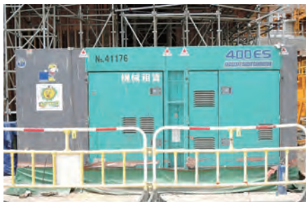
设置栏杆以防止有人容易地闯进低电压设备的范围 Railing to restrict unauthorized access to working zone of low voltage equipment.
