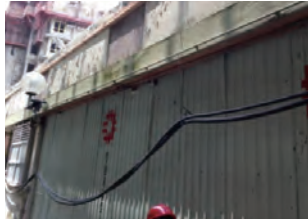
室外电线，应在高位挂定 Fixing the outdoor cable at high level
