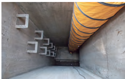
为深井提供机械通风系统 Deep well provided with mechanical ventilation
