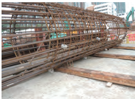
钢筋笼底部放置楔子 Proper wedges to be provided at bottom of reinforcement casing
