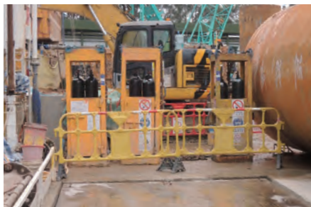
乙炔气瓶和氧气瓶须贮存在有良好通风的地方 Store the acetylene and oxygen cylinders in a well ventilated area
