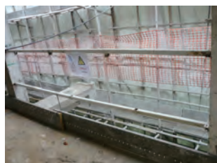
设有防护围栏的外间开口 External opening provided with protective barrier
