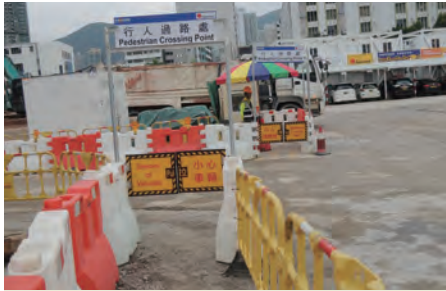
在硬地以可摺合的围栏分隔行人和车辆 Folding type barrier to separate pedestrians and vehicles on a hard paved road
