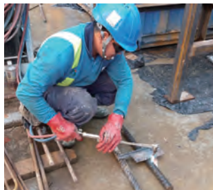
在火焰切割工作时，焊接工人应佩戴合适的个人防护装备 Welder should put on adequate personal protective equipment during the course of flame cutting works
