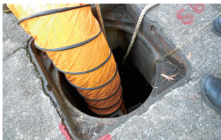
在密闭空间入口提供机械通风／救生绳 Mechanical ventilation/lifeline provided at the entrance fo confined space
