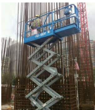
工人操作及使用动力操作升降工作平台时，须穿上全身式安全带并系稳于工作平台上指定的牢固点上 Worker needs to wear safety harness attached to a designated anchor point of the mobile elevating work platform when the platform in operation.
