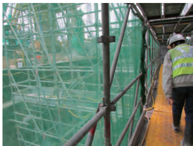
工作平台应设有踢脚板、顶部护栏和中间护栏 Working platform with toe board, top and intermediate guard-rails
