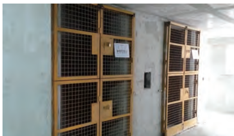
为升降机槽入口提供全高度的四页钢闸 Provision of 4-leaf full height steel barrier to lift shaft opening
