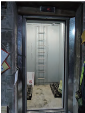
升降机槽内的建筑工地升降机机厢 Builders' lift car inside lift shaft
