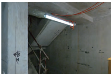
电力装置（例如照明装置和电线）尽安装于离地面至少两米高处 Electrical installations such as lighting & wiring to be mounted/fixed at high level ( \geq 2\text{m} )
