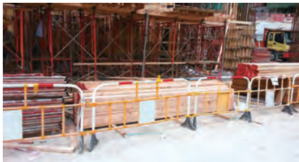
物料存放区应妥善围封及把物料存放有序 Area for materials is securely fenced off and stored in an orderly manner
