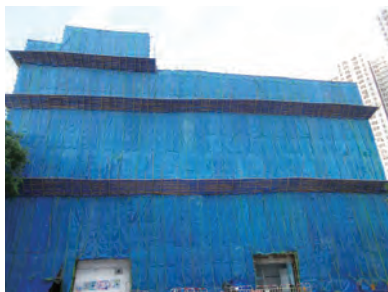
利用保护幕和以塑胶或柏油帆布制造的隔尘网，围封整幢须拆卸的建筑物，再搭建中层斜棚。 Building to be demolished to be fully enclosed by protective screen and dust screens of plastic or tarpaulin sheet, with intermediate catch-fans
