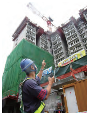
讯号员利用无线电沟通，以确保工序安全进行 Signaler using radio means for a safe lifting operation
