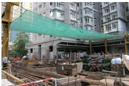
为扎铁工地提供保护网 Safety net provided above steel bending workplace
