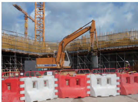
设有吸音装备的气压碎石机 Pneumatic breaker equipped with noise absorber
