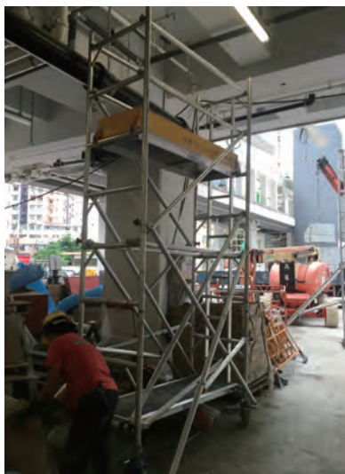
装有踢脚板，顶部及中间护栏的工作平台 Mobile working platform with toe board, top & intermediate railing
