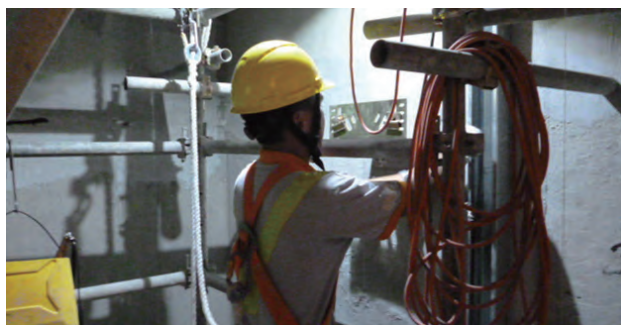
全身式安全带要挂在升降机槽内的救生绳 Safety harness attached to lifeline inside lift shaft
