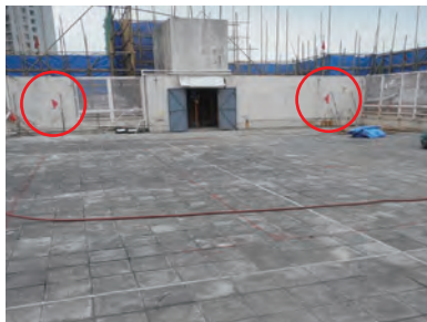
移动拆卸机械在红旗标示的范围内，可安全进行作业 Red flags set up to demarcate the restricted area for safe operation of moving machinery
