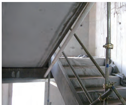
楼梯设置 Guard-rails along staircase
