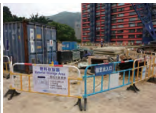
在围封范围划定安全的出入途径 Designated safe means of access to enclosed area
