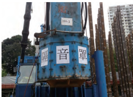
利用隔音罩减少噪音 Reduce noise by means of noise barrier
