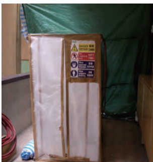
以帆布完全围封石棉工程范围 Full enclosure of asbestos work zone by canvas sheet
