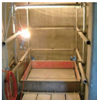
安全通道进入升降机槽的工作平台 Proper access to working platform in lift shaft
