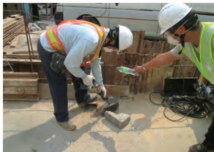
使用手提气动碎石机时佩戴全套个人防护装备，例如护耳罩、安全鞋、头盔、眼罩、手套、口罩等。 Full personal protective equipment such as ear muff, safety shoes, safety helmet, goggles, gloves, mask, etc. for using handheld pneumatic breaker
