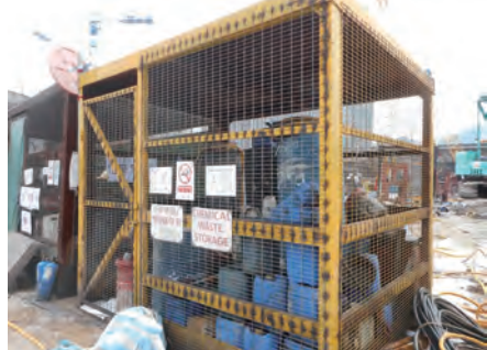
应为危险物料贴上标签，及妥善存放于订明的地方 Dangerous materials should be properly labeled and stored in designated area
