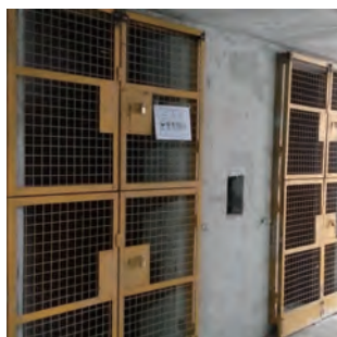
安装全高度四扇金属闸门，防止工人擅闯升降机槽。 Full height 4-leaf metallic gate to restrict unauthorized access to lift shaft
