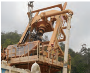
穿上防堕装置的工人在设有护栏的工作平台上操作机械 Barrier and fall arrest system for workers working at height
