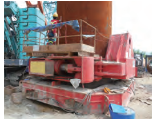
设有护栏的工作平台 Working platform with railings for workers working at height
