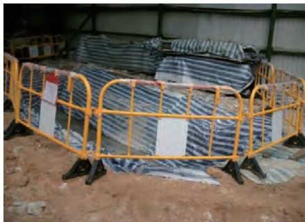
深坑的斜面盖上塑胶布料，以免受天气影响 Profile of slope of a deep excavation is protected from weather with PVC sheet
