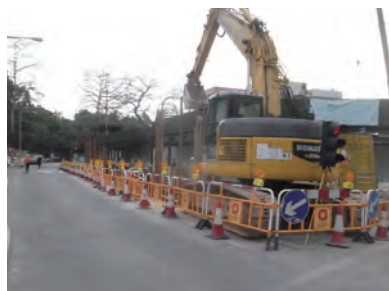
以重型建筑机械及围栏确定出安全工作地带 Work safety zone demarcated by construction machine and barrier
