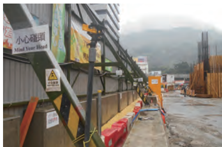
防止尘埃四散的自动洒水系统 Automatic water spraying system to control dust
