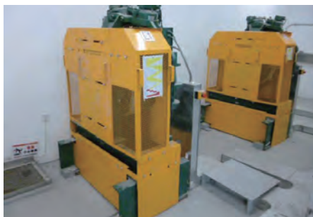
升降机或电动绞车必需安装护罩 Guard provided for lift machines and electric winch
