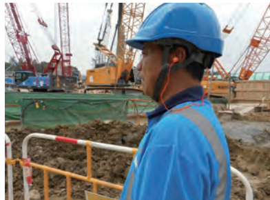
在噪音环境下工作应佩戴合适的护耳罩或耳塞 Suitable ear muff or ear plugs adopted in a noisy working environment
