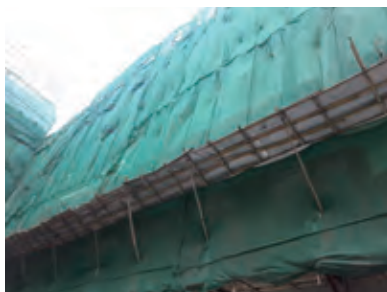
斜棚应从建筑物外棚向外伸延1,500毫米 Catch-fan projected at least 1,500mm horizontally from the scaffolding
