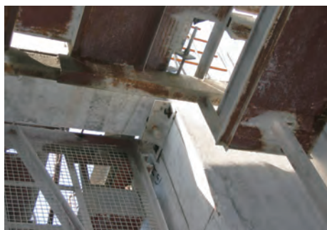
提供钢料托架,方便安装横梁 Temporary bracket for fixing precast beam
