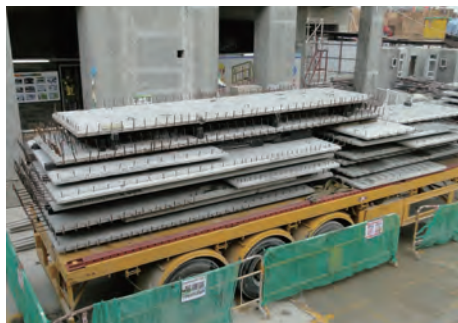
妥善围封未下架的预制楼面板 Loaded precast concrete slabs are properly fenced off
