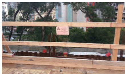
楼边位置安装有适当的木制围栏 Proper timber guard rail along edges of working floor
