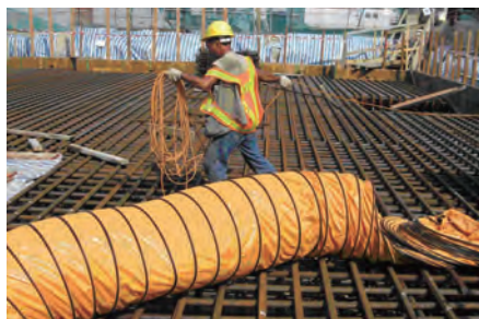
天气炎热时，为大型桩帽内的工作间提供机械通风 Mechanical ventilation is provided to a working area inside a large pile cap during hot weather
