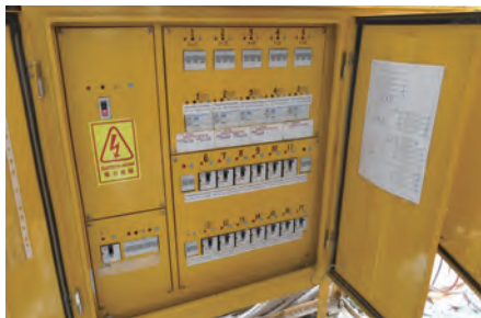
典型配电箱（屏）都装置电路保护器如MCB/RCD Typical distribution board with circuit protection device as MCB, RCD
