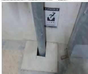
封盖好的楼洞需要贴上警告标示 Cover to the floor opening securely fixed with warning notice
