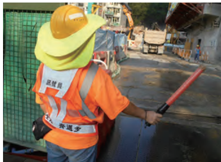
安排讯号员于狭窄通路指挥交通 Signaller to control/direct the traffic in a narrow road
