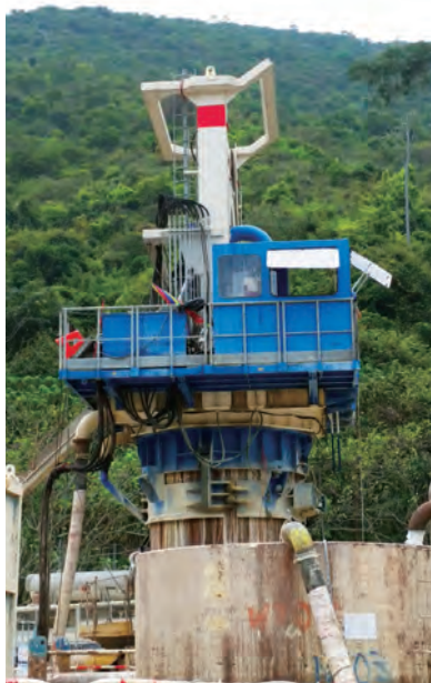
为大口径钻桩工程进行高空工作的操作员／ 工人应有安全措施提防从高处坠下 Large diameter bored pile with operators / workers working at height-to be cautious of hazard of falling from height
