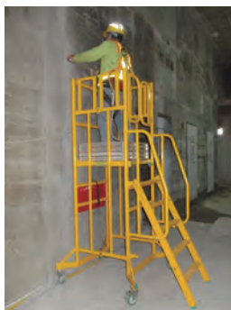
安全梯台于两旁设置扶手 Step platform with handrails on both sides
