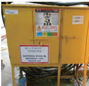
在消除故障后，只有注册电工方可重设配电箱内的开关 Only Registered Electrical Worker allowed to reset the switch of distribution board after fault rectification
