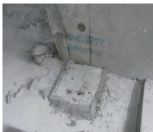
临时以水泥封盖好的楼洞 Properly cover floor opening
