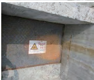
封盖好的楼洞需要贴上警告标示 Cover to the floor opening securely fixed with warning notice
