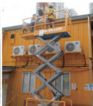
动力操作升降工作平台四边装设护栏，避免工人发生意外而受伤 Mobile elevating work platform fitted with guard on four sides for protection of workers from accident
