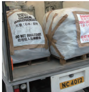
贮存石棉废物于容器内，并加上标签 Containers for asbestos waste and stuck with label
