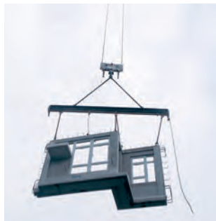
建筑地盘常用的吊梁 Commonly used spreader beams on construction site
