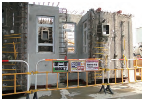
妥善放置贮存及围封预制组件 Precast concrete unit properly stored
