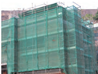
安全网完全覆盖整个棚架 Entire metal scaffolding is covered with safety net
