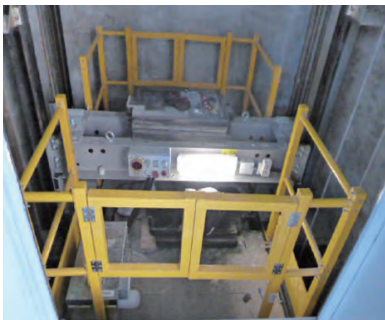
升降机顶上的工作台设有围栏及踢脚板 Working platform with railing and toe board on lift car top
