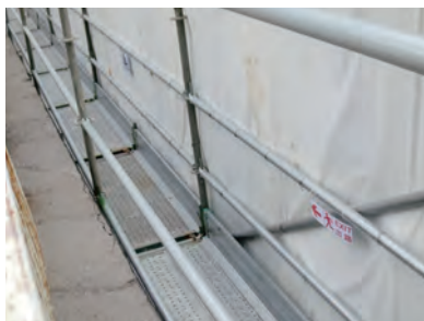
设有金属桥板、金属踢脚板、顶部护栏和中间护栏的工作平台。 Working platform with metal plate, metallic toe board, and top and intermediate guard-rails
