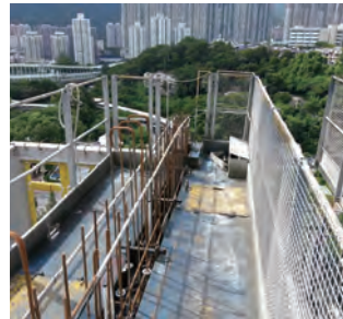
工作平台护栏以金属丝网围封 Parapet wall of a working platform is fenced with wire mesh
