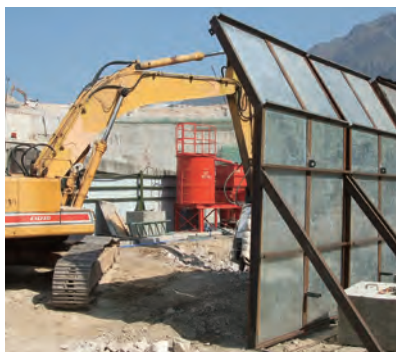
进行岩石挖掘工程时设置隔音屏。 A noise screen is provided during rock excavation.
