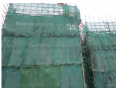
保护幕应覆盖整个外墙棚架 Entire bamboo scaffolds should be covered with protective screen
