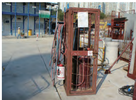
乙炔气和氧气瓶须时存于通风的地方 Store the acetylene and oxygen cylinders in well ventilated area
