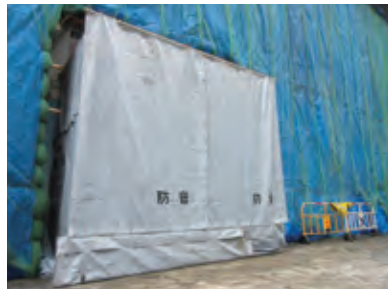
为拆卸工程范围提供隔音屏障 Noise screen provided for demolition works
