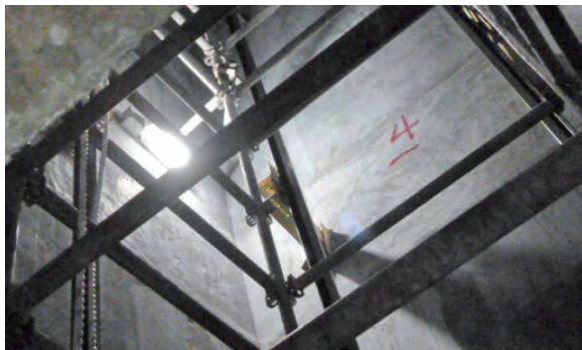
升降机槽中有充足的照明 Sufficient lighting for works in the lift shaft
