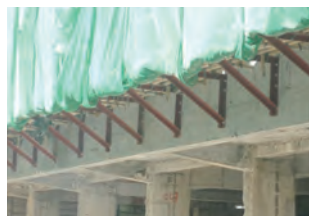
鋼料托架必須有足夠強度和按照註冊結構工程師核准的施工說明書安裝 Steel bracket with adequate strength installed according to the method statement approved by registered structural engineer
