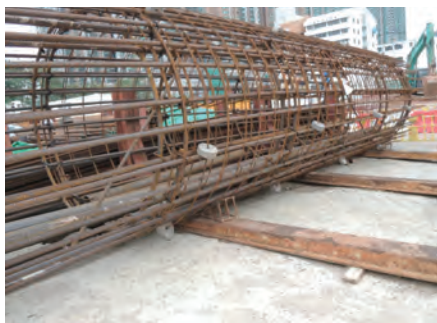
鋼筋籠底部放置楔子 Proper wedges to be provided at bottom of reinforcement casing
