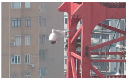
吊運區域低層裝設附有錄影功能的閉路電視系統，可供操作員監察吊運作業過程 CCTV camera installed at low level of lifting zone for operator to monitor the lifting operation process
