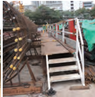
為安全紮結鋼筋籠提供弧型結構支 架底座 Arc-shaped fabrication frame provided for a safe erection/tying of reinforcement casing
