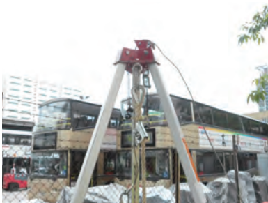
在密閉空間工作時，工人的救生繩需繫穩在密閉空間外 The lifeline of the worker working inside the confined space is tied securely outside a confined space
