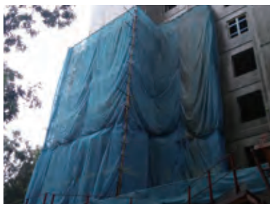
保護幕應覆蓋整個受工程影響的外牆 The affected façade of metal scaffolding for works should be covered with protective screen
