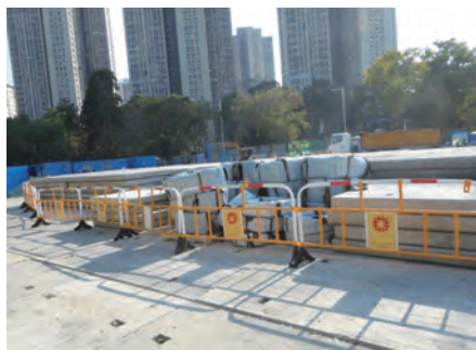
在指定並圍起的安全範圍內整齊堆放物料 Materials stacked neatly in a safe fenced and designated area
