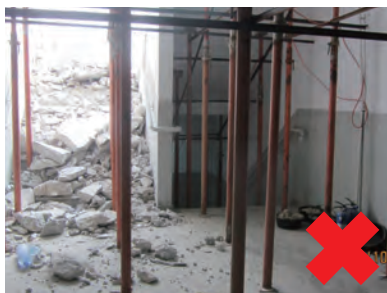
往返工作樓層的通道給廢料阻塞 Obstructed access/egress
