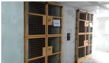
為升降機槽入口提供全高度的四頁鋼閘 Provision of 4-leaf full height steel barrier to lift shaft opening
