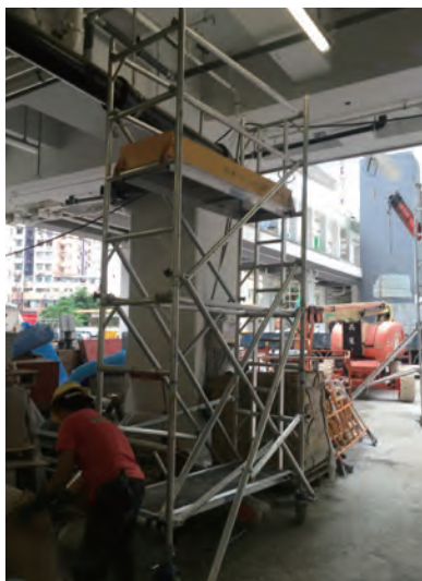
裝有踢腳板，頂部及中間護欄的工作平台 Mobile working platform with toe board, top & intermediate railing
