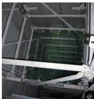
適用於升降機井道的金屬棚架 Metal scaffold for working inside lift shaft
