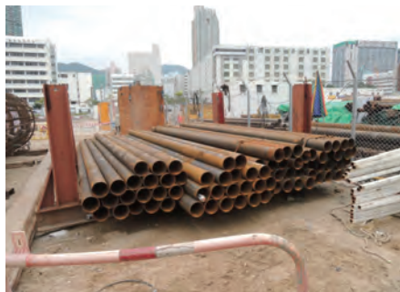
在指定並圍起的範圍內整齊堆放物料 Materials stacked neatly in a designated and fenced area
