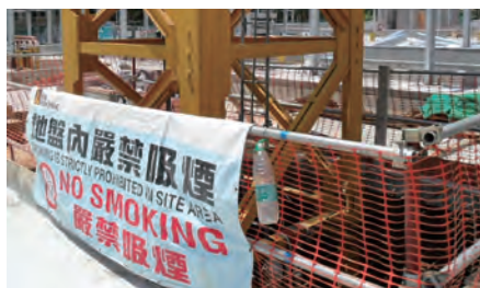
樓洞的邊緣設置圍欄 Guard-rail around floor opening
