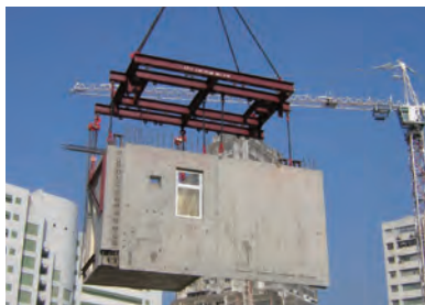
安全吊運大型預製組件 Lifting volumetric precast concrete unit with lifting frame
