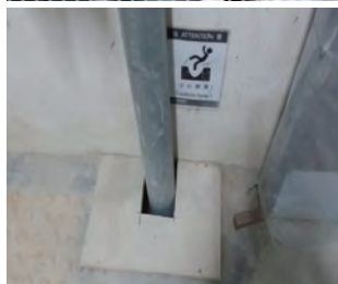
封蓋好的樓洞需要貼上警告標示 Cover to the floor opening securely fixed with warning notice
