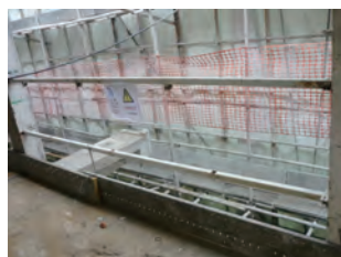
設有防護圍欄的外間開口 External opening provided with protective barrier
