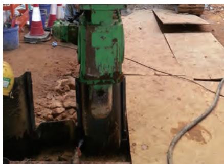
利用隔音罩減少噪音 Reduce noise by means of noise barrier
