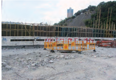
在樓面地台開口位置，應豎設圍欄防止物料下墮 Hole/opening on the demolishing floor should be protected with fencing from falling object
