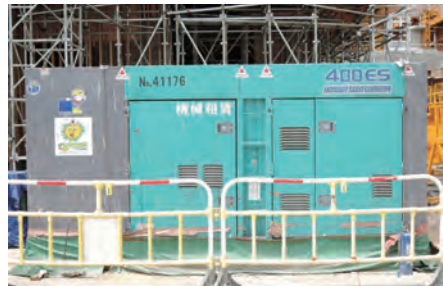
設置欄杆以防止有人容易地闖進低電壓設備的範圍 Railing to restrict unauthorized access to working zone of low voltage equipment.
