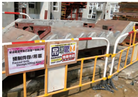
妥善放置貯存及圍封預製樓梯 Precast concrete staircases properly stored/fenced off
