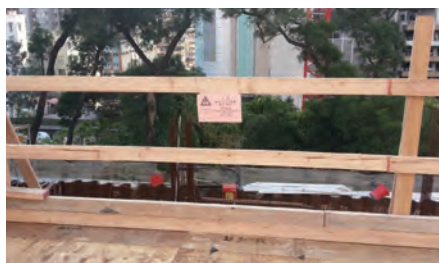
樓邊位置安裝有適當的木製圍欄 Proper timber guard rail along edges of working floor
