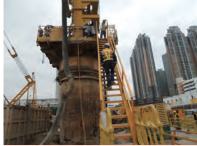
提供有扶手的樓梯往返工作平台 Provide staircase to working platform
