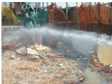
在工地灑水以減少塵埃飄散 Spraying water to reduce the risk of spreading dust from the works site
