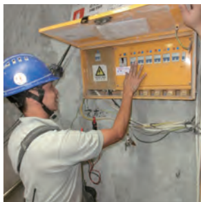
在消除故障後，只有註冊電工方可重設配電箱內的開關 Only Registered Electrical Worker allowed to reset the switch of distribution board after fault rectification
