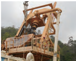
穿上防墮裝置的工人在設有護欄的工作平台上操作機械 Barrier and fall arrest system for workers working at height
