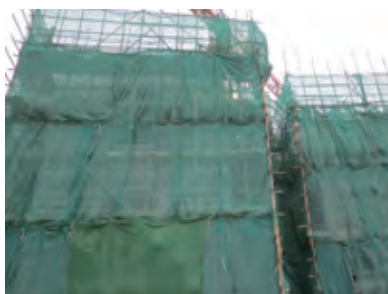
保護幕應覆蓋整個外牆棚架 Entire bamboo scaffolds should be covered with protective screen
