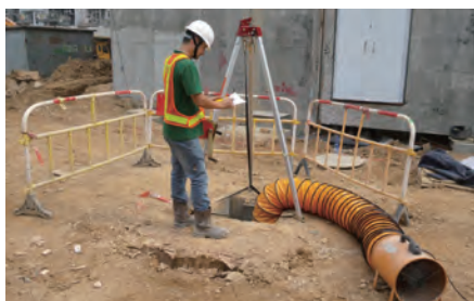
機械通風系統需為密閉空間抽入足夠的鮮風 Fresh air supply via mechanical ventilation system to a confined space
