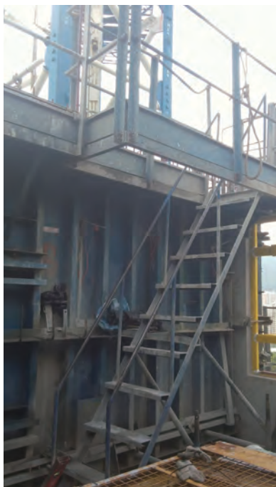
兩旁設有扶手的固定式鋼梯 A steel ladder (fixed type) with handrail on both sides.
