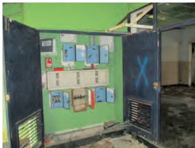
拆卸工程前，要求電力公司必需把主供電截斷 Prior to demolition, the main power supply must be dead and disconnected by Power Company
