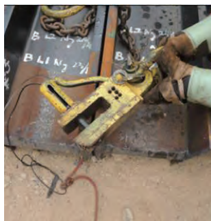
可扣緊工字樁末端的特製起重裝置 Lifting gear tailor designed to clip the end of H-pile
