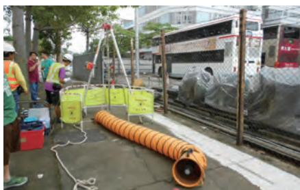
為深井提供機械通風系統 Deep well provided with mechanical ventilation
