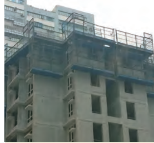
在工作平台邊緣安裝護欄 Guard-rails installed to perimeter of large steel formwork
