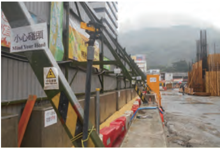
防止塵埃四散的自動灑水系統 Automatic water spraying system to control dust
