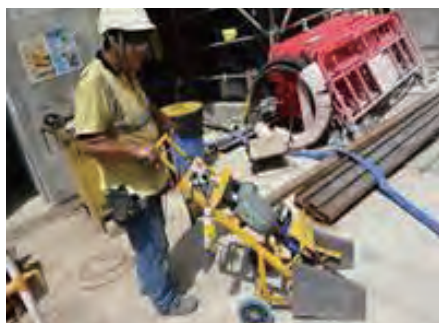
輔助運輸工具可減少體力處理操作時的危害 Use of semi-automatic breaker rack to reduce manual handling operation
