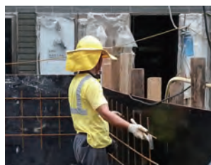
工人戴上配有遮陽設備的安全帽在陽光下工作 Worker with sunshade facility working under sunlight
