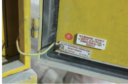
金屬可導電部份如門，須由等位電線接地，並掛上標籤牌（安全接地終端 - 切勿移去） Bonding conductor should be connected to the metal door with warning label "safety electrical connection - do not remove"
