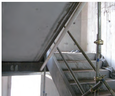
樓梯設置 Guard-rails along staircase
