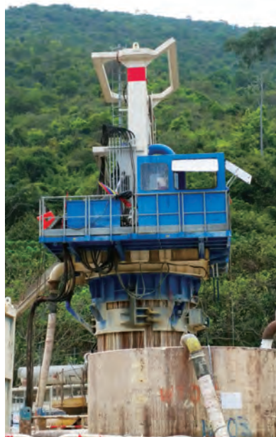
為大口徑鑽樁工程進行高空工作的操作員／ 工人應有安全措施提防從高處墜下 Large diameter bored pile with operators / workers working at height-to be cautious of hazard of falling from height
