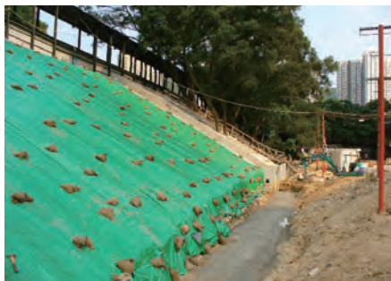
在斜坡底設 U 形排水道，並用防水布保護斜坡面 Provide U-channel at toe of cutting and cover slope surface with tarpaulin
