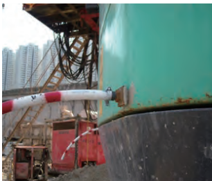
圍封工作地區及為移動機械安裝防撞棒 Fence off works area and provide warning rod on moving plant
