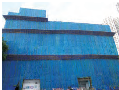
利用保護幕和以塑膠或柏油帆布製造的隔塵網，圍封整幢須拆卸的建築物，再搭建中層斜棚。 Building to be demolished to be fully enclosed by protective screen and dust screens of plastic or tarpaulin sheet, with intermediate catch-fans
