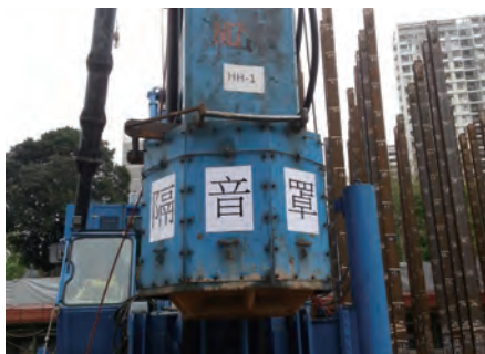
利用隔音罩減少噪音 Reduce noise by means of noise barrier
