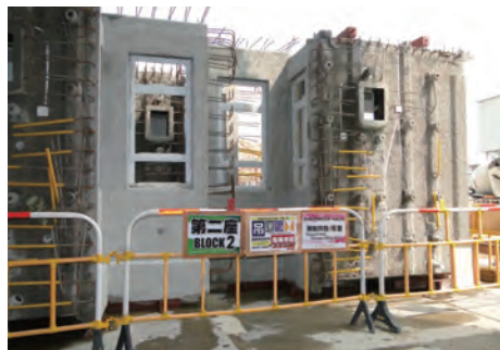
妥善放置貯存及圍封預製組件 Precast concrete unit properly stored
