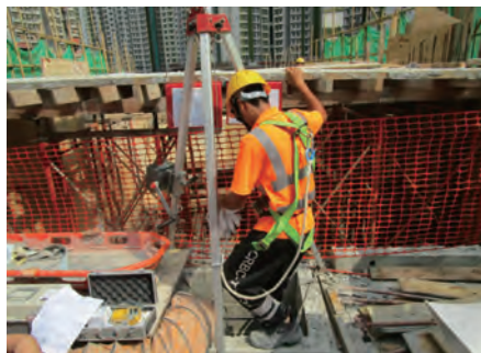
工人進入密閉空間前，應把全身式安全帶和救生繩繫穩。 Full-body harness and lifeline securely fixed before entering a confined space
