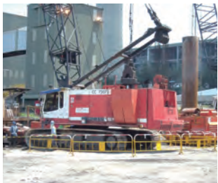
圍封工作地區及為移動機械安裝防撞棒 Fence off works area and provide warning rod on moving plant
