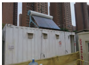
太陽能熱水系統（左圖）為淋浴室（右圖）提供熱水供應 Solar water heating system (left) to provide hot water to shower room (right)
