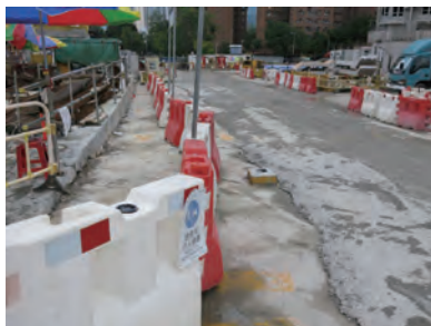
在硬地以重型圍欄分隔行人和車輛 Heavy duty barrier to separate pedestrians and vehicles on a hard paved road
