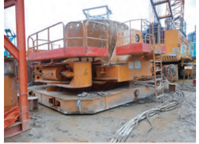
維持一個適當高出工作平台的鐵筒可防止意外下墮 Maintain a suitable height of casing above the working platform
