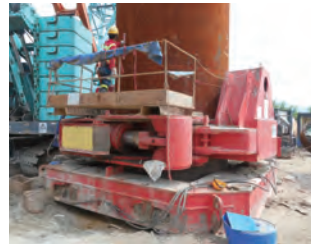
設有護欄的工作平台 Working platform with railings for workers working at height
