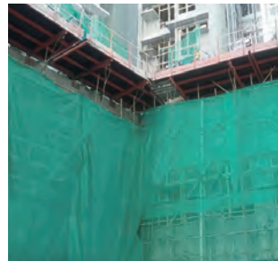
棚架須要合資格人員檢查，並須把填妥的表格5貼於棚架顯眼的位置 A scaffold should be inspected by competent person with a duly signed Form 5 posted on a conspicuous space
