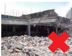
缺乏支撐的橫樑 No support to beam
