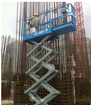
工人操作及使用動力操作升降工作平台時，須穿上全身式安全帶並繫穩於工作平台上指定的牢固點上 Worker needs to wear safety harness attached to a designated anchor point of the mobile elevating work platform when the platform in operation.
