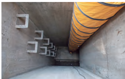
為深井提供機械通風系統 Deep well provided with mechanical ventilation
