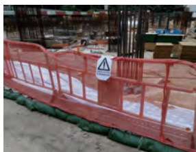
在挖掘工程邊緣設置的圍欄和土堤並掛上的警告標誌 Barrier with warning sign and earth bund along the edge of the excavation
