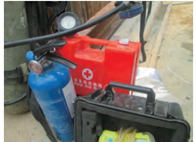
在密閉空間入口附近設置的急救箱和滅火器具 Provision of first aid box & fire-fighting apparatus near the entrance of a confined space
