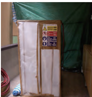
以帆布完全圍封石棉工程範圍 Full enclosure of asbestos work zone by canvas sheet
