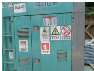
於電力裝置張貼足夠及合適的安全告示 Adequate notice should be posted to the electrical installation
