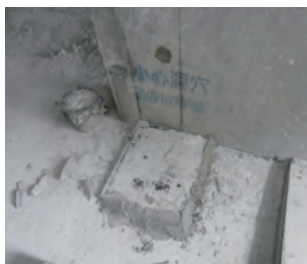
臨時以水泥封蓋好的樓洞 Properly cover floor opening
