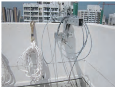
天台上的吊船設備。救生繩以布料、塑膠套管或類似的方法保護，以免被尖角損壞。 Facilities of gondola at roof. The lifeline is protected with fabric material, plastic tube or similar means to prevent damage by sharp corner.
