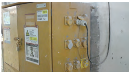
最終電路不得有電纜接頭 No cable joint in the final circuits
