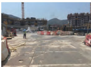
灑水以免塵土飛揚 Dust control with water spraying
