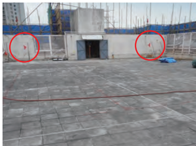
移動拆卸機械在紅旗標示的範圍內，可安全進行作業 Red flags set up to demarcate the restricted area for safe operation of moving machinery
