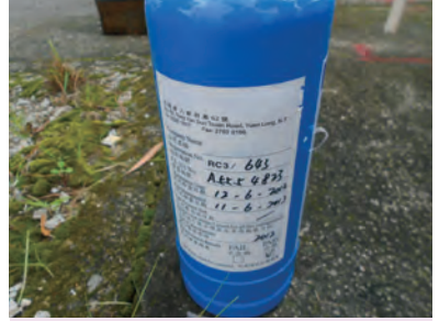
在密閉空間附近設置滅火器具 Provision of fire-fighting apparatus near a confined space
