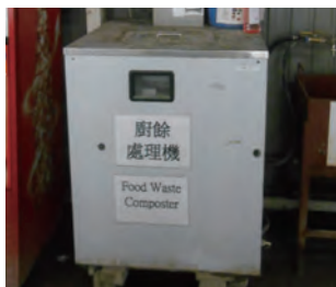
地盤收集廚餘的處理機 A typical food waste composting machine
