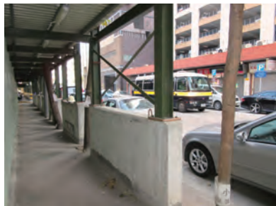
在圍板和有蓋行人路提供臨時照明，以方便行人。 Hoarding and covered walkway with adequate temporary lighting for pedestrian
