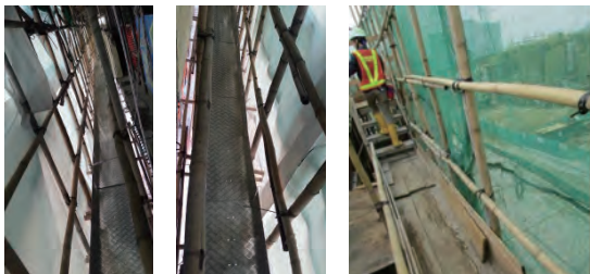
棚架上的工作平台須由踢腳板、中及高欄和密鋪的橋板路組成 Intermediate and top guard-rails with toe board plus closely planking form a working platform on scaffolding
