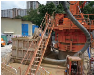
另一設置扶手的樓梯，供通往工作平台 Provide handrails to staircase leading to working platform
