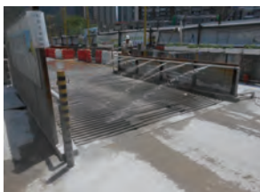
車輪清洗處的噴水器正在運作 Operation of water-jet in a vehicle wheel – washing area
