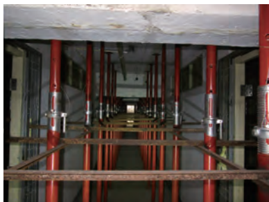
提供支撐和支柱承托須拆卸的建築物 Shoring and propping for buildings to be demolished
