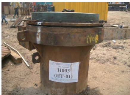
整個打樁過程須使用膠墊以減少噪音 Plastic cushion to reduce noise generated during the course of piling
