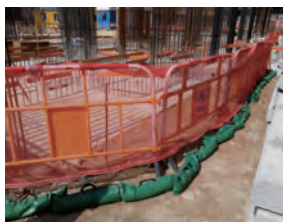
在挖掘工程邊緣設置的圍欄和土堤並掛上的警告標誌 Barrier with warning sign and earth bund along the edge of the excavation
