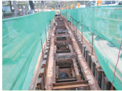
為深度超過1.2米的挖掘溝槽提供支撐設施 Shoring support to excavation with depth greater than 1.2m
