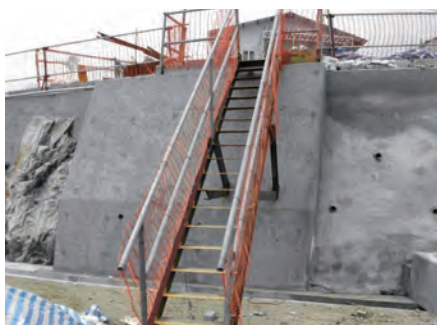
提供樓梯方便進出挖掘工地／斜坡 Provide staircase for access to and egress from mass excavation/slope
