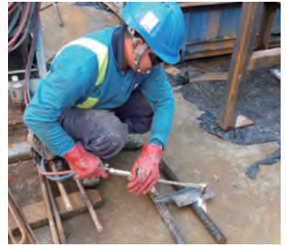
在火焰切割工作時，焊接工人應佩戴合適的個人防護裝備 Welder should put on adequate personal protective equipment during the course of flame cutting works
