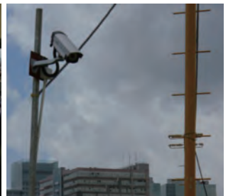
安裝閉路電視系統監察拆卸工地的各個區域。 CCTV system to monitor various areas of the demolition site.
