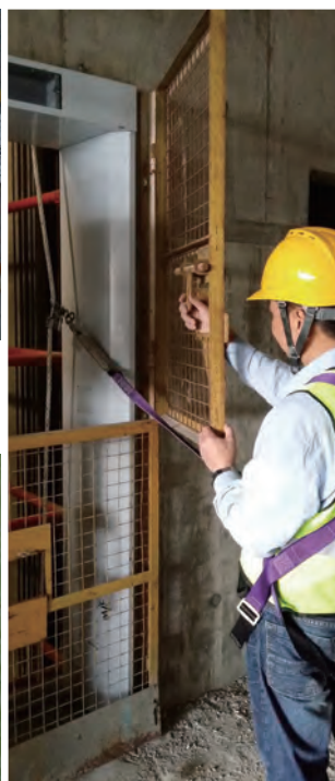
當需要進入升降機槽或井底工作時，工人必需將隨帶吊繩緊固於獨立救生繩 Worker should attach the lanyard to the independent lifeline before making access to lift pit/shaft
