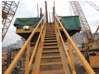
為工作平台提供的護欄和踢腳板 Provide barrier and toe-board to working platform
