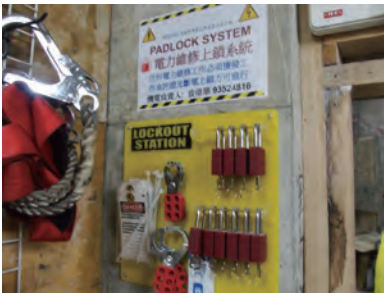
一套齊全的工地電力上鎖系統 A well equipped padlock system of a construction site
