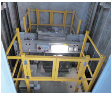
升降機頂上的工作台設有圍欄及踢腳板 Working platform with railing and toe board on lift car top
