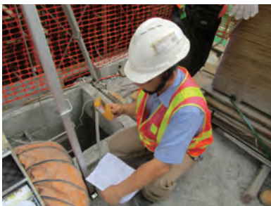
安全主任應在工作許可證上記錄空氣測試結果 Safety officer records the results of air test of a confined space in the certificate
