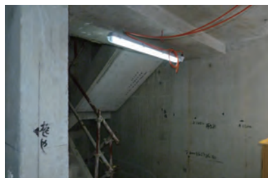
電力裝置（例如照明裝置和電線）盡安裝於離地面至少兩米高處 Electrical installations such as lighting & wiring to be mounted/fixed at high level ( \geq 2\text{m} )
