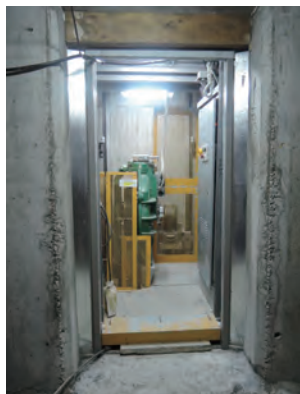
升降機槽內的建築工地升降機臨時機房 Builders' lift cathead inside lift shaft
