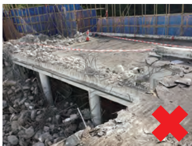
沒有妥善圍封／承托拆卸工程範圍 No proper fencing/support to demolition areas
