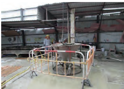
簡單圍欄可防止意外發生 Fencing off lifing appliance to prevent accident
