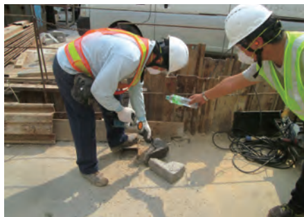
使用手提氣動碎石機時佩戴全套個人防護裝備，例如護耳罩、安全鞋、頭盔、眼罩、手套、口罩等。 Full personal protective equipment such as ear muff, safety shoes, safety helmet, goggles, gloves, mask, etc. for using handheld pneumatic breaker
