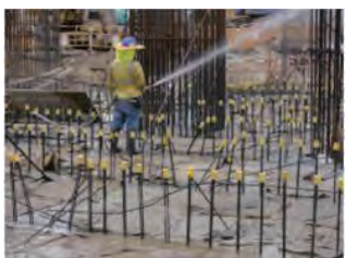
以鋁槽和膠蓋覆蓋金屬枝 Aluminium trough and plastic caps to cover the metal bars
