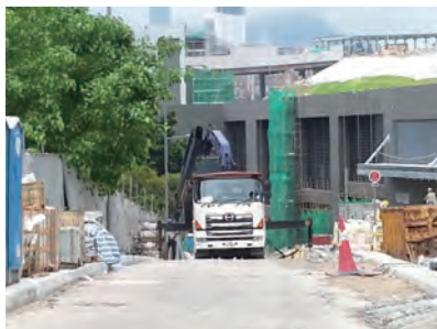
當隨車式起重機運作前，其支重腳撐應完全伸展及其蹯板正確放在起重墊板上 Lorry-mounted mobile crane under operation should fully extend the outrigger legs
