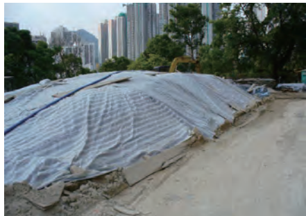
用防水布為斜坡提供適當的保護 Protect slope with tarpaulin cover
