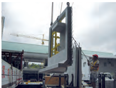
穿上反光工作服、配合安全頭盔及手套等才可進行工作 Reflective clothing, safety helmet, gloves, etc. in place for lifting works at height
