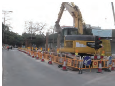
以重型建築機械及圍欄確定出安全工作地帶 Work safety zone demarcated by construction machine and barrier
