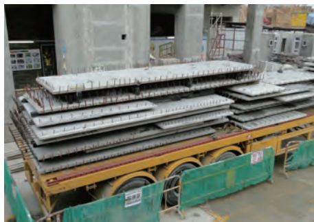
妥善圍封未下架的預製樓面板 Loaded precast concrete slabs are properly fenced off
