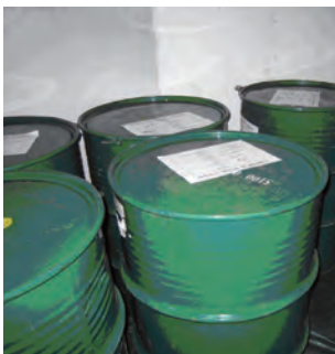
貯存石棉廢物於容器內，並加上標籤 Containers for asbestos waste and stuck with label
