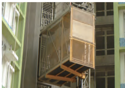
升降機吊籠要有足夠圍封 Substantial enclosure to builder's lift car cage
