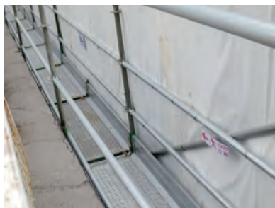
設有金屬橋板、金屬踢腳板、頂部護欄和中間護欄的工作平台。 Working platform with metal plate, metallic toe board, and top and intermediate guard-rails
