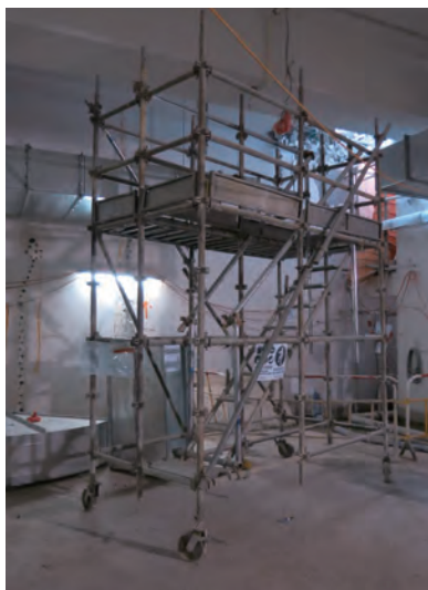
設有輪子鎖定裝置的流動工作平台 Mobile working platform fitted with castors locking device
