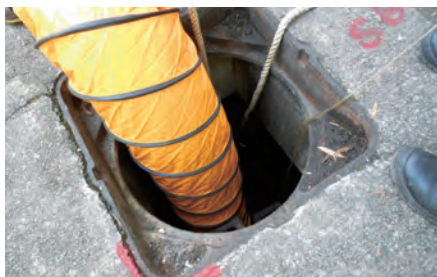
在密閉空間入口提供機械通風／救生繩 Mechanical ventilation/lifeline provided at the entrance fo confined space
