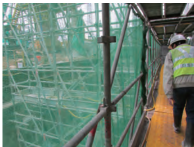
工作平台應設有踢腳板、頂部護欄和中間護欄 Working platform with toe board, top and intermediate guard-rails
