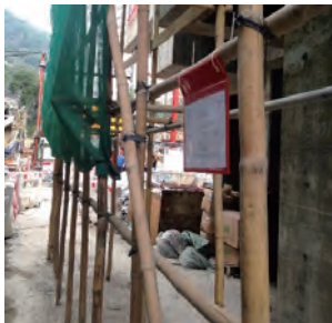
棚架須要合資格人員檢查，並須把填妥的表格5貼於棚架顯眼的位置 A scaffold should be inspected by competent person with a duly signed Form 5 posted on a conspicuous space
