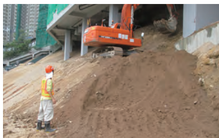
為挖土機操作員安排訊號員 Signaler works with the excavator operator
