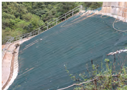
在斜坡底設 U 形排水道，並用防水布保護斜坡面 Provide U-channel at toe of cutting and cover slope surface with tarpaulin
