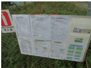
在密閉空間外的當眼處應展示風險評估報告、工作許可證、安全設施檢查清單和核准工人／合資格人士證明書 Risk assessment report, permit-to-work certificate, safety facilities checklist and certificate of certified worker/competent person displayed in a conspicuous location outside a confined space
