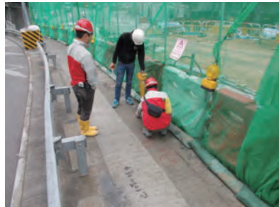
以探測器和量度工具等去確定地下公用設施的位置 On site identification for existing underground utilities with detector and measuring instrument
