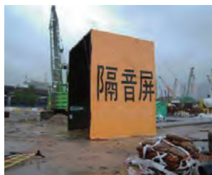
為建築地盤設置隔音屏 Noise screen provided for construction site
