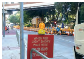
為行車道上的工程採取臨時交通安排 Temporary traffic arrangement for work carried out on carriageway
