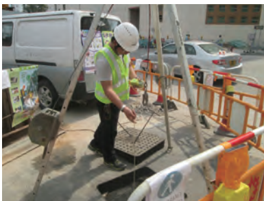
安全主任以氣體探測器測試密閉空間內的空氣成份 Safety officer uses multi-gas detector to conduct air-testing of the confined space
