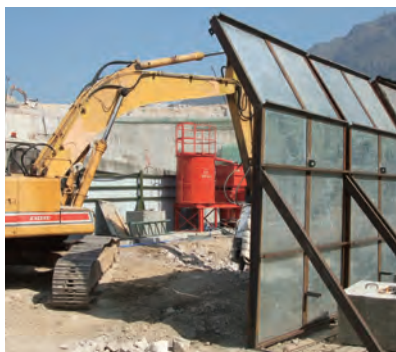
進行岩石挖掘工程時設置隔音屏。 A noise screen is provided during rock excavation.
