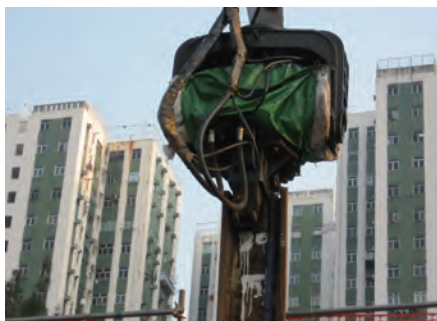
利用震鎚減少打閉板樁產生的噪音 Noise attenuation using vibration hammer during sheet piling installation
