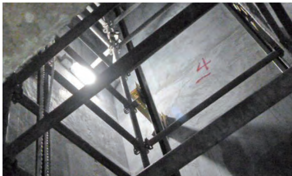
升降機槽中有充足的照明 Sufficient lighting for works in the lift shaft
