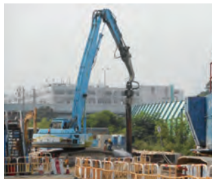
圍起施工範圍防止工人意外墮入洞穴 Fencing off works area to prevent accidental fall into holes
