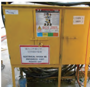
在消除故障後，只有註冊電工方可重設配電箱內的開關 Only Registered Electrical Worker allowed to reset the switch of distribution board after fault rectification
