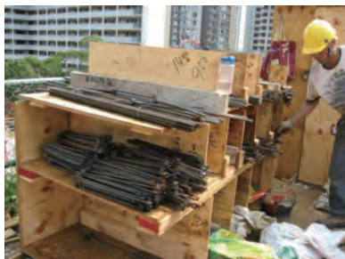
2S – 工地材料放置整齊 2S – An orderly storage of materials
