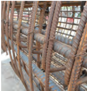
紮結鋼筋籠的鐵線應朝籠內方向 Tying wire to reinforcement casing arranged to point inside
