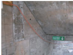
一般電線，如在走廊或樓梯應在高位掛定 Fixing the cable at high level in corridor, staircase
