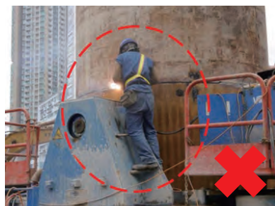
工人沒有適當保護引致人體從高處墜下的 風險 Hazard of fall of person from height due to lack of fall protection measure
