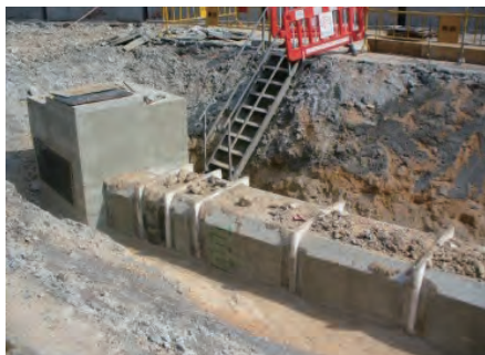
提供臨時樓梯，以供安全進出挖掘工地 Temporary staircase for a safe access/egress from excavation
