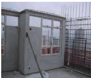
為外牆安裝支撐托架 Install supporting bracket for facade
