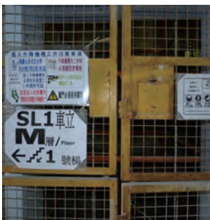
在閘門上張貼足夠的安全／警告告示 Sufficient safety/warning notices and permit-to-work posted to barrier
