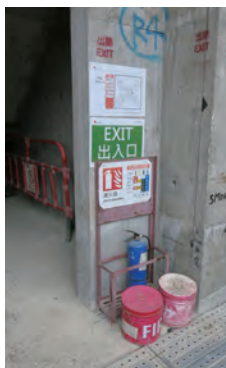
在標準樓層提供滅火筒和沙桶 Provision of fire extinguisher and buckets of sand on typical floor
