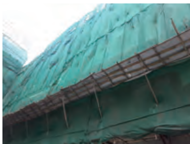
斜柵應從建築物外棚向外伸延1,500毫米 Catch-fan projected at least 1,500mm horizontally from the scaffolding
