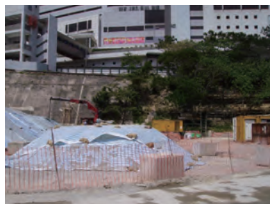
挖掘的物料應妥善遮蓋及圍封 Excavated material should be properly covered and fenced off
