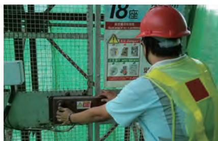
物料吊重機進行安全檢測 Perform regular safety checking/inspection to material hoist
