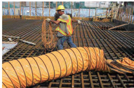
天氣炎熱時，為大型樁帽內的工作間提供機械通風 Mechanical ventilation is provided to a working area inside a large pile cap during hot weather
