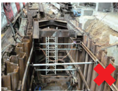
未有於泥坑提供安全進出通道引致工人墜下泥坑的危害 Hazard of fall of person into excavation due to unsafe access
