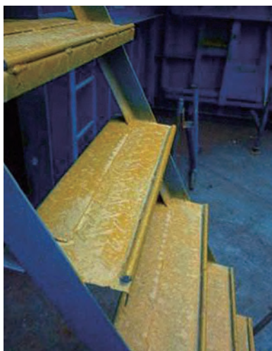
梯子級面加上金屬杆，增強防滑效果 Access staircase with additional steel rod as anti-slip device
