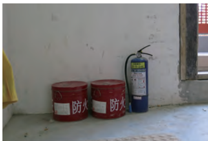
在標準樓層提供滅火筒和沙桶 Provision of fire extinguisher and buckets of sand on typical floor
