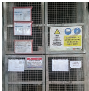
在閘門上張貼足夠的安全／警告告示 Sufficient safety/warning notices and permit-to-work posted to barrier
