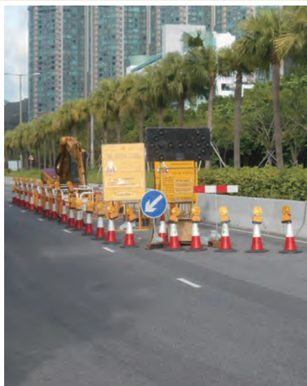
進行接駁地下公用設施至地盤的工程時，在行車道用圓錐筒／燈具圍起施工範圍 Fencing off the works area with cones/lanterns at carriageway for underground utilities to be connected to the construction site
