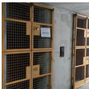
安裝全高度四扇金屬閘門，防止工人擅闖升降機槽。 Full height 4-leaf metallic gate to restrict unauthorized access to lift shaft
