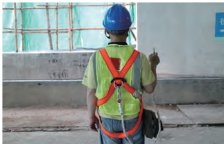
全身式安全帶 (背面) Back view of a full-body safety harness
