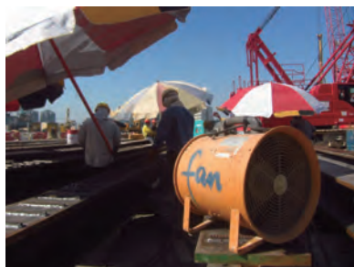
使用風扇／吹風機保持工作地點空氣流通 Adequate ventilation for the works area by fans or blowers
