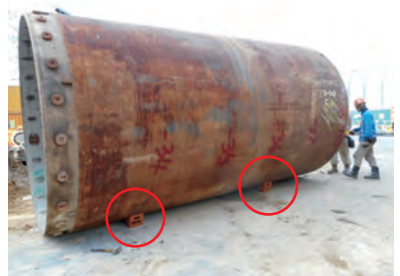
在大型圓形鋼套管底部放置楔子 Provide proper wedges at bottom of large circular steel casing
