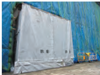
為拆卸工程範圍提供隔音屏障 Noise screen provided for demolition works
