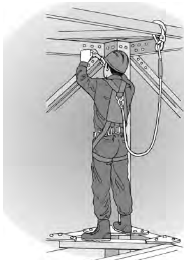
工作前應將隨帶吊繩繫於牢固點 Tie the lanyard to anchorage point securely before works commencement
