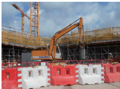
設有吸音裝備的氣壓碎石機 Pneumatic breaker equipped with noise absorber
