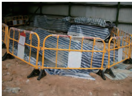
深坑的斜面蓋上塑膠布料，以免受天氣影響 Profile of slope of a deep excavation is protected from weather with PVC sheet
