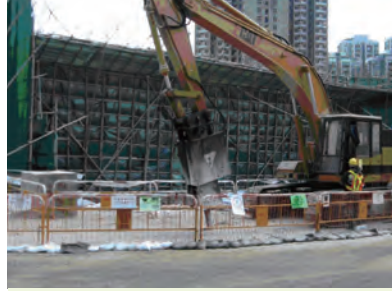
為免大量地面水流進土坑，挖掘工程的邊緣應放有土堤或沙包等 Provide earth bund or sand bags along edge of excavation to curb surface water run off
