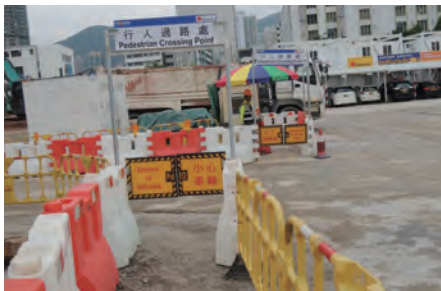
在硬地以可摺合的圍欄分隔行人和車輛 Folding type barrier to separate pedestrians and vehicles on a hard paved road
