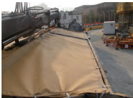
以膠布覆蓋卸泥貨車，以防易生塵埃的物料飛散 Dump truck with PVC cover to prevent spread of dusty materials
