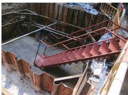
提供樓梯方便進出挖掘工地／斜坡 Provide staircase for access to and egress from mass excavation/slope
