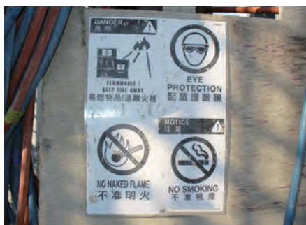
氣體焊接要注意的安全事項 Safety measures about gas welding
