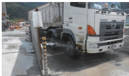
車輛清洗處正進行車輪清洗 Wheels of a vehicle under cleaning in a washing bay
