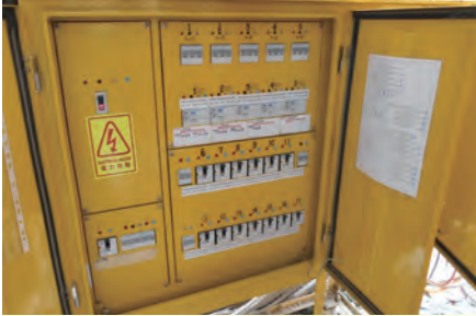
典型配電箱（屏）都裝置電路保護器如MCB/RCD Typical distribution board with circuit protection device as MCB, RCD
