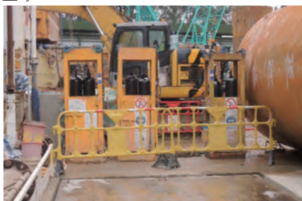
乙炔氣瓶和氧氣瓶須貯存在有良好通風的地方 Store the acetylene and oxygen cylinders in a well ventilated area
