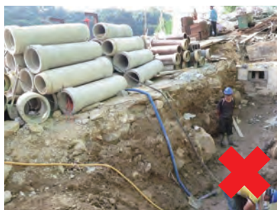
遭墜下溝槽的物件擊中的危害 Hazard of being struck by materials falling into trench
