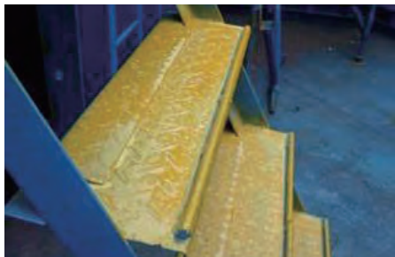
於梯級加裝鋼棒，有助防滑 Additional steel rod on the staircase as anti-slip device
