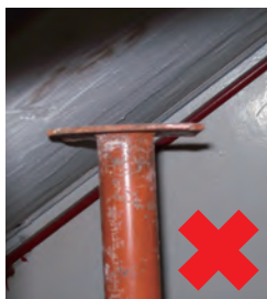
撐桿未有貼緊樓底 Props do not support the bottom of ceiling
