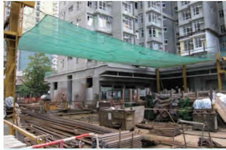
為紮鐵工地提供保護網 Safety net provided above steel bending workplace
