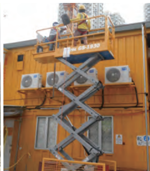
動力操作升降工作平台四邊裝設護欄，避免工人發生意外而受傷 Mobile elevating work platform fitted with guard on four sides for protection of workers from accident
