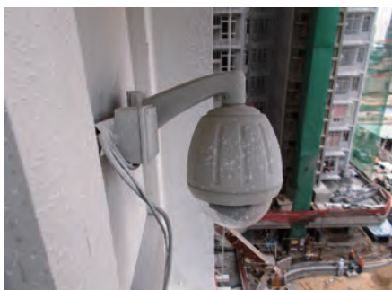
閉路電視攝錄機設置在吊運區上方，協助塔式起重機操作員進行吊運操作 CCTV camera with recording function positioned above lifting zone to assist tower crane operator to carry out the lifting
