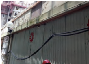
室外電線，應在高位掛定 Fixing the outdoor cable at high level
