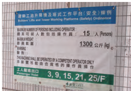
建築工地升降機旁需有展示載人數目的告示 Capacity displayed adjacent to entrance of a builder's lift
