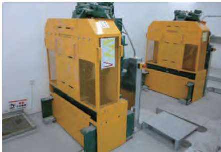
升降機或電動絞車必需安裝護罩 Guard provided for lift machines and electric winch
