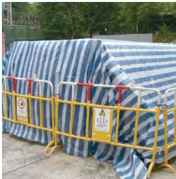
妥善遮蓋／堆放物料 Properly covered/stacked materials
