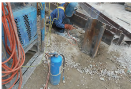
在燒焊地點附近提供輕便的手提滅火筒 A portable fire extinguisher provided near the welding spot
