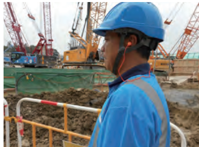
在噪音環境下工作應佩戴合適的護耳罩或耳塞 Suitable ear muff or ear plugs adopted in a noisy working environment
