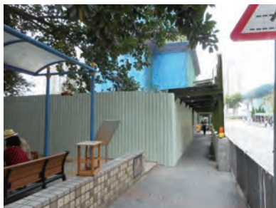
沿地盤界線的圍板和有蓋行人路設置墜台，以保護行人。 Hoarding and covered walkway with catch platform along the site boundary to protect pedestrian
