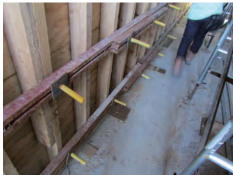
對突出的螺栓作好防護 Protection for projecting bolts
