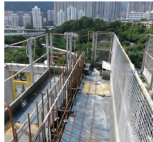
工作平台護欄以金屬絲網圍封 Parapet wall of a working platform is fenced with wire mesh
