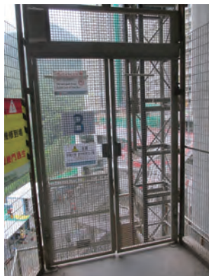
建築工地升降機裝有全高度的閘門 Full height gate for a builder's lift
