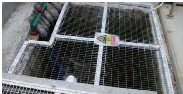
臨時以水泥封蓋好的樓洞 Properly cover floor opening
