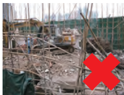
棚架損毀 Damage of scaffolding
