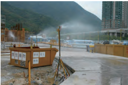
在運料路上灑水，防止塵埃四散。 Dust control by water spraying over the haul road
