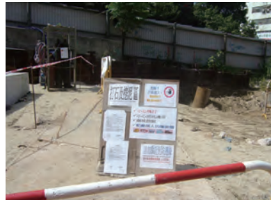
挖泥區放置圍欄及警告告示 Barrier with warning notice to excavation
