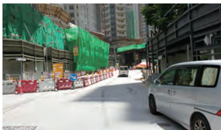
連接地盤入口處的路障，組成連續的路障 Barriers linking up to form a continuous barrier at site entrance
