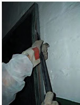
Respiratory protective equipment and protective clothing used for asbestos abatement work
