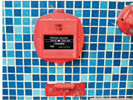
Weatherproof type break glass unit at outdoor locations
