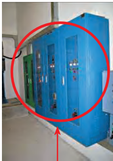
Double doors / enclosure for control panels inside pump rooms
