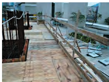
Working platform provided for steel fixing works at heights ( \geq 2\text{m} )
