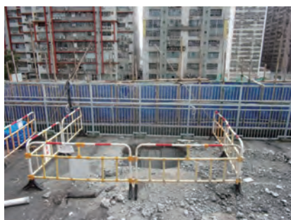
Barrier erected at the opening of refuse chute. Scaffold and nylon mesh at the building perimeter must be higher than the floor level by 1 meter
