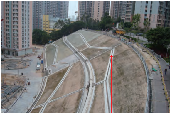
Slope surface drainage system
