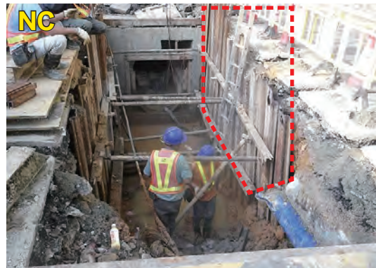
Inadequate safe access
