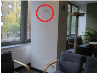
Anchorage (eyebolt on wall) for fall arresting system for routine maintenance
