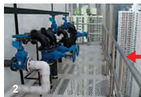
Maintenance platform with safe and easy access to valves and pipes
