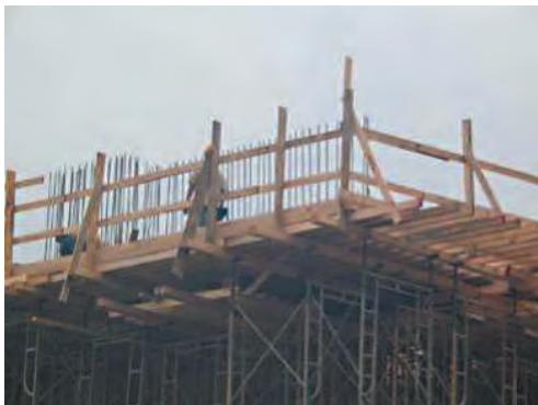
Working platform with adequate railings and toe boards was provided during working at heights
