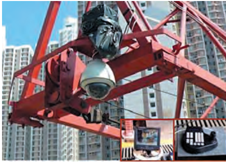
Tower crane CCTV, monitor and control panel
