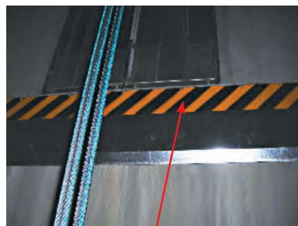
Warning stripes at the bottom of landing opening
