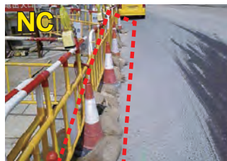
Should be free-standing (Bag filled with sand as ballast is not acceptable)
