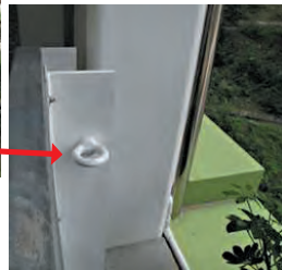
Fall Arrest System at planter on both sides of the footbridge
