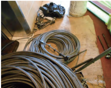
Replacement of suspension ropes
