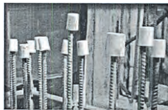
Injury caused by falling on unprotected protruded steel bars Protection of workers from injury using one of the protective options
