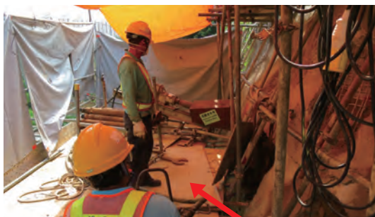
Temporary platform for soil nails works
