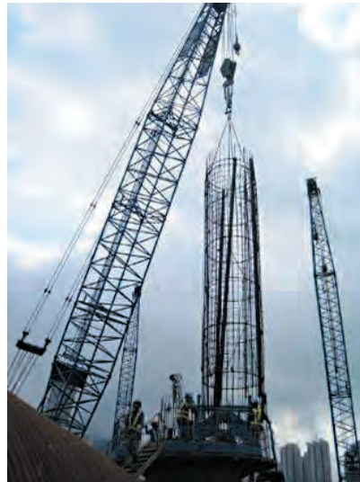
Lifting steel cage (vertical)
