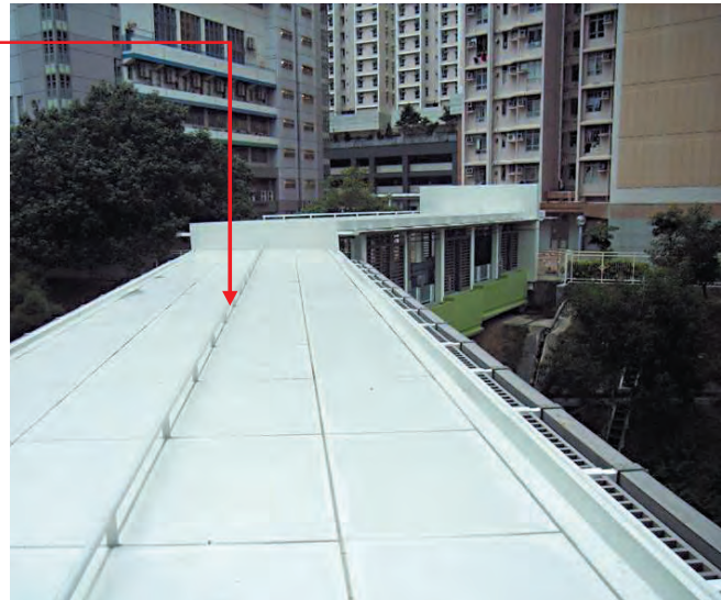
Footbridge with fall arrest system
