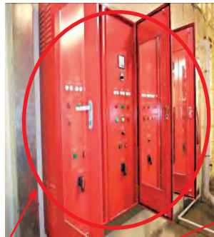
Double doors / enclosure for control panels inside pump rooms
