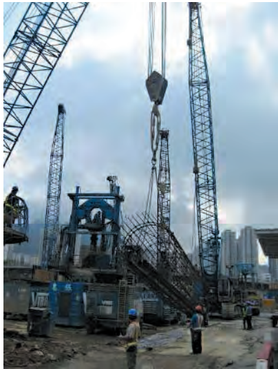
Lifting steel cage by 2 cranes (horizontal)
