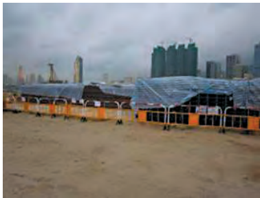
Proper storage of H-pile material
