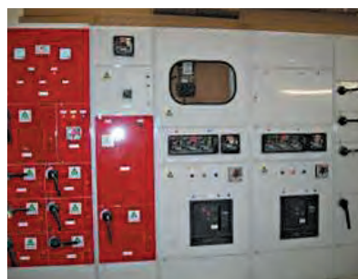
Modular design switchboards
