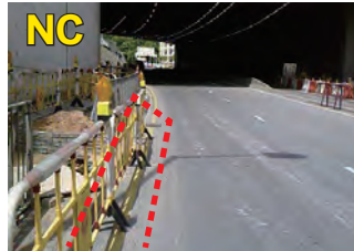
With continuous pedestrian barriers but without adequate traffic cone
