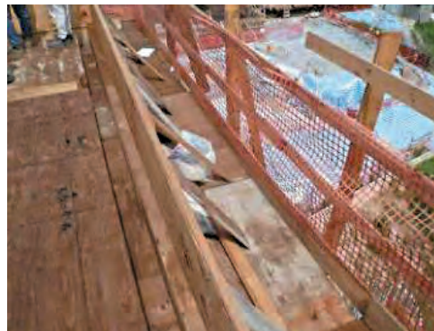
Working platform with adequate railings and toe boards was provided during working at heights
