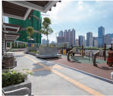
Tactile Guide Path and non-slip paving
