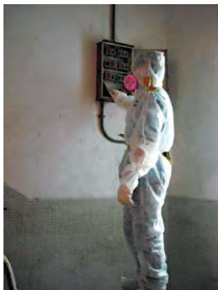
Asbestos removal works for fuse box
