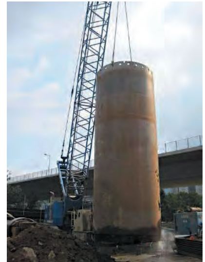
Lifting steel casing (vertical)
