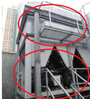
Provide permanent working platform with railings, toe-boards and access ladder for repair / maintenance of chillers on the roof
