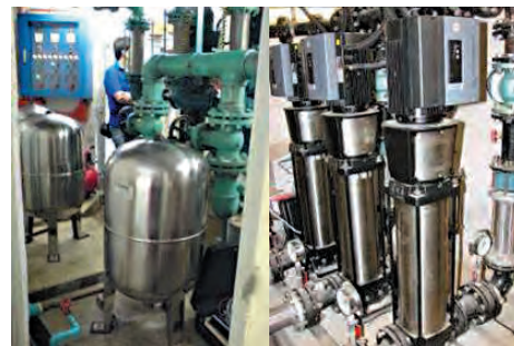
Small stainless steel pressure vessels with VSD control
