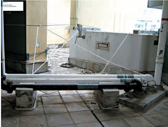
Previous arrangement – Two supports for one gondola holding down / fixing to roof floor
