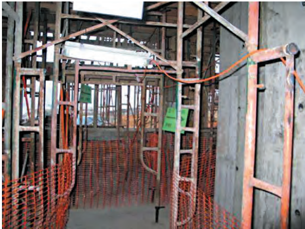
Adequate lighting and fencing off hazardous area
