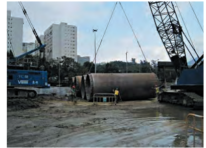
Lifting casing (horizontal)
