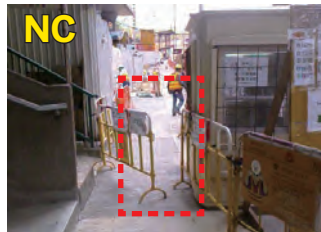
Barriers should be hooked / fastened to form continuous barriers
