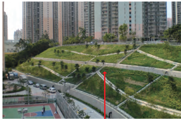
Hydroseeding slope surface protection
