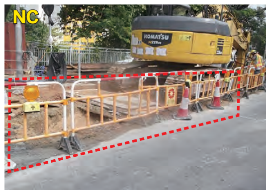
Traffic cone max. spacing 3m
