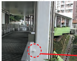
Fall Arrest System at planter on both sides of the footbridge
