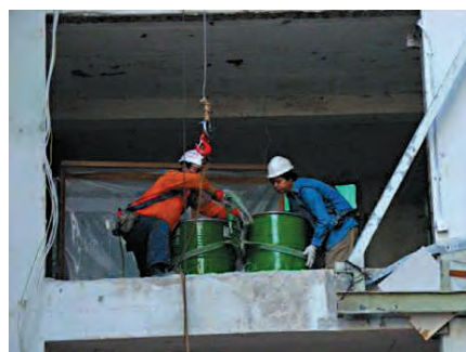
Transferring sealed drum to the ground
