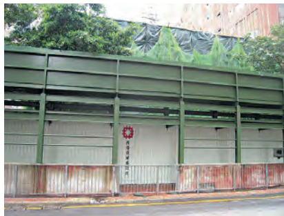
Double deck hoarding / covered walkway to protect pedestrians; locations and extent of hoarding should be clearly defined
