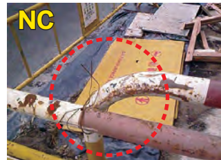
Barriers should be painted so that they stand out conspicuously in contrast
