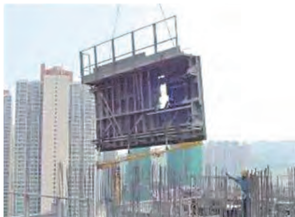
If rotary symmetry cannot be fully achieved, designated site crews should be assigned to look after every movement of formwork to ground level
