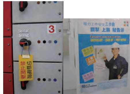
Properly isolate the source of electricity with lockout and tagout procedure
