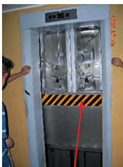
Warning stripes at the bottom of lift car
