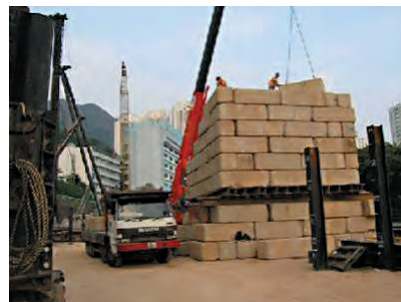
Typical concrete block kentledge
