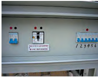
Circuit protective device (RCCB) provided for sockets for portable equipment
