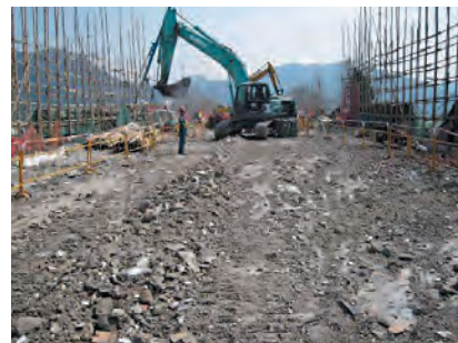
Stacking of demolished debris not to exceed allowable height. Debris is to be cleared from time to time
