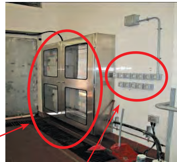
Weatherproof switch panels used in wet environments
