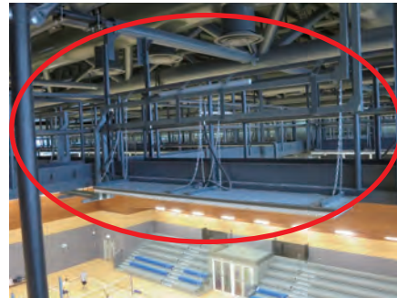
Provide working platform for repair / maintenance of building services installed at high level
