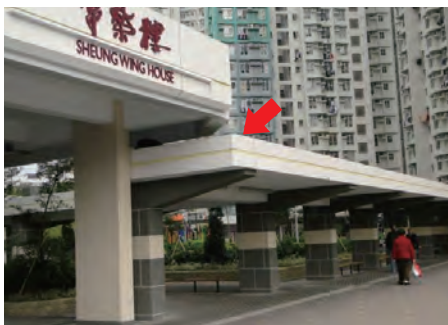
Provide pergolas for protection from the weather as well as from falling objects.
