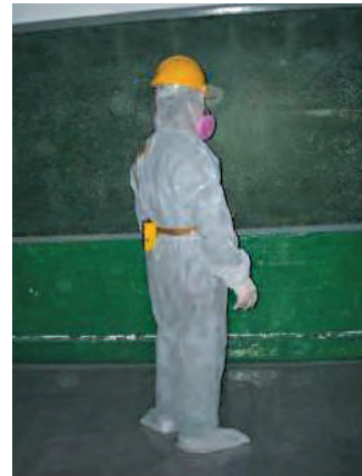
Respiratory protective equipment and protective clothing used for asbestos abatement work
