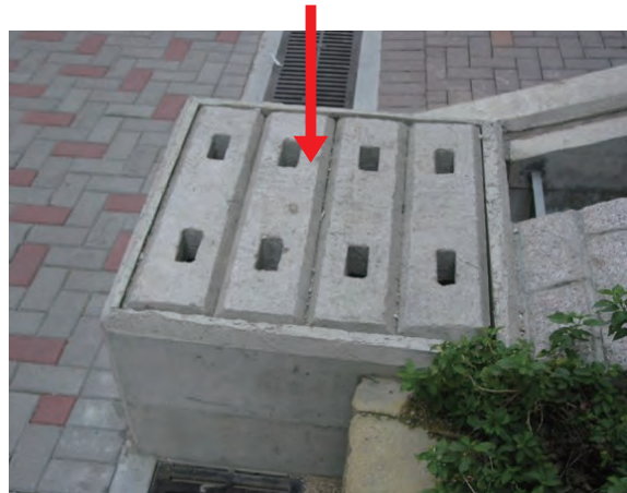
Catchpit covered up with concrete strips
