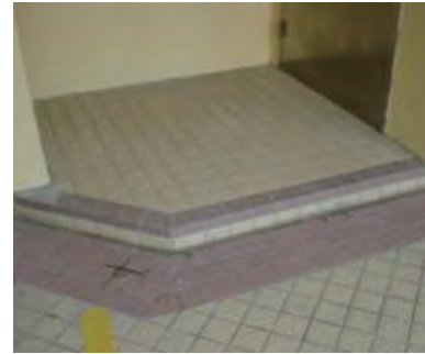
Non-slip nosing in contrasting colour
