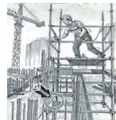
Injury caused by falling on unprotected protruded steel bars Protection of workers from injury using one of the protective options
