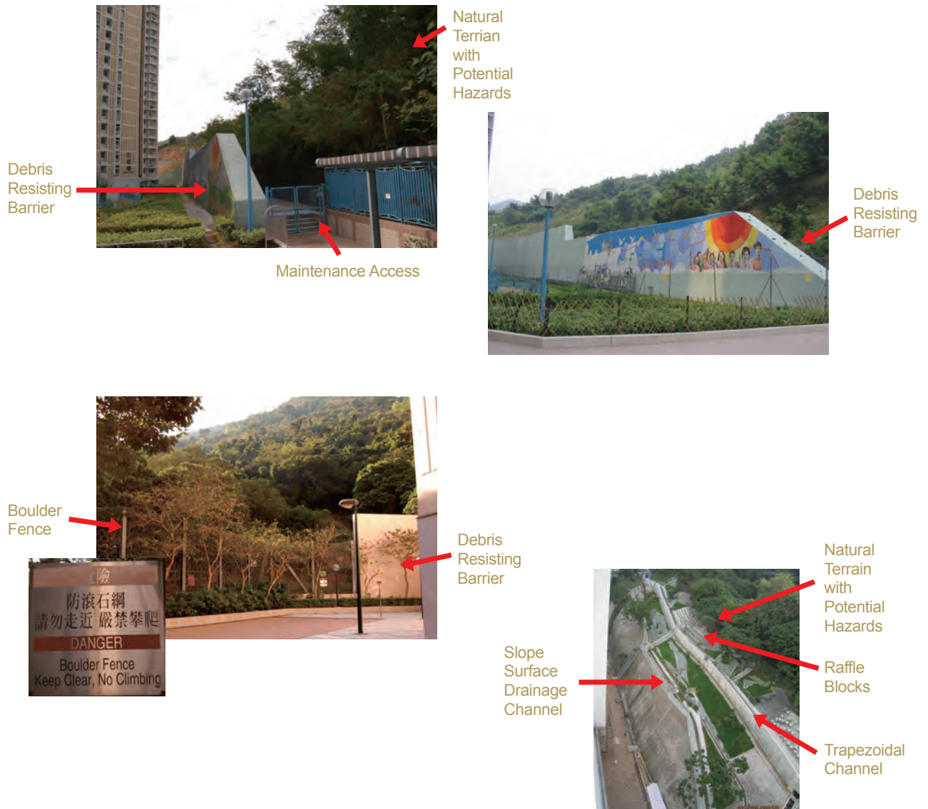
Debris Resisting Barrier with Maintenance Access to Protect Public Housing from Natural Terrain Hazards (Project: Sha Tin Area 4D)
