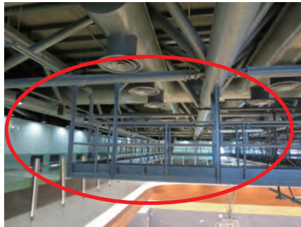
Provide working platform for repair / maintenance of building services installed at high level
