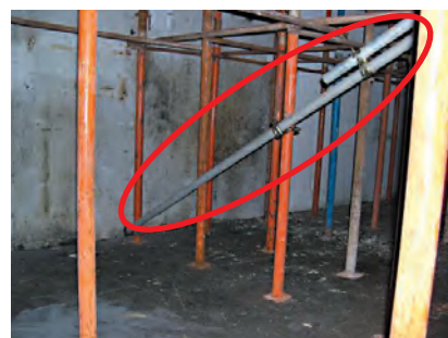
Clamping instead of tack welding to bracing should be specified in Demolition Plan; tack welding is difficult to assess for adequacy
