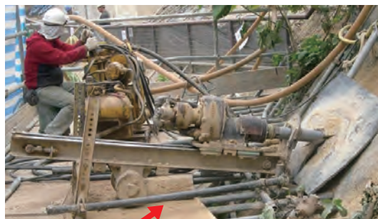
Temporary platform for soil nails works
