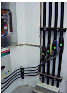
Prefabricated branch cable riser
