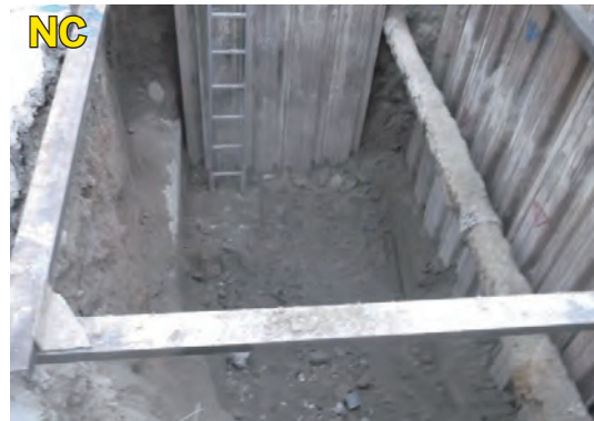
Inadequate support
