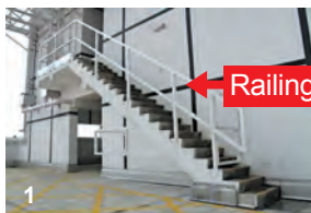
External stair from main roof to maintenance platform
