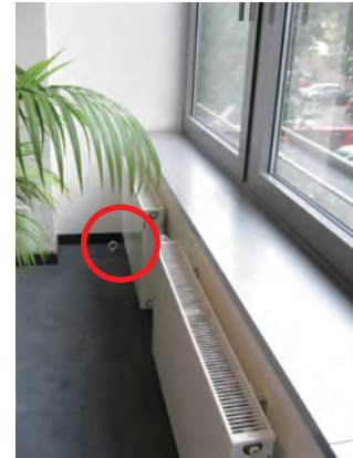
Anchorage (eyebolt on floor) for fall arresting system for routine maintenance
