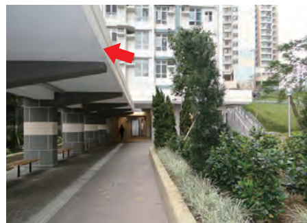
Covered walkways for protection from the weather as well as from falling objects.
