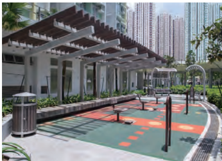
Provide pergolas for protection from the weather as well as from falling objects.
