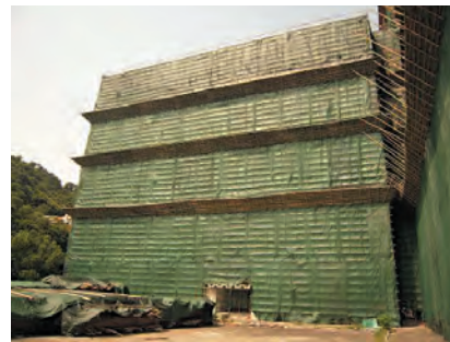
Scaffold, nylon mesh and periphery catch platforms / fans to prevent demolished debris from falling out of the block
