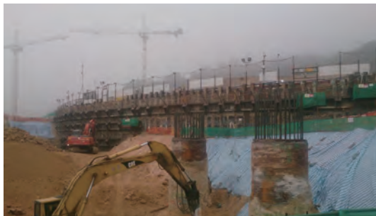
General view of Excavation and Lateral Support Work Using Temporary Ground Anchors
