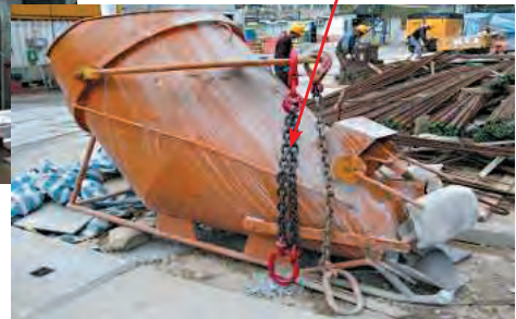
New design double chain sling for lifting of hopper
