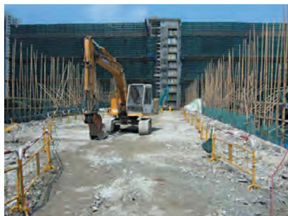
The route for movement of mechanical breaker must be defined in Demolition Plan. Adequate propping should be provided underneath
