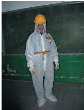
Respiratory protective equipment and protective clothing used for asbestos abatement work
