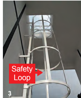
Cat ladder from maintenance platform to upper roof
