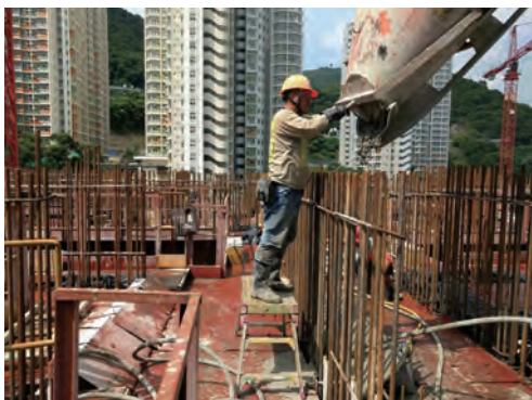
Hop-up platform provided for concrete pouring at heights ( < 2\text{m} )
