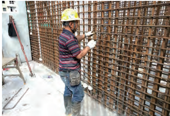
Fixing of fabric reinforcement
