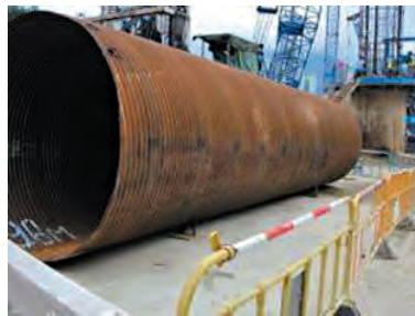
Proper storage of steel liner
