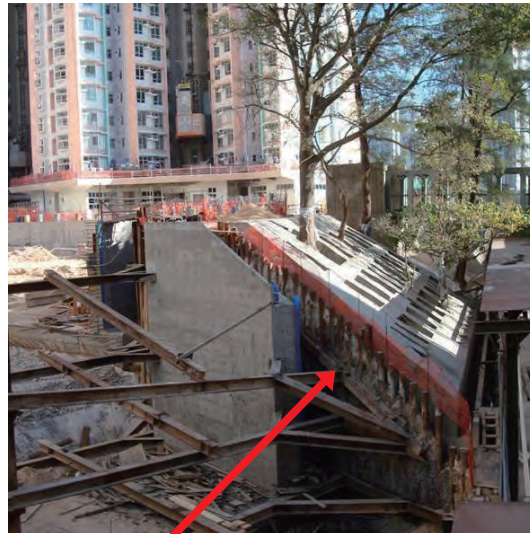
Temporary works for excavation works
