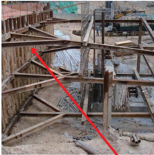
Temporary works for excavation works
