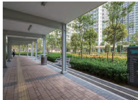
Covered walkways for protection from the weather as well as from falling objects.
