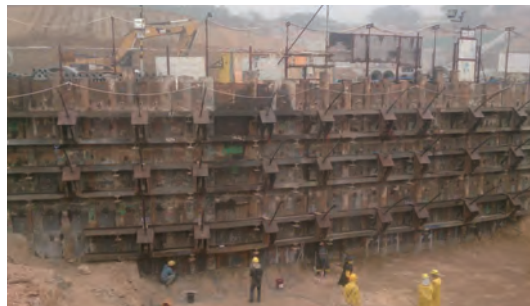
General view of Excavation and Lateral Support Work Using Temporary Ground Anchors
