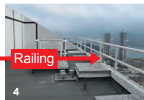
Upper roof with safe access to top of water tanks
