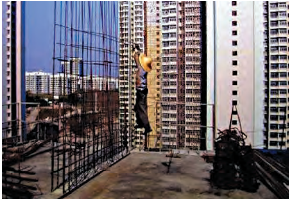
Traditional rebar fixing
