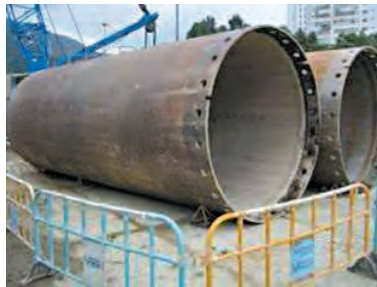
Proper storage of steel casing
