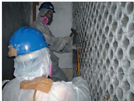
Asbestos removal works for grille panel
