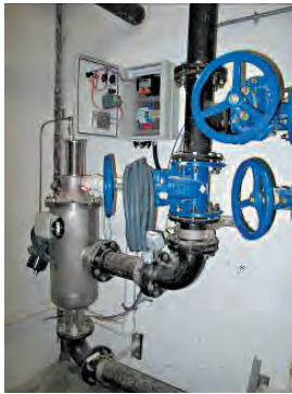
Provision of bucket type strainer in flushing water incoming pipe
