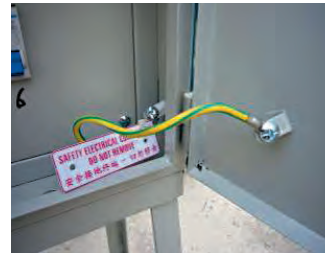
Effective earthing for all circuits / exposed conductive parts
