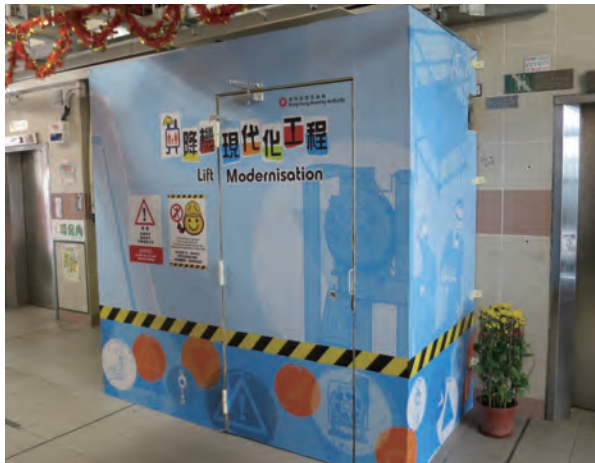
For lift modernization works - before dismantling the landing doors, provide full-height fire resistant boarding with an access door
