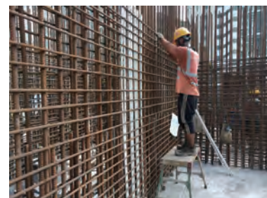
Hop-up platform provided for steel fixing works at heights ( < 2\text{m} )
