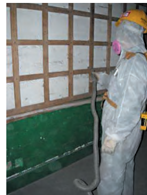
Asbestos particles removing
