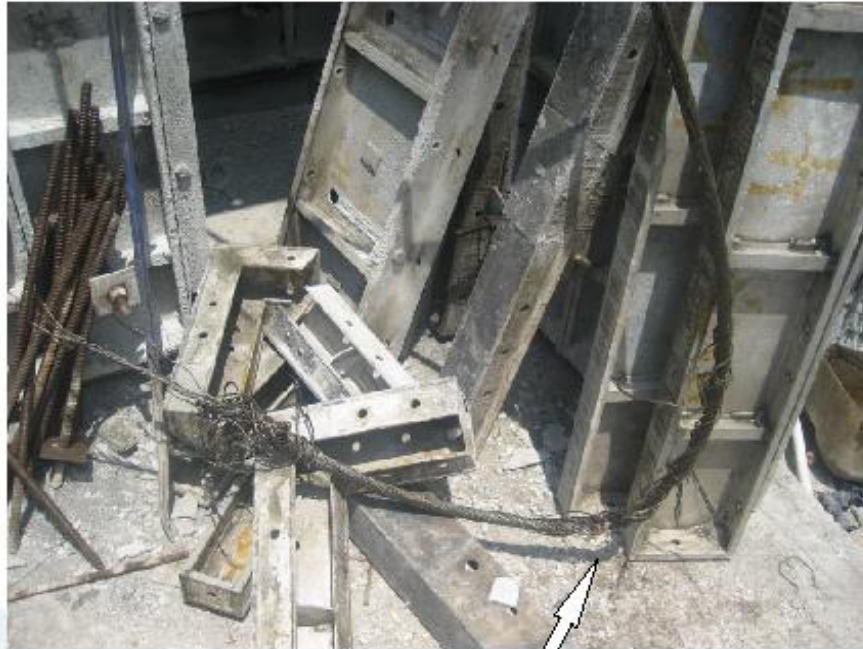
Hoisted Load (Concrete Skip) Fallen Down
