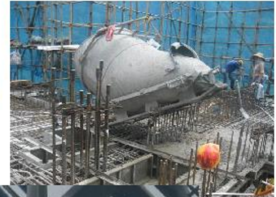
Hoisted Load (Concrete Skip) Fallen Down
