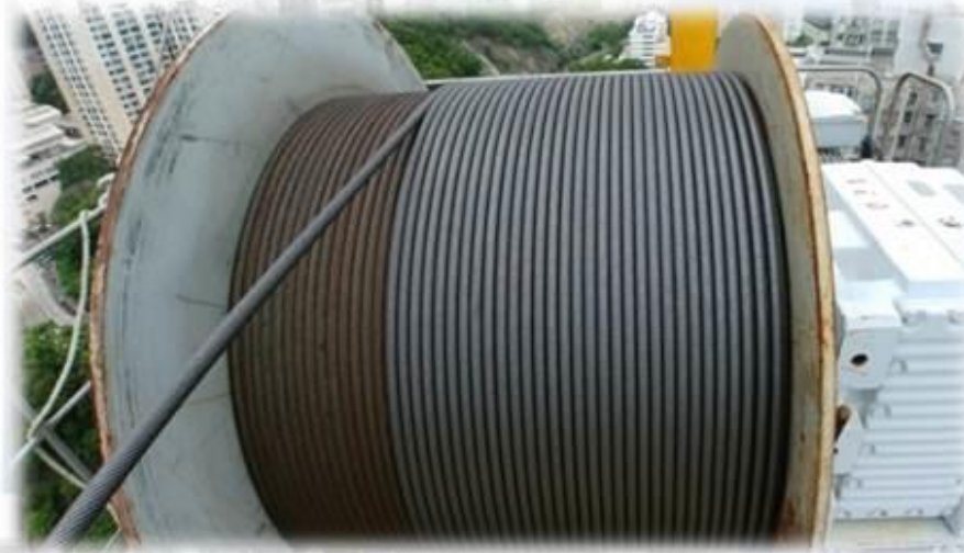
New Wire Ropes installation in the Tower Crane Hoisting
