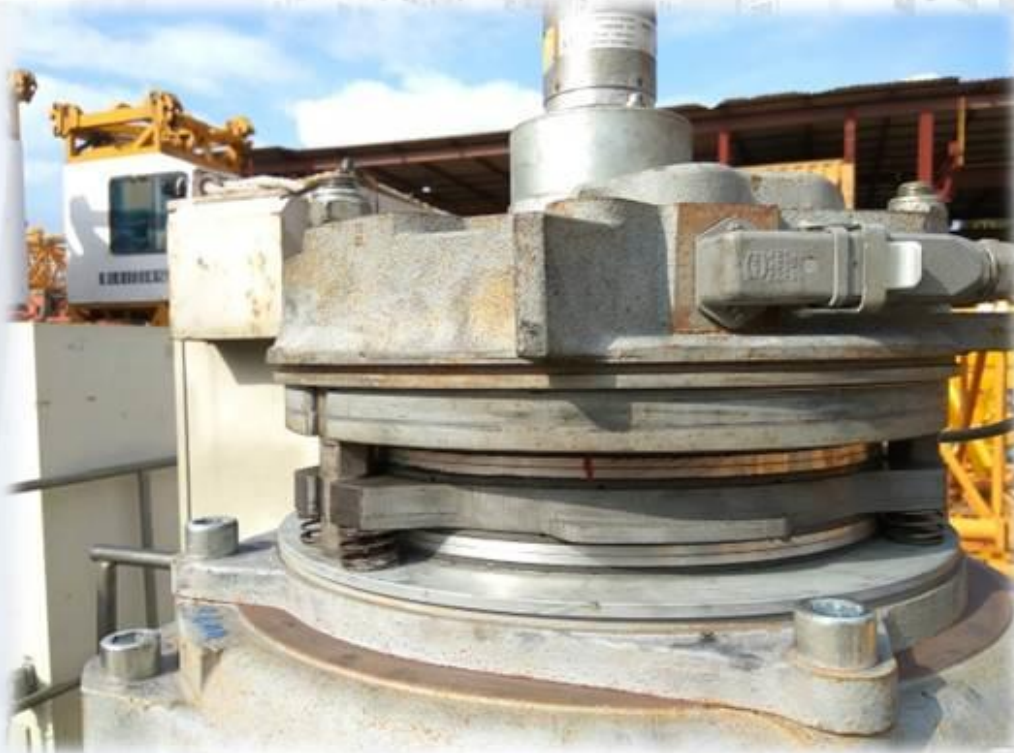
Checking the Tower Crane Motor and Brake
