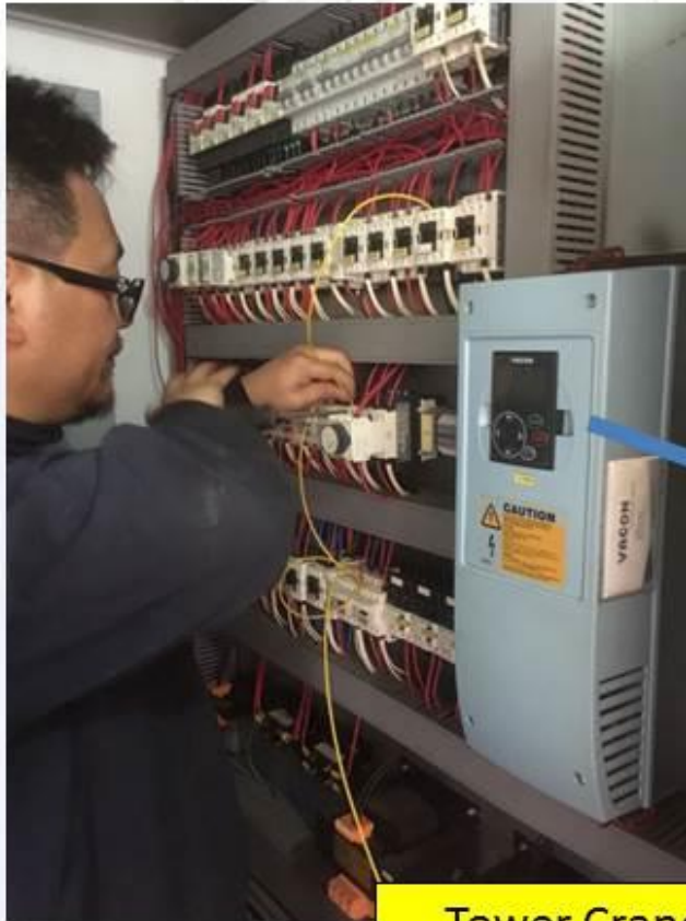
Tower Crane Inverter in Control Panel
