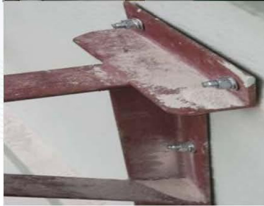
在狗臂架上安裝 3粒繫穩錨絲 3 anchor bolts are installed on metal bracket
