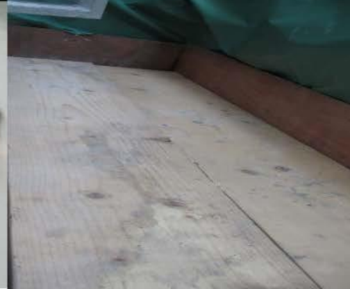
安裝踢腳板 及橋板 Installation of toe- board and planking board
