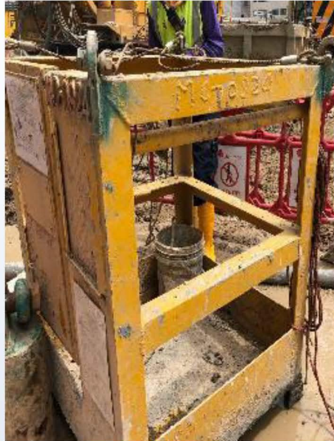
Man Cage Rigging Operation
