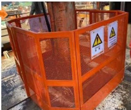
Improvement to Rigid RCD's Fences 改善鑽機鑽動圍欄
