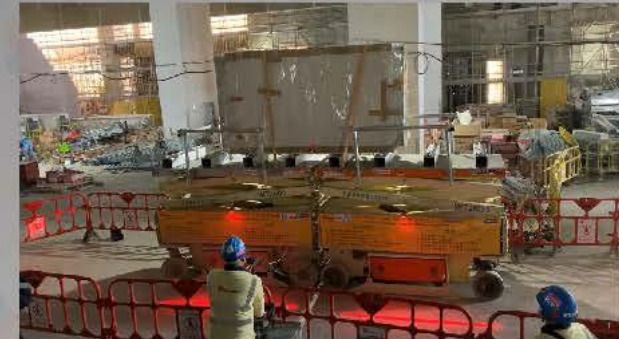
Synchronized Tailor Made Lifting Platform Capacity: 908kg
