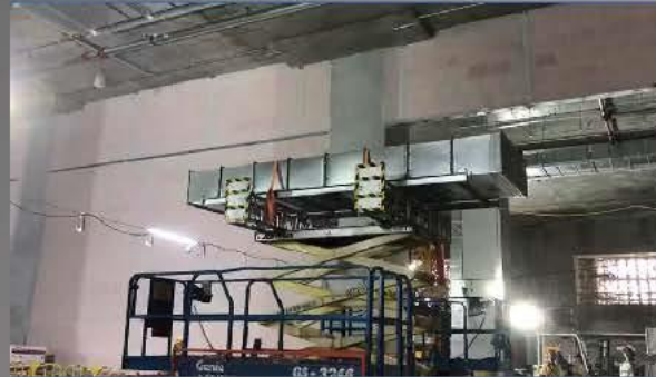
Tailor Made Lifting Platform Capacity: 454kg
