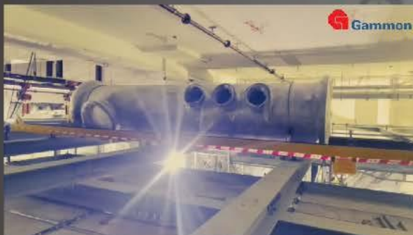
Pipe Header Module Delivery and Installation
