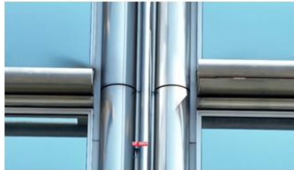
▲ Close Up Inspection
