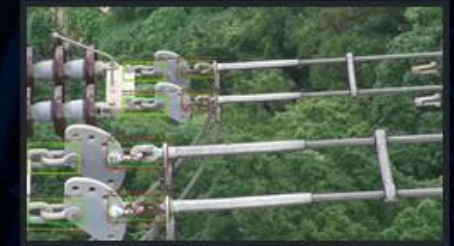
Pylon Tower / Radio Station Inspection
