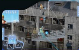
Use of Suspended Working Platform
