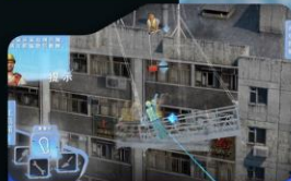
Use of Suspended Working Platform
