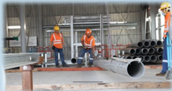
Assembly at Workshop
