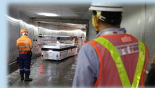
Horizontal Transportation by Lifting Robot
