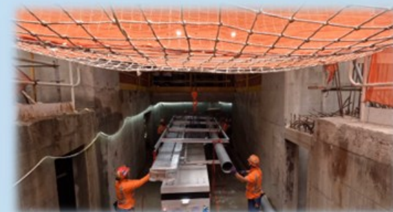
Tunnel to SG
