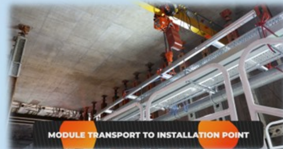
Hoisting beam at Tunnel
