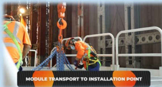
Rigging activity on proper platform
