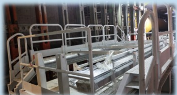
Maintain proper access / egress & guardrail for rigging activity
