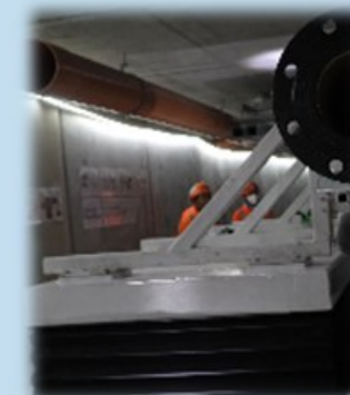
Modules installation at ceiling
