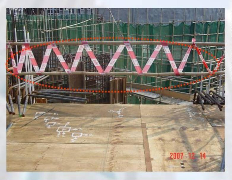
(PASS standard: Provide securely fixed timber / metal fencing with top railing (900mm-1150mm), middle railing (450mm to 600mm) & toeboard.)
