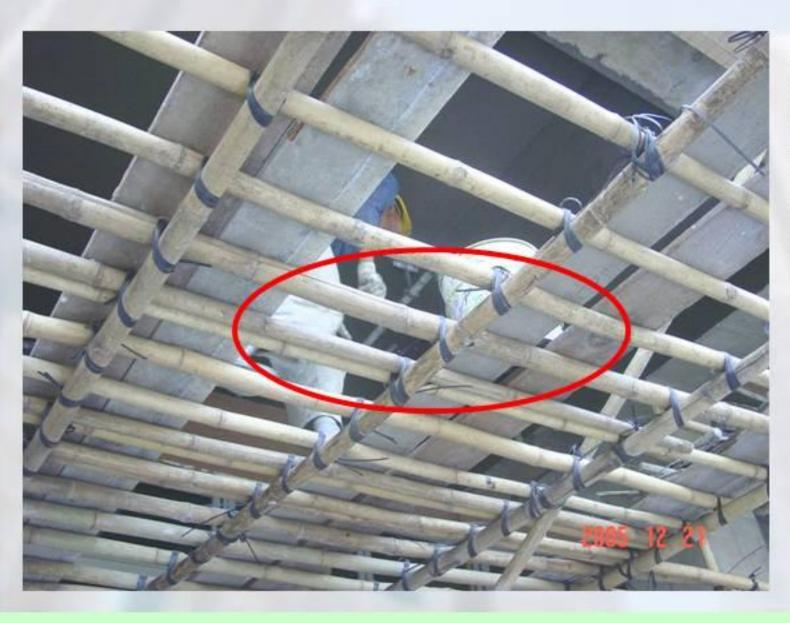
(PASS standard: To be closely boarded with a minimum of 3 supports and adequately restrained at both ends.)
