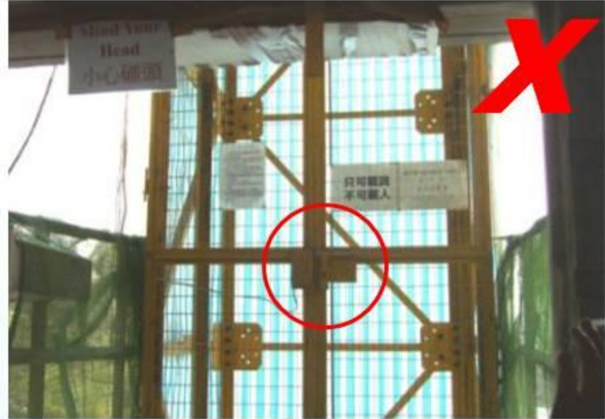
Unlocked material hoist gate when not in use
