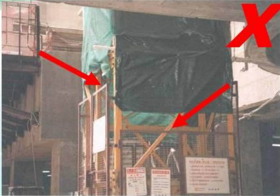
Material hoistway not fully covered
