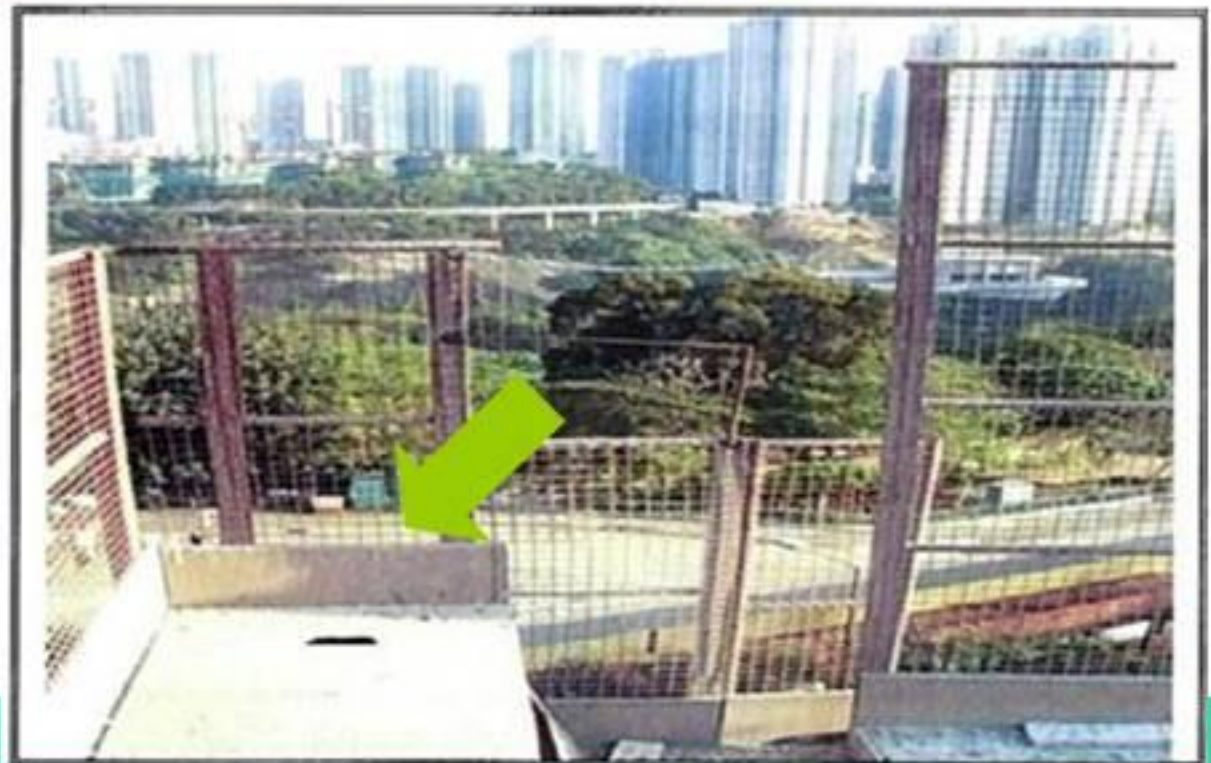
close boarding at floor opening
