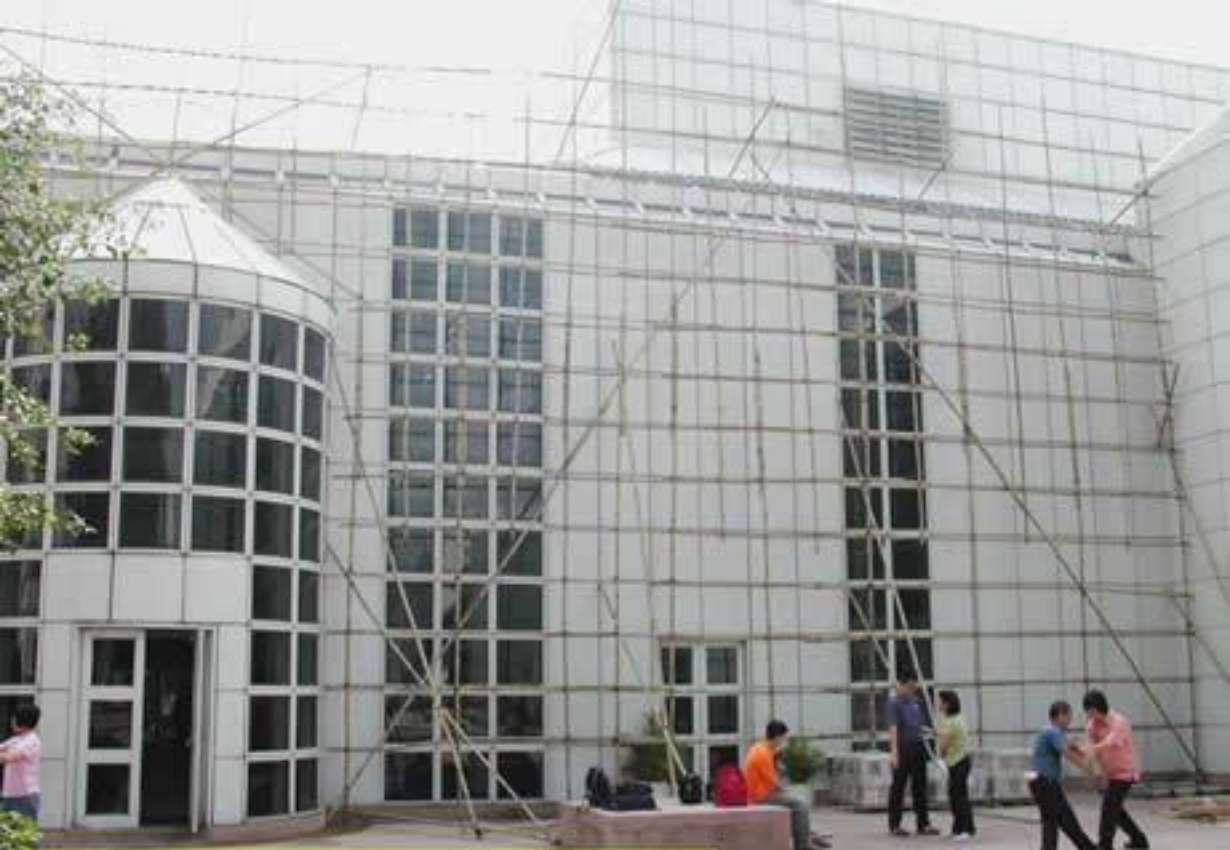
Single Layered Bamboo Scaffolds
