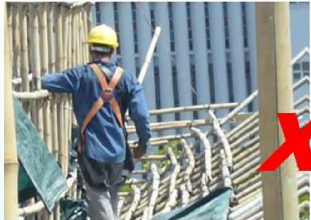
Safety harness not properly attached to fall arresting system – independent lifeline
