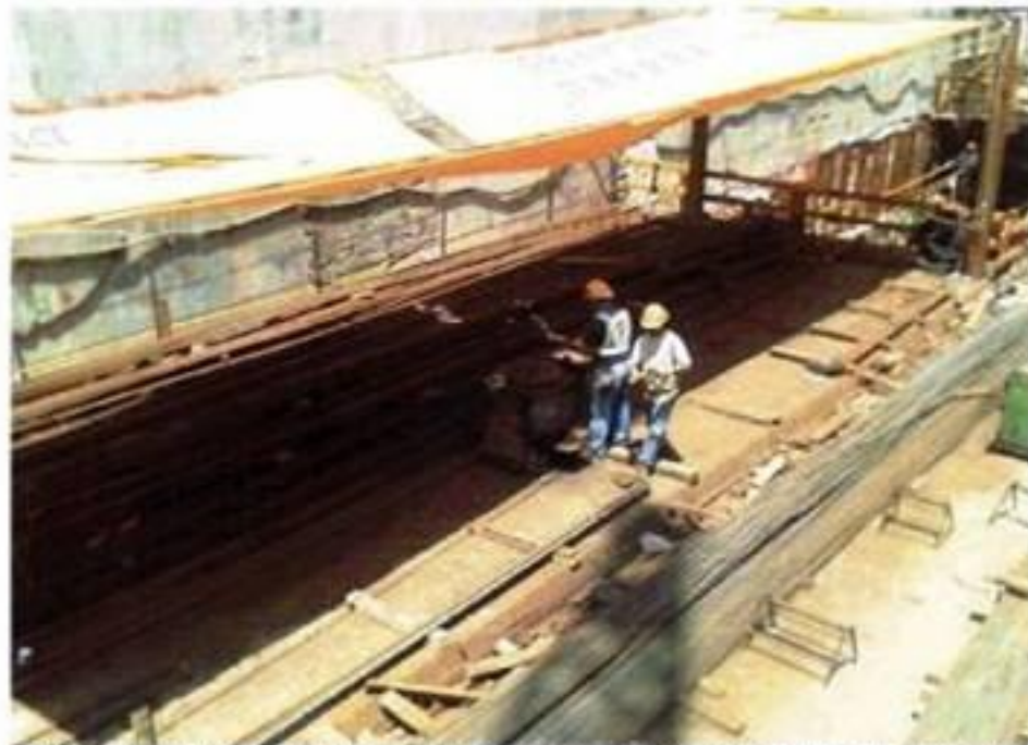
Heavy Duty Tarpaulin sheets are extended during rebar bending works to provide shelter for steel fixer in sunny and rainy weather.
