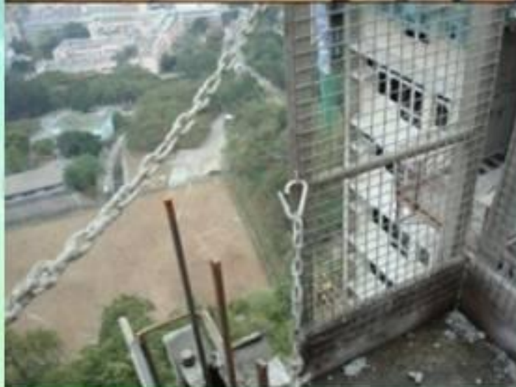
Defective fencing of working platform
