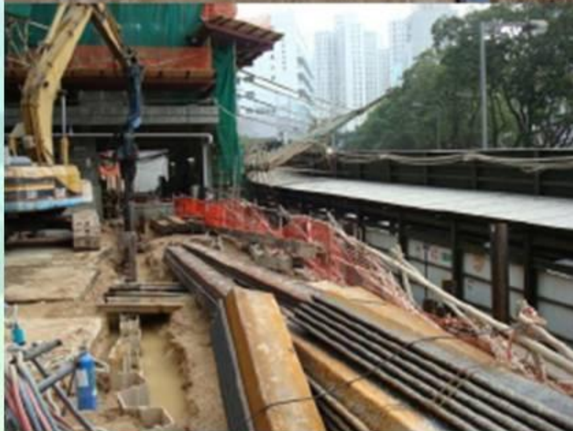
Storage of sheet piles on edge of slope
