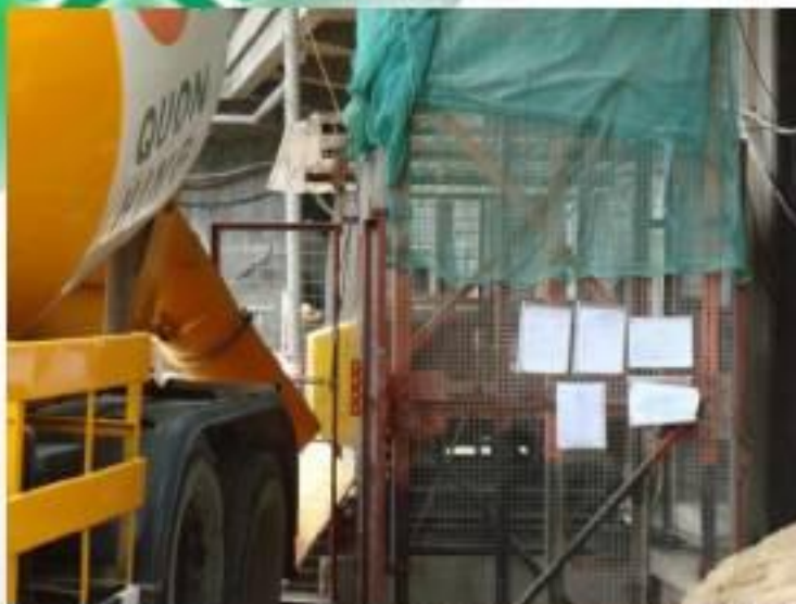
Defective interlocking gate
