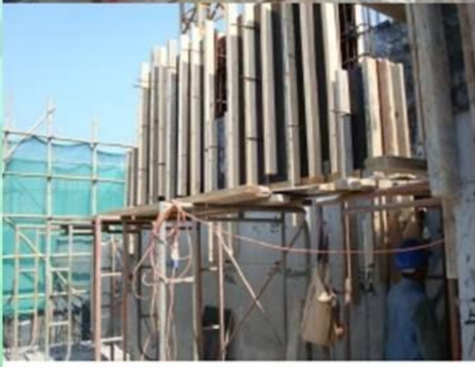
Unsafe working platform
