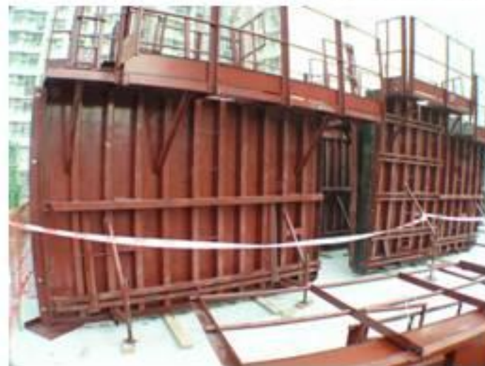
Metal Formwork
