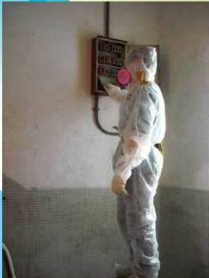
Asbestos Removal Works for Fuse Box
