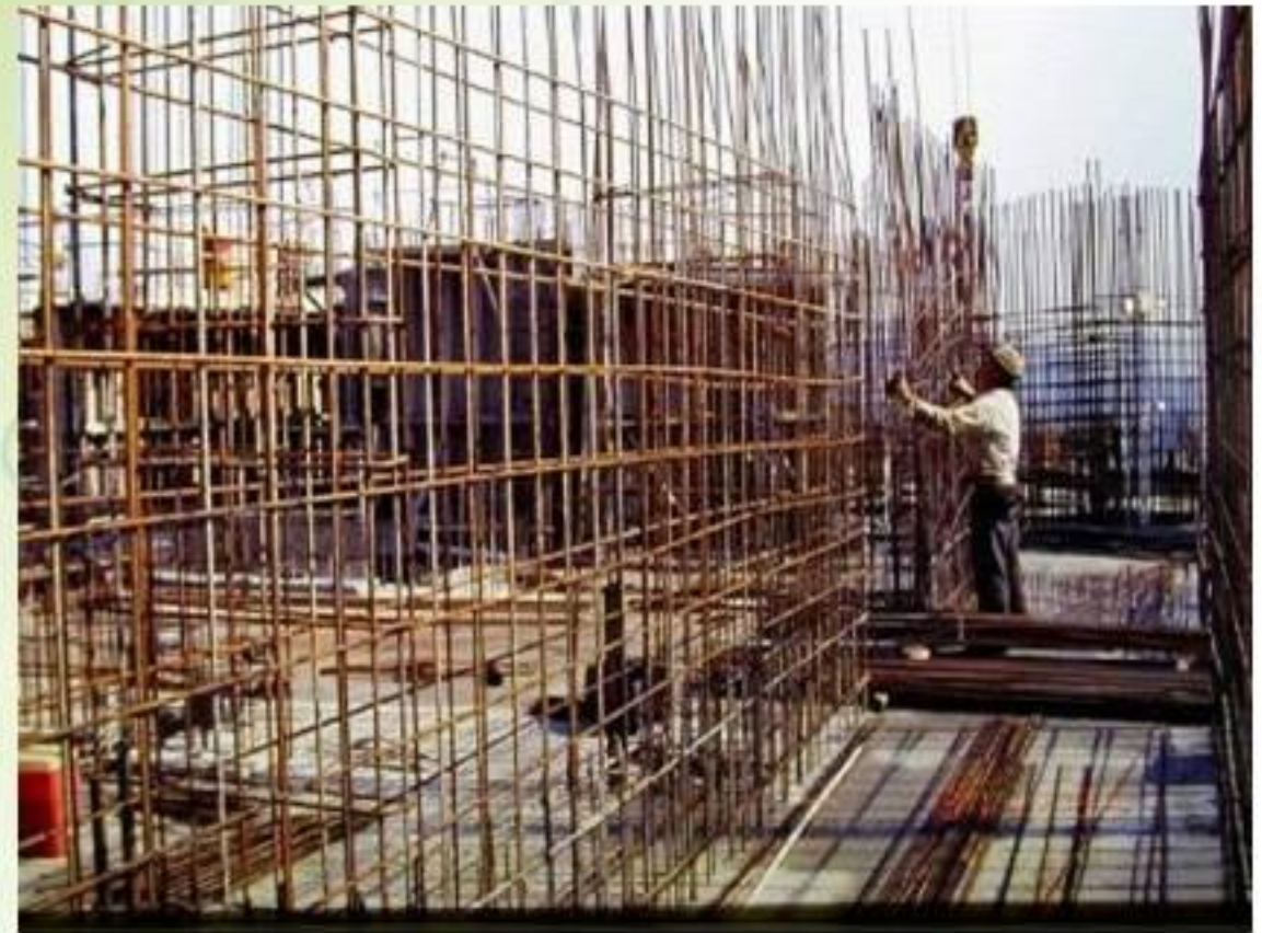
Fixing of Fabric Reinforcement
