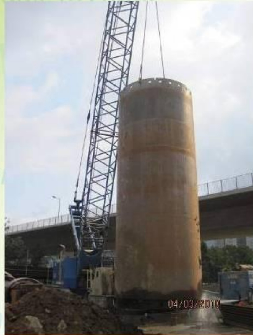
Lifting Steel Casing (Vertical)
