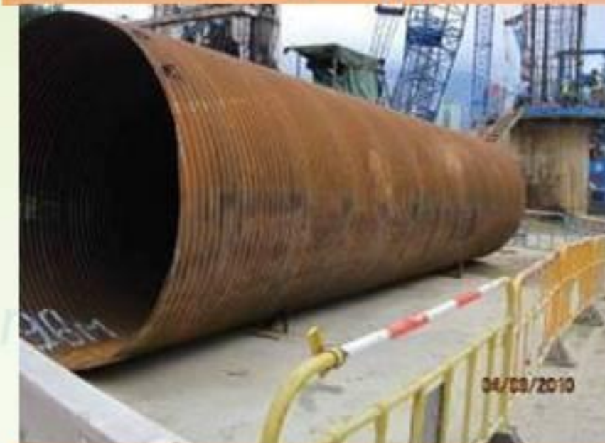
Proper Storage of Steel Liner
