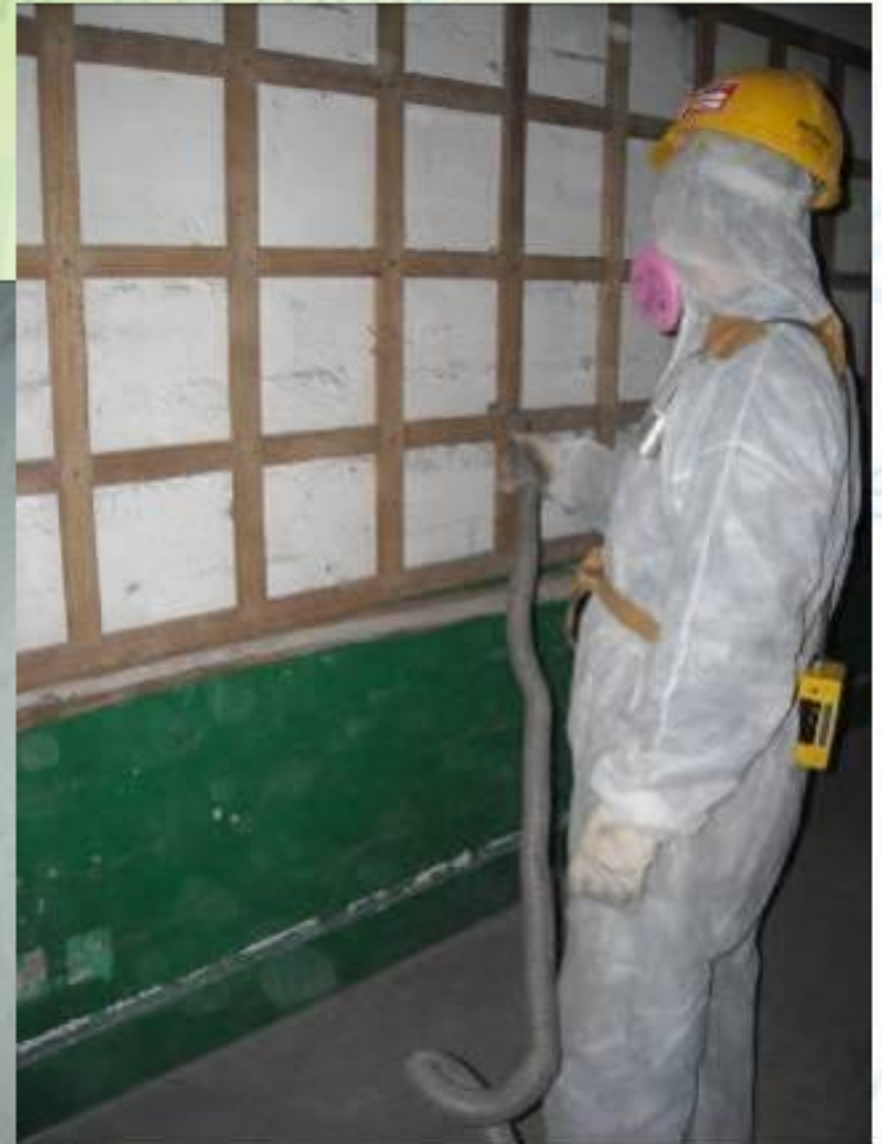
Asbestos Particles Removing
