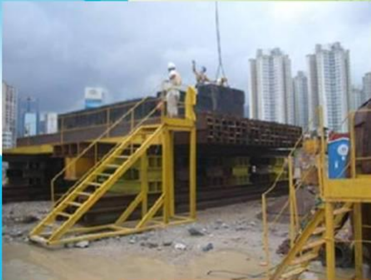
Final Set up of Mass Steel Kentledge
