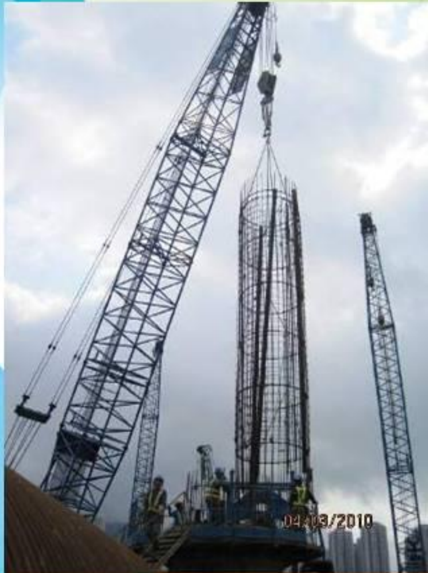
Lifting Steel Cage (Vertical)
