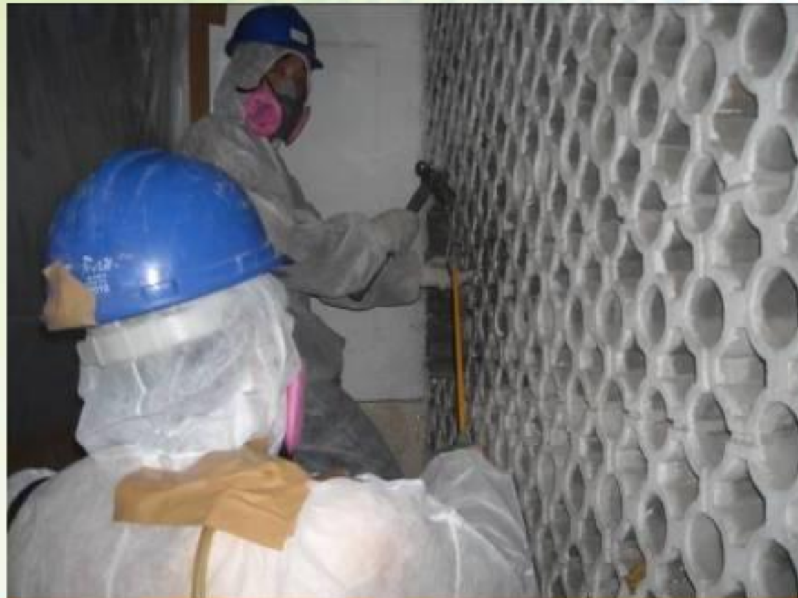
Asbestos Removal Works for Grille Panel
