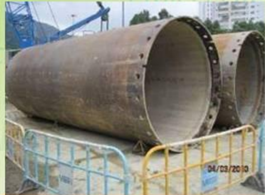
Proper Storage of Steel Casing
