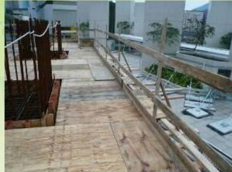
Working Platform Provided for Steel Fixing Works at Heights (above 2m)
