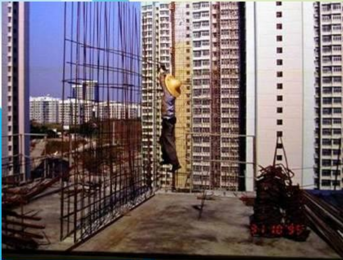
Traditional Rebar Fixing
