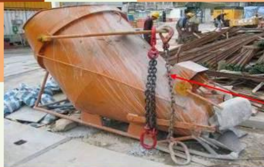
New Design Double Chain Sling for Lifting of Hopper
