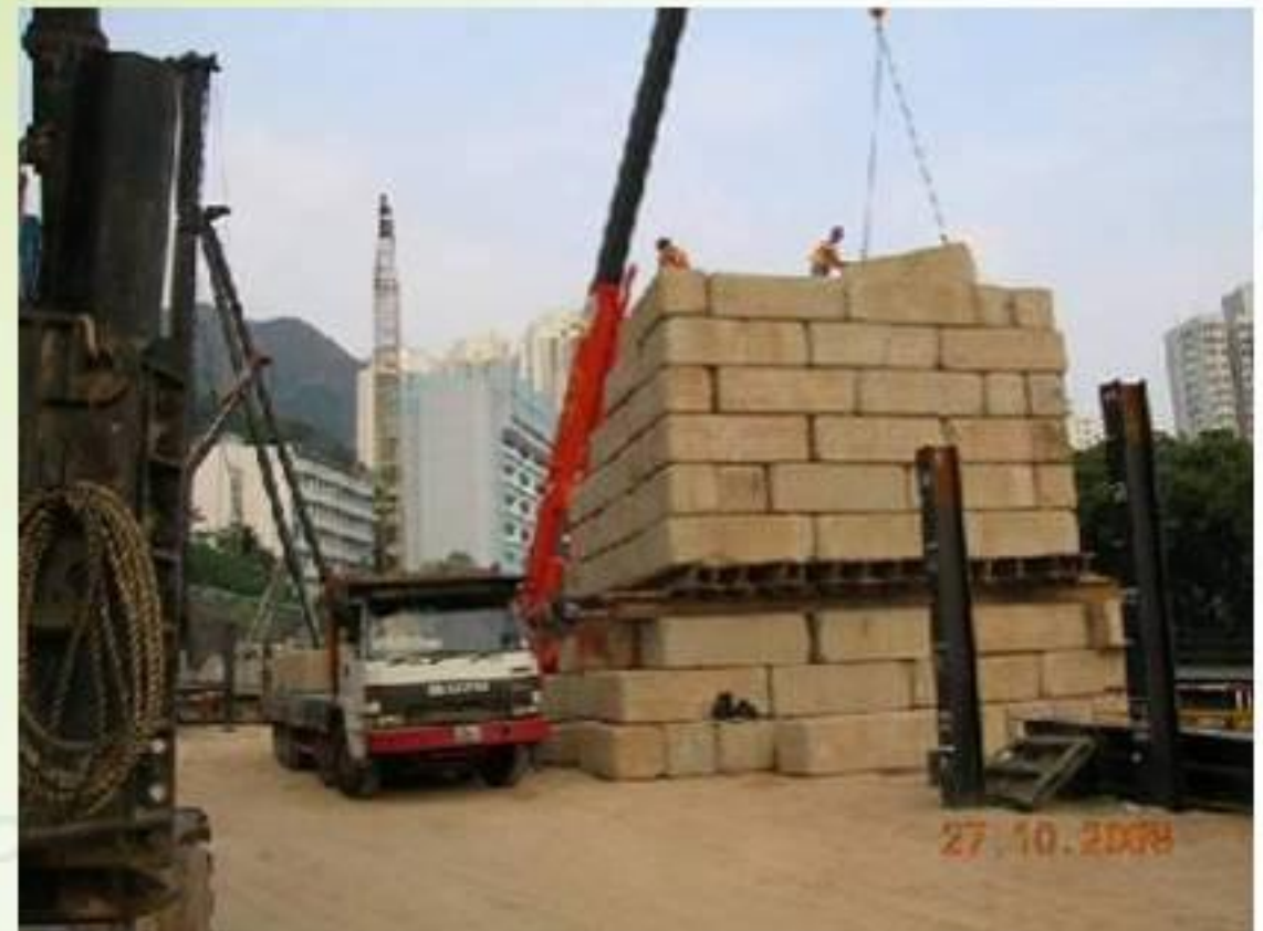
Typical Conc. Block Kentledge
