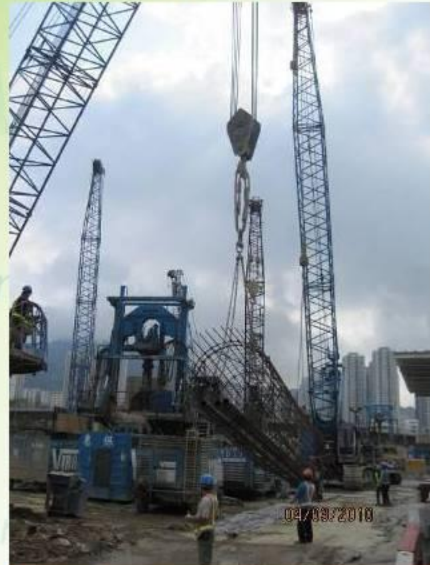
Lifting Steel Cage by 2 Cranes (Horizontal)
