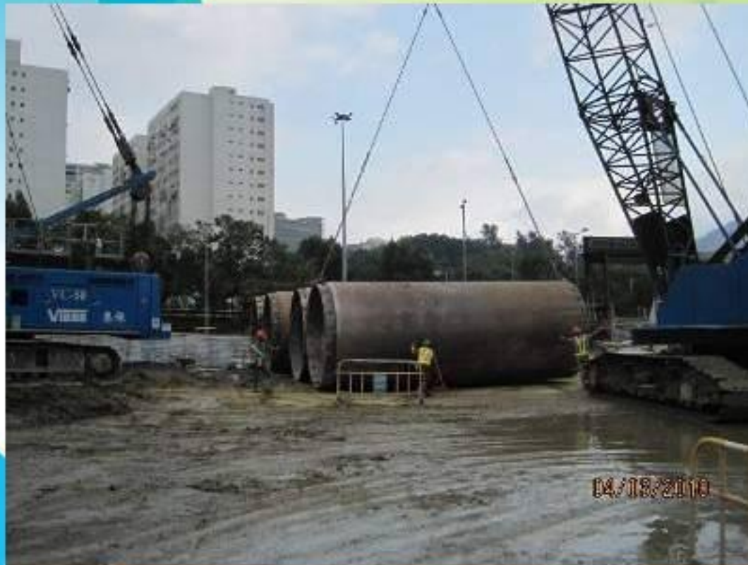
Lifting Casing (Horizontal)
