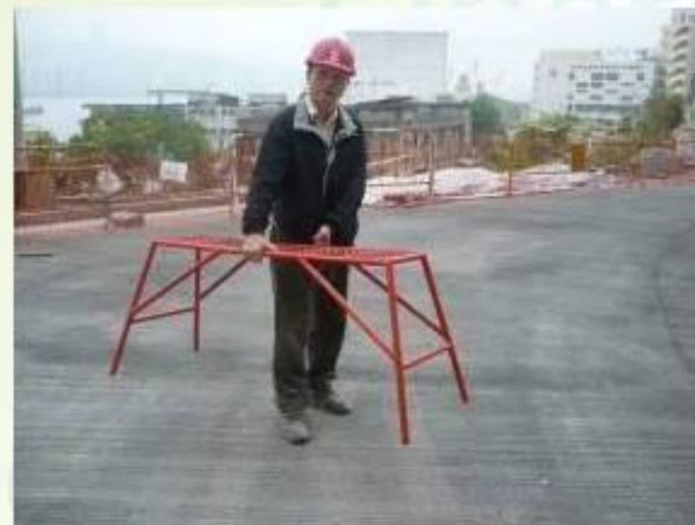
Working Platform Provided for Steel Fixing Works at Heights (above 2m)
