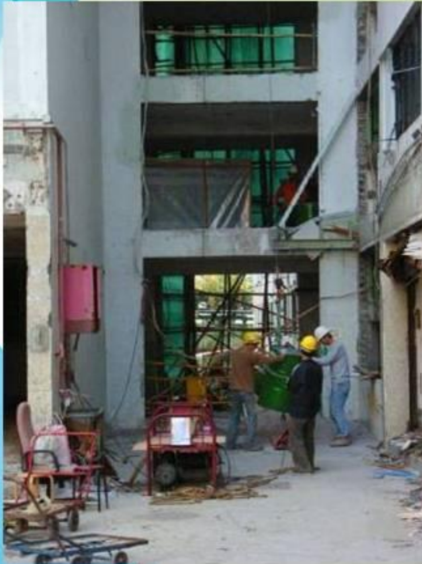
Transferring Sealed Drum to the Ground
