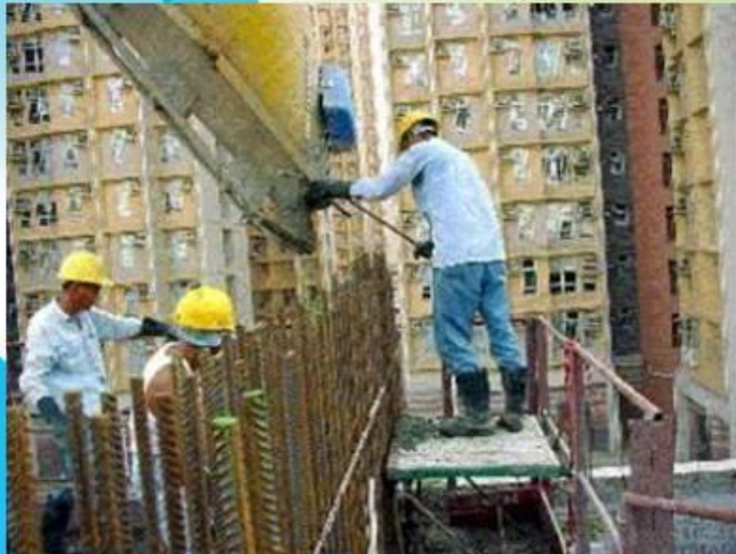
Temporary Working Platform Provided for Concrete Pouring at Heights (below 2m)
