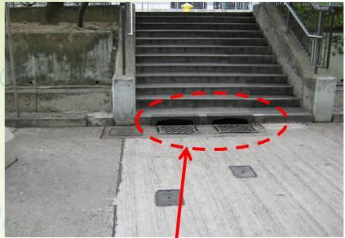
Gullies in front of stairway
