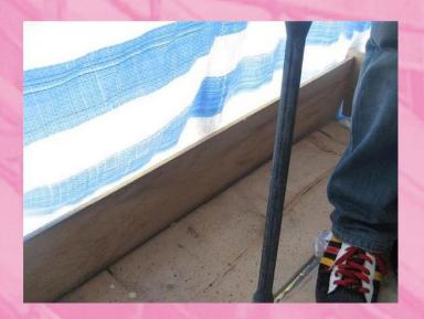
Toeboard, Closed Planking & Tarpaulin Sheet Envelope of Truss-out Scaffold
