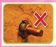
Diagram 4: Extra space at drill hole was stuffed with nylon strip, which was no use for the anchor to hold the base material effectively.
