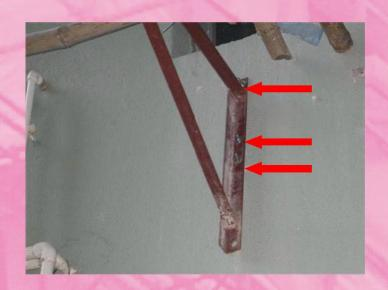
Three Anchor Bolt for Steel Bracket
