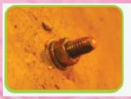
Diagram 3: An expansion anchor bolt installed at the base material matched the drill hole.
