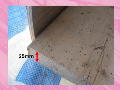
Thickness of Planking = 25mm for Planking of 200mm wide
