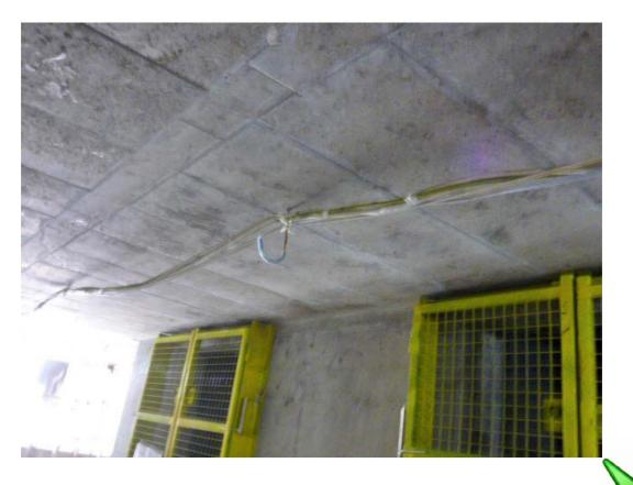
**Electric Cables were Adequately Suspended**
