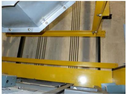
Guard-rails and toe-boards were installed on the car top.
