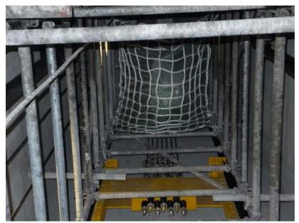
Metal scaffolding was provided inside the lift shaft together with safety nets.
