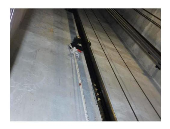
Independent life lines were installed to the steel bracket above the car top.
