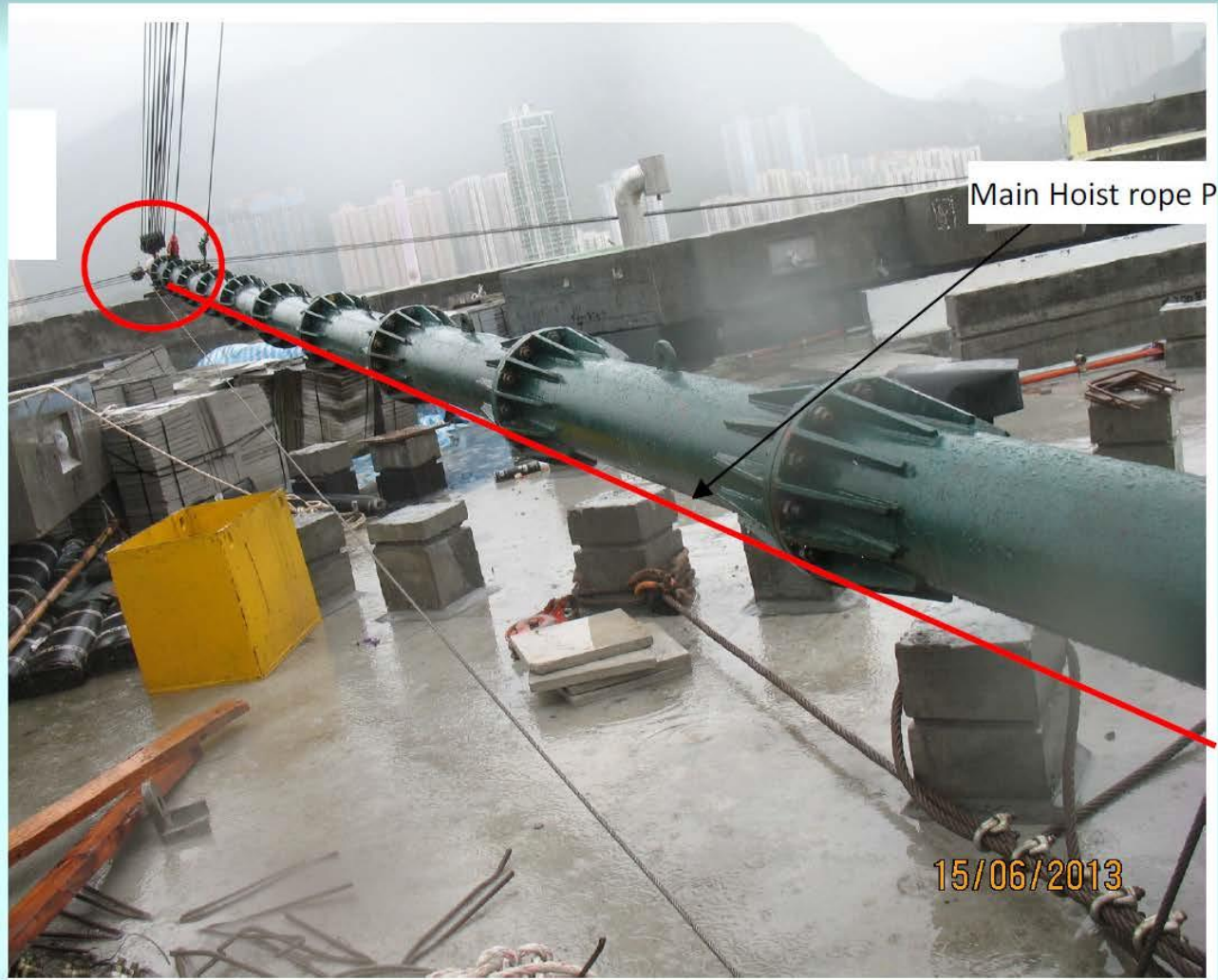
Boom rested on parapet and pull by 2 side wires
