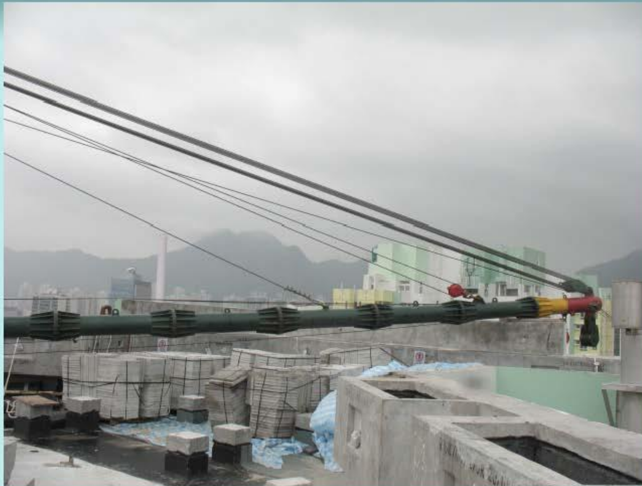
Boom rested on Parapet
