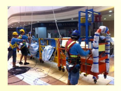
Failure of single climber and safety lock lead to excessive tilting of SWP, also makes rescue difficult in case of emergency
