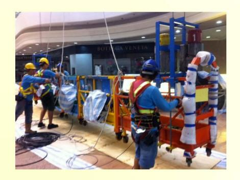
Single climber & safety lock make it difficult to rescue in inaccessible or isolated locations i.e. end walls
