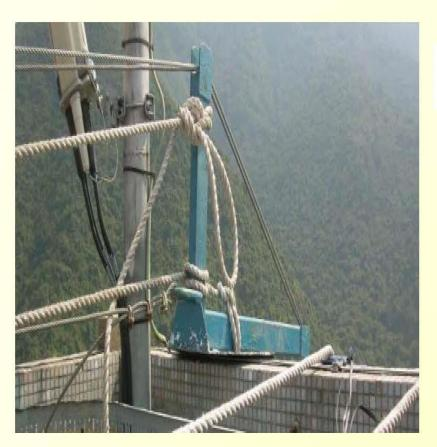
the Code of Practice of Labour Department provides guideline for practitioners. It does not mean that the practitioner must install outriggers as illustrated by the Code. The practitioners must, however, ensure that the outriggers was firmly anchored.
