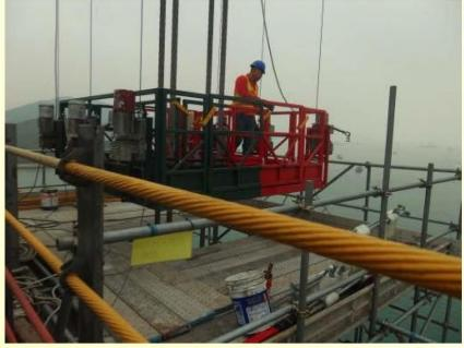
Single climber & safety lock system make it difficult to rescue in confined spaces in case of climber and/or safety lock failure
