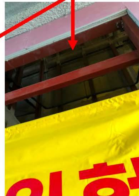
Lift Shaft Opening Fenced with Safety Net
