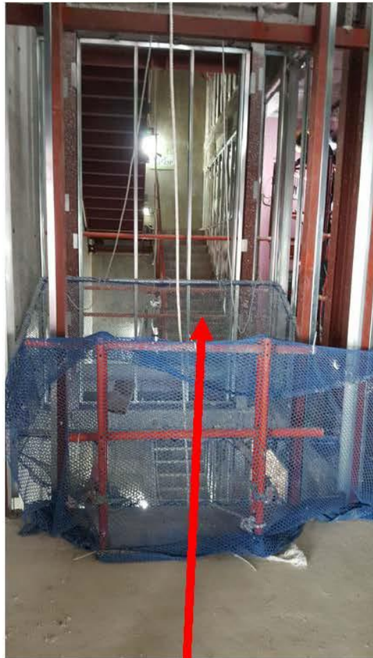
Safety Net at Opening
