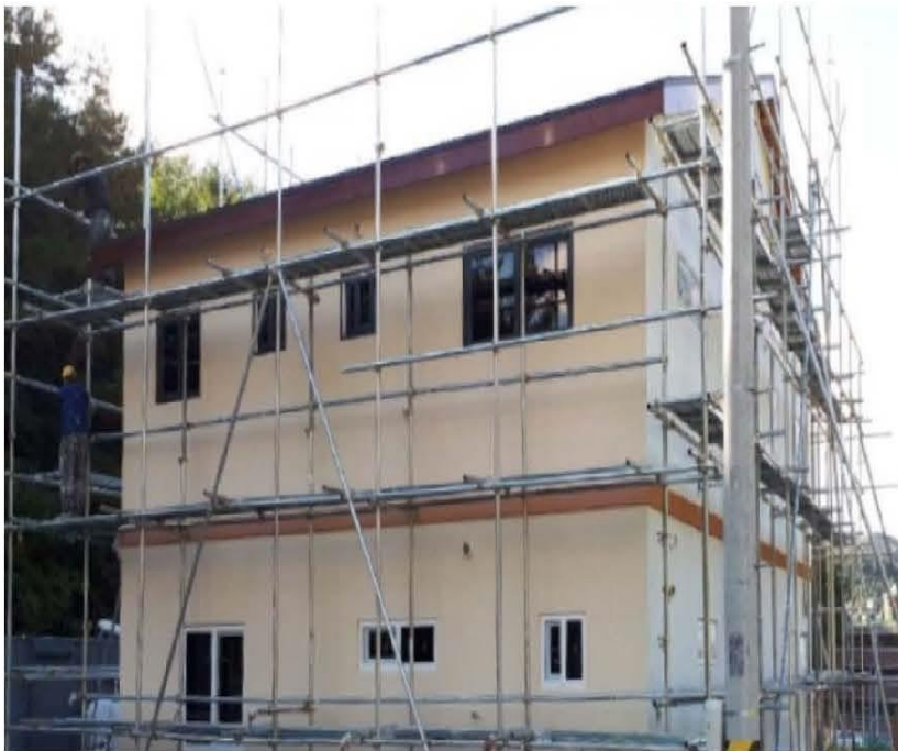
[Steel pipe scaffolds]
