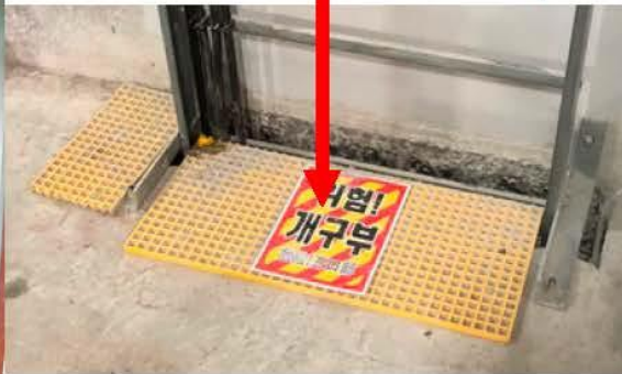
Fibre Board at Floor Opening
