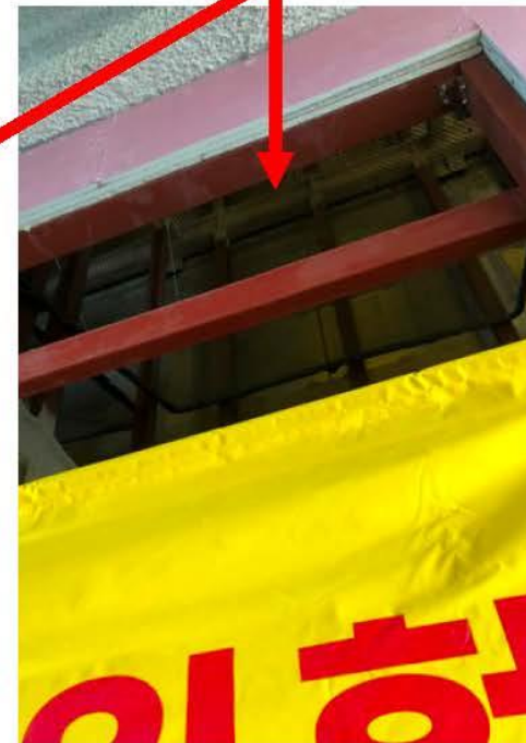
Lift Shaft Opening Fenced with Safety Net
