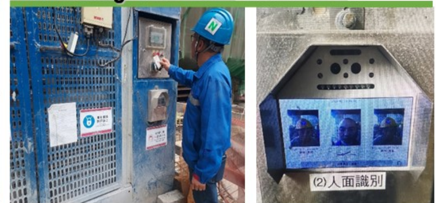
Face recognition for material hoist
