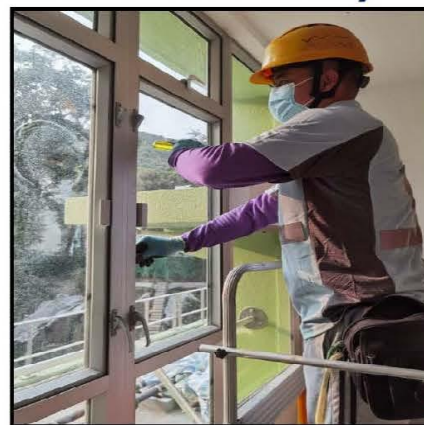
Installing the glazing beads
