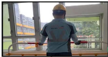
Barricading working area
