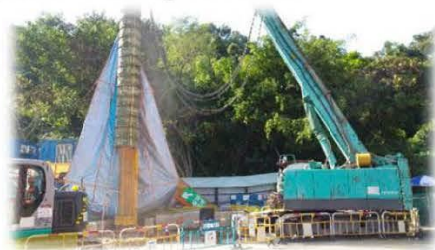
Boring machine for socketed H pile, mini pile, pipe pile etc.
