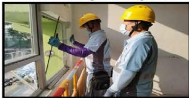
Barricading working area
