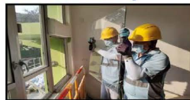
Shifting the panel to the position
