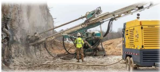
Drill machine for soil nail
