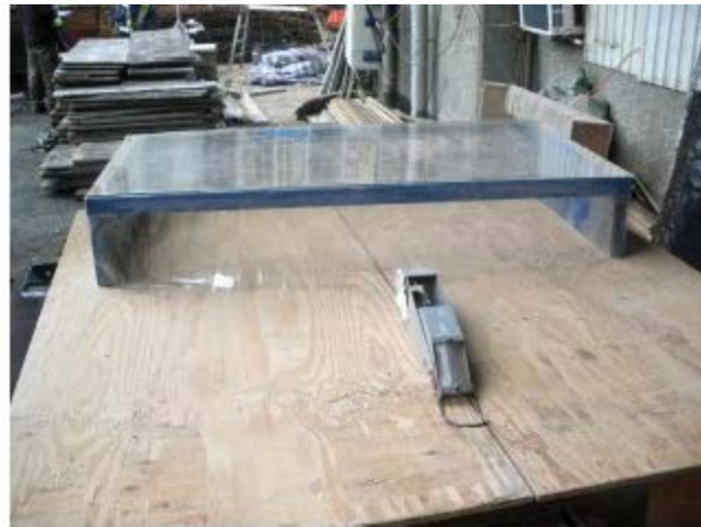
PH 01 : The cover putting onto the bench saw
