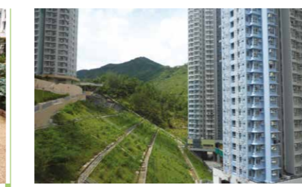
▲ 水泉澳邨斜坡綠化 Green treatment to slopes at Shui Chuen O Estate
